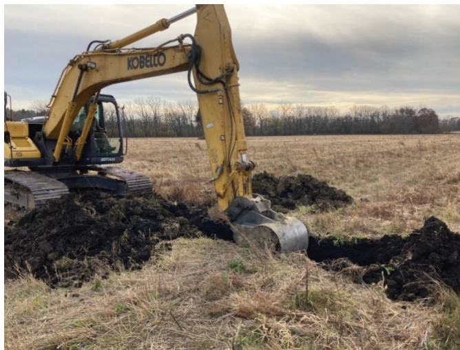
An excavator disabling drainage tile at the Meachem Road ILF site in Racine County.
