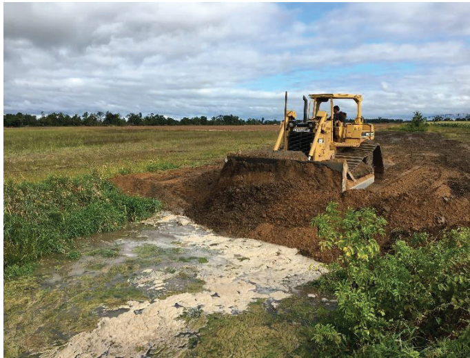
The filling of drainage ditches to restore wetland hydrology at the Plover Soik ILF project.
