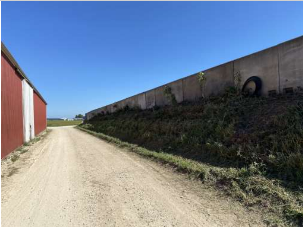
Photo #: IMG_3667 Date/Time: 9/4/2024 10:57 AM Photo taken by: J. Borgrud Photo Location Williams Bedrock Bovines – Main Farm Description: Looking north towards the VTA from between the feed storage area and the machine sheds
