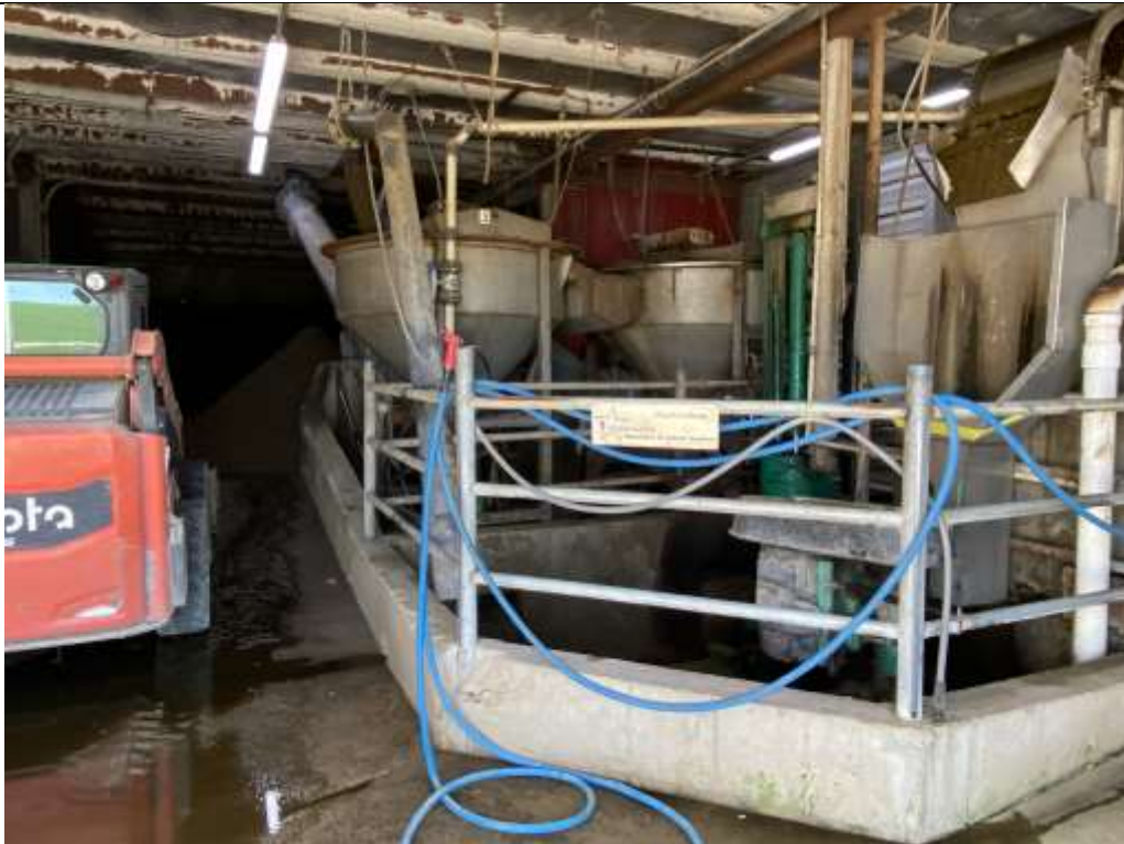
Photo #: IMG_3655 Date/Time: 9/4/2024 10:43 AM Photo taken by: J. Borgrud Photo Location Williams Bedrock Bovines – Main Farm Description: Looking into the sand separation building located between the freestall barns
