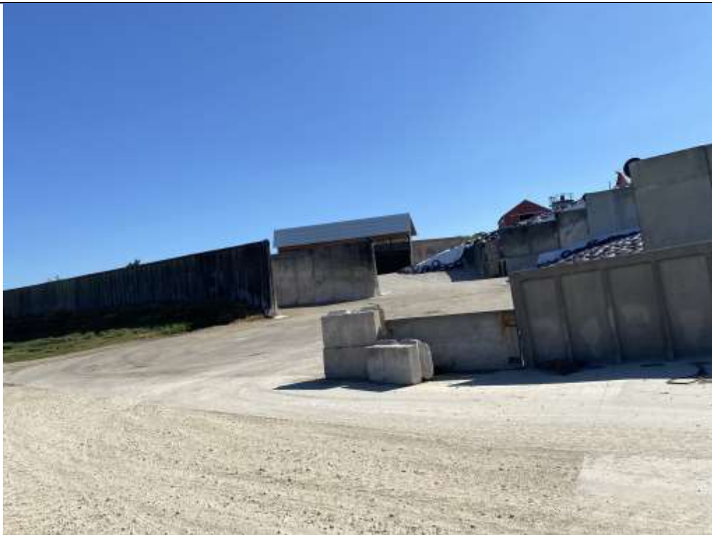
Photo #: IMG_3670 Date/Time: 9/4/2024 10:58 AM Photo taken by: J. Borgrud Photo Location Williams Bedrock Bovines – Main Farm Description: Looking east at the feed storage area from the south east corner of the VTA
