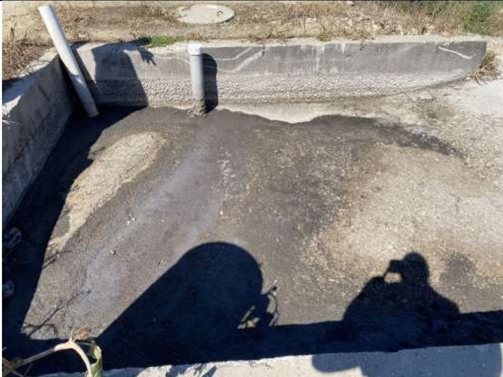
Photo #: IMG_3671 Date/Time: 9/4/2024 10:58 AM Photo taken by: J. Borgrud Photo Location Williams Bedrock Bovines – Main Farm Description: Concrete sediment basin for feed storage area
