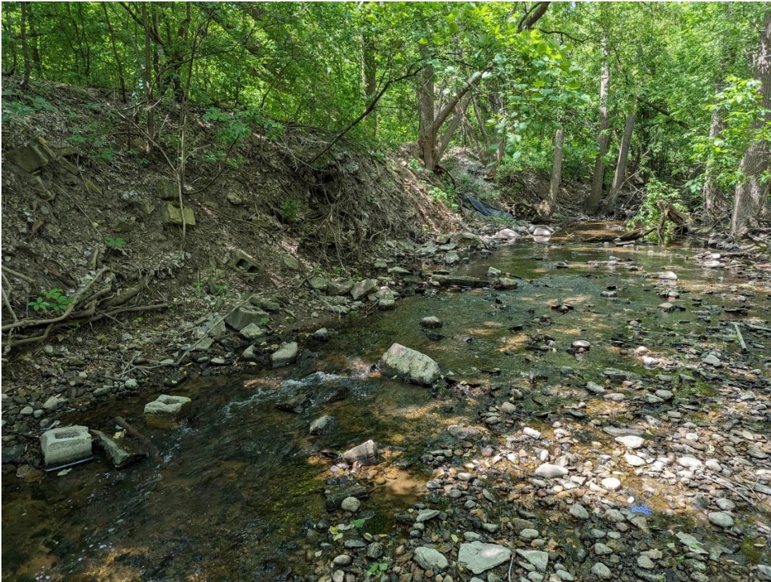
Image 2.3 – Bank with exposed roots.
