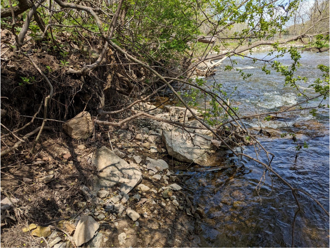
Image 1.4 – Bank, undercut, with fallen trees.
