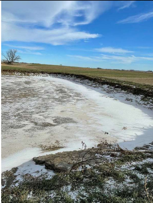
Photo taken by: E. Struck Photo date: 12/05/2024 Description: Photo 13. WSF1 southern end. Note ramp in foreground and earthen bottom and side walls. Photo facing SE.
