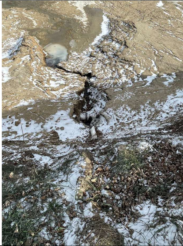
Photo taken by: E. Struck Photo date: 12/05/2024 Description: Photo 16. WSF1 earthen sidewall erosion. Photo facing E.
