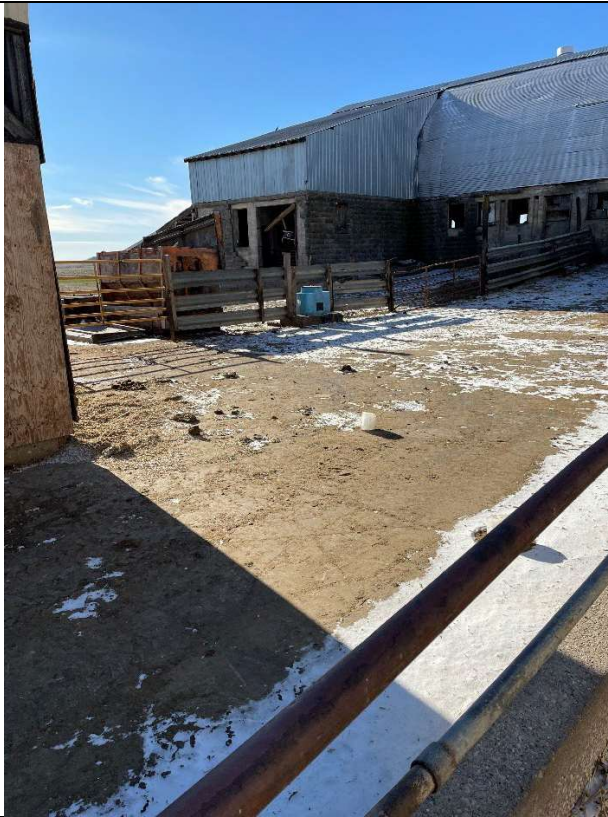
Photo taken by: E. Struck Photo date: 12/05/2024 Description: Photo 3. Outdoor lot without runoff controls. Photo facing SE.
