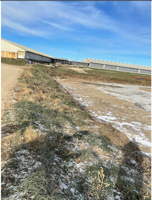
Photo taken by: E. Struck Photo date: 12/05/2024 Description: Photo 12. WSF1 west sidewall. Note frozen solids and earthen bottom and side walls.. Photo facing N.
