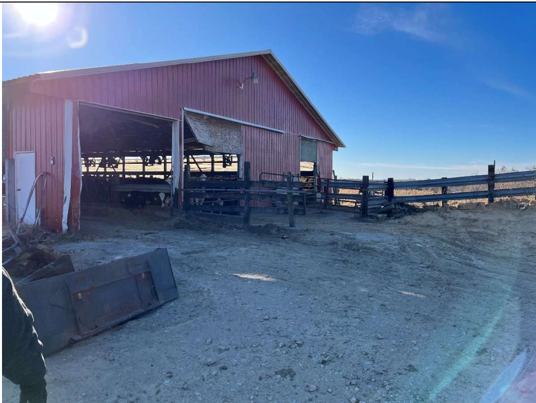
Photo taken by: S. Wettach Photo date: 12/05/2024 Description: Photo 6. North end of Marks Avenue freestall barn. Photo facing SW.
