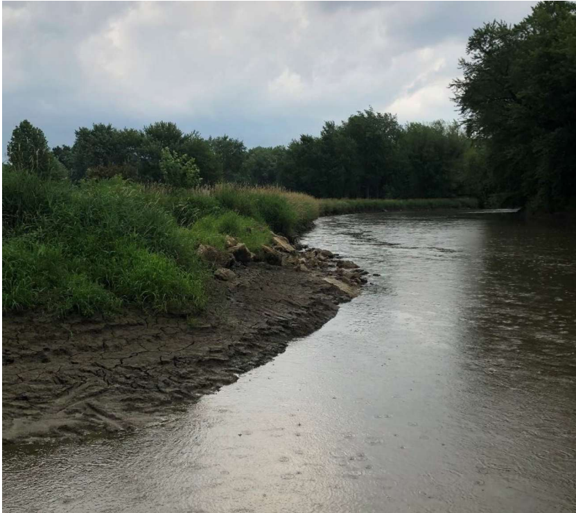
Image 6 – Vegetative overhang and predominately bare banks
