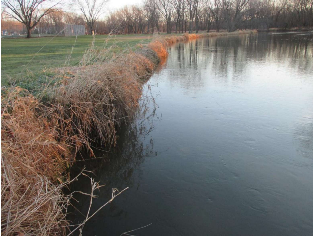
Image 3 – Severe vegetative overhang
