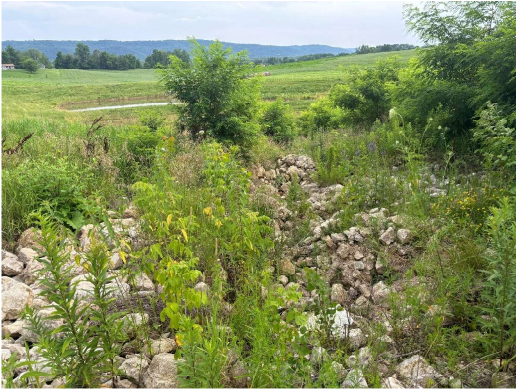
Image 2.3 – South-facing view from pre-pre-sedimentation riprap area with vegetative development and flow path.
