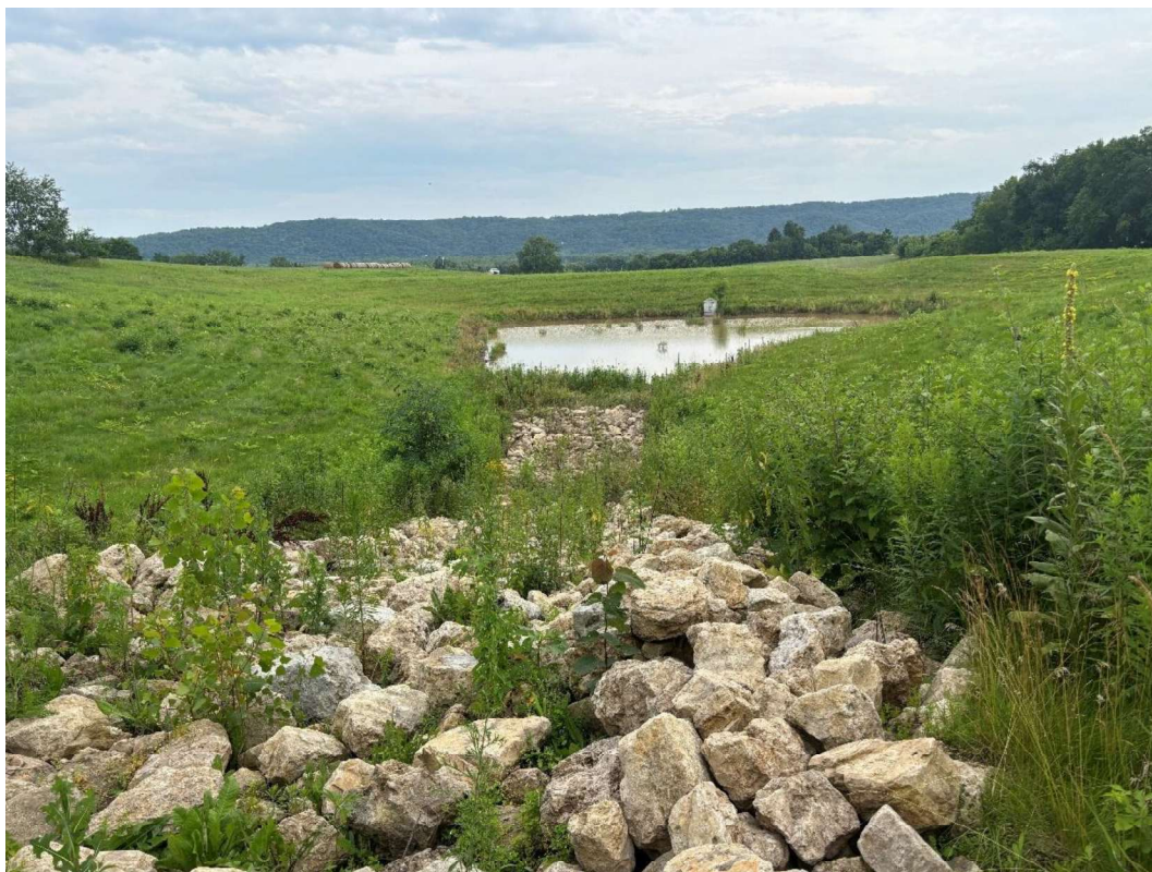
Image 1.5 – Riprap flow path from pre-sedimentation basin into Pond #1.
