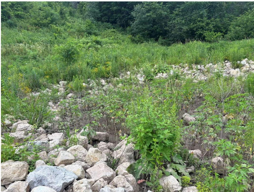
Image 1.4 – Pre-sedimentation basin into Pond #1.
