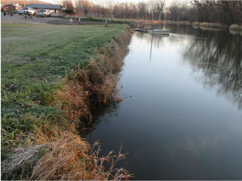
Image 1 – Severe vegetative overhang and extremely steep banks. As demonstrated by the dock walkway, the river is much higher than average which conceals most of the exposed banks and erosion
