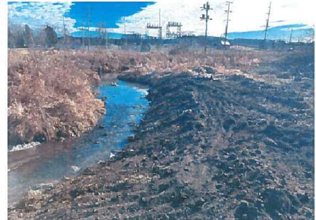
Site 2 rip rap covered with soil.
