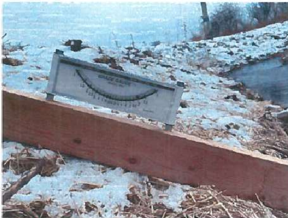
Site 4 at a 2:1 slope with adequate mulch.
