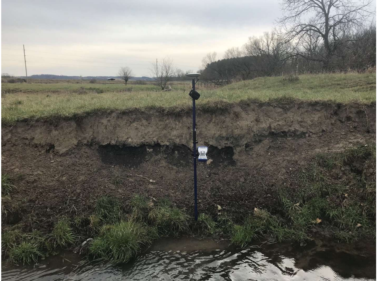
Looking at center proposed riprap near pond.
