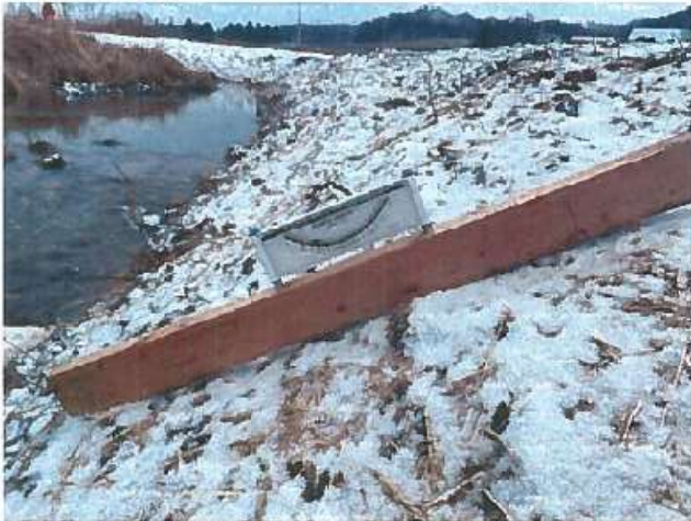
Site 1 at roughly 2:1 slope with adequate mulch.
