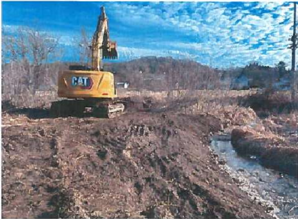
Site 3 rip rap covered with soil.
