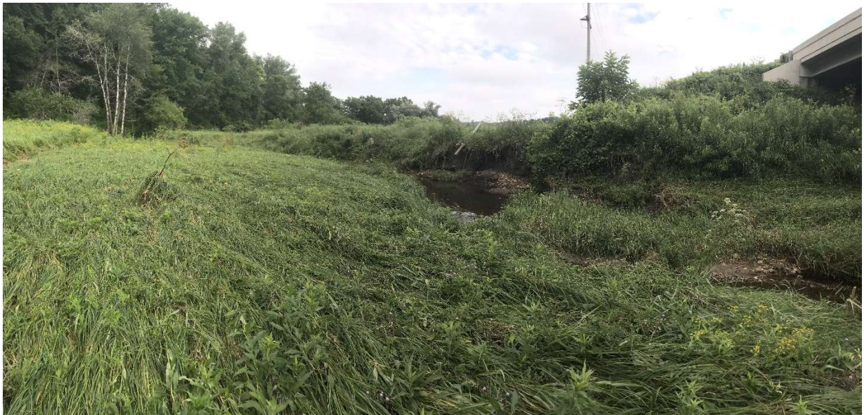
Looking upstream near HWY 23 bridge.
