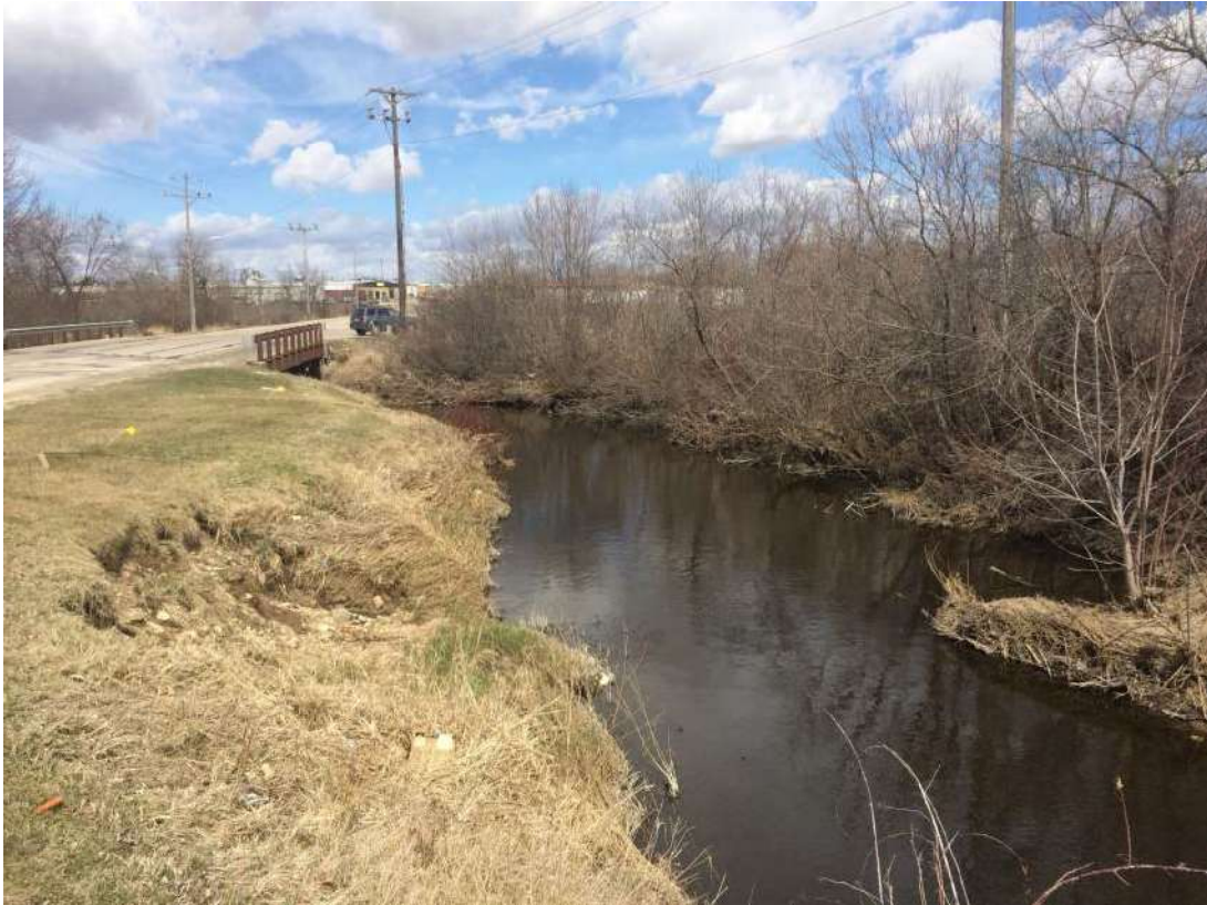
Figure 13. SB4/NB4 Streambank Image 1
