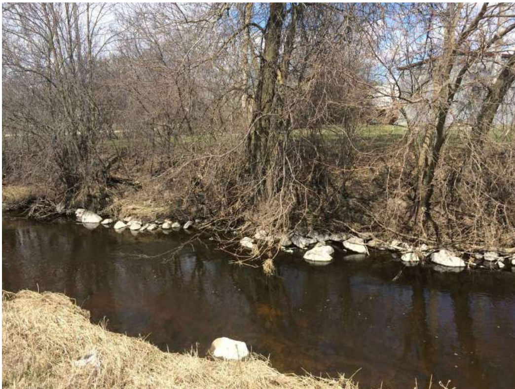
Figure 5. SB1/NB1 Streambank Image 2
