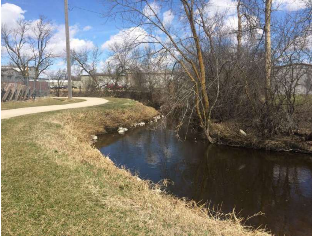
Figure 4. SB1/NB1 Streambank Image 1
