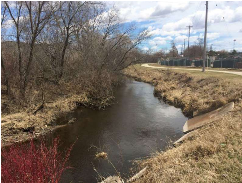
Figure 12. SB3/NB3 Streambank Image 3
