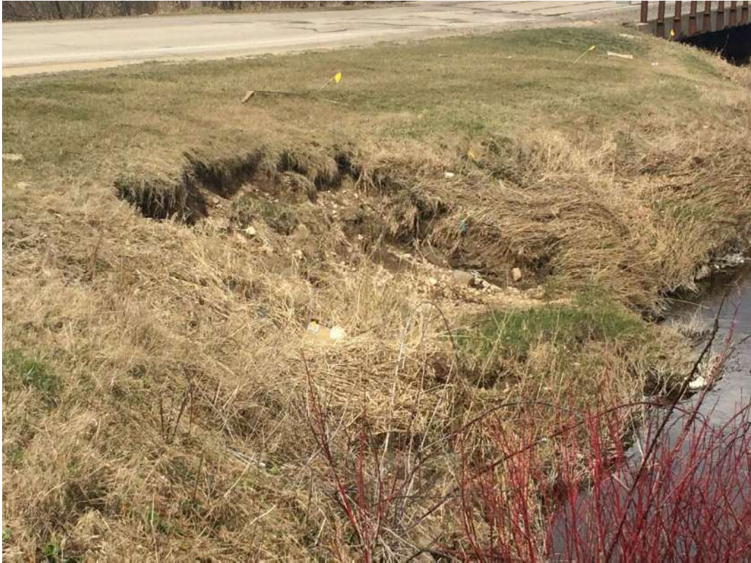
Figure 15. SB4/NB4 Streambank Image 3
