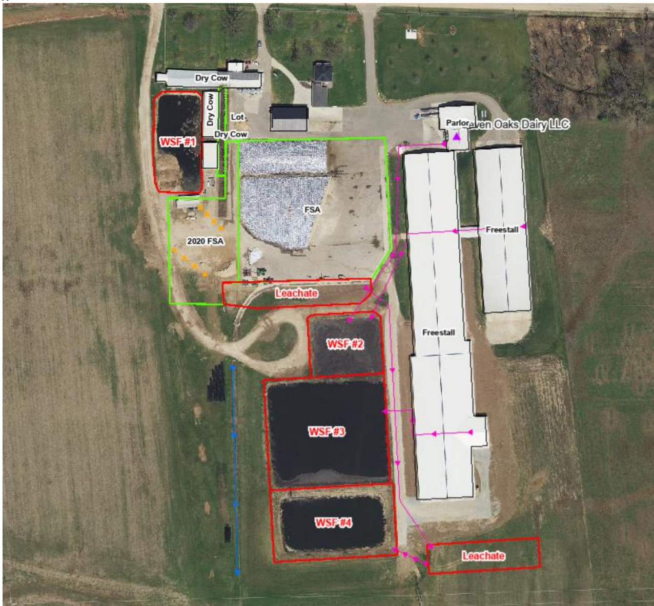
Figure 1. Aerial overview of Seven Oaks Dairy main site. Pink arrows indicate manure transfer lines. Yellow arrows indicate contaminated runoff and leachate flow paths. Blue arrows indicate approximate stormwater flow.
