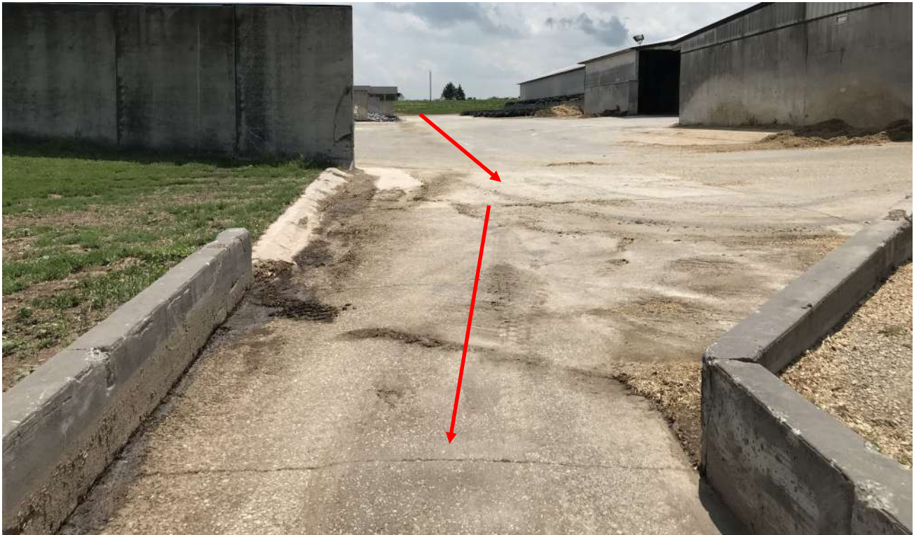
Photo #: 65 Photo Description: The runoff collection system for the east feed storage area. Runoff from the FSA is directed north and into this concrete swale. The red arrows represent the flow path. Date/Time of Photo: 07/07/2020 13:28 Photo Location: Main Site Photo By: James Salscheider
