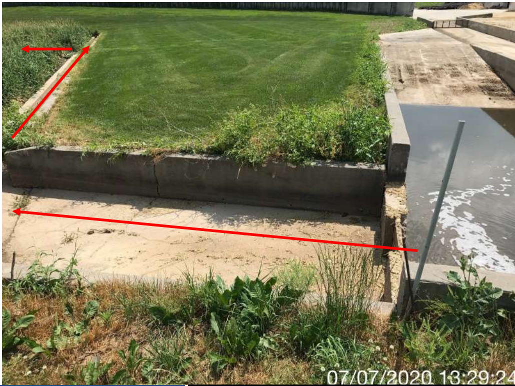
Photo #: 69 Photo Description: The reception basin for the FSA runoff collection system. Runoff from the concrete swale is transferred to this basin and then onto the spreader bar where it then flows through the VTA. The red arrows represent the flow path of runoff. Date/Time of Photo: 07/07/2020 13:29 Photo Location: Main Site Photo By: Brian Hanson
