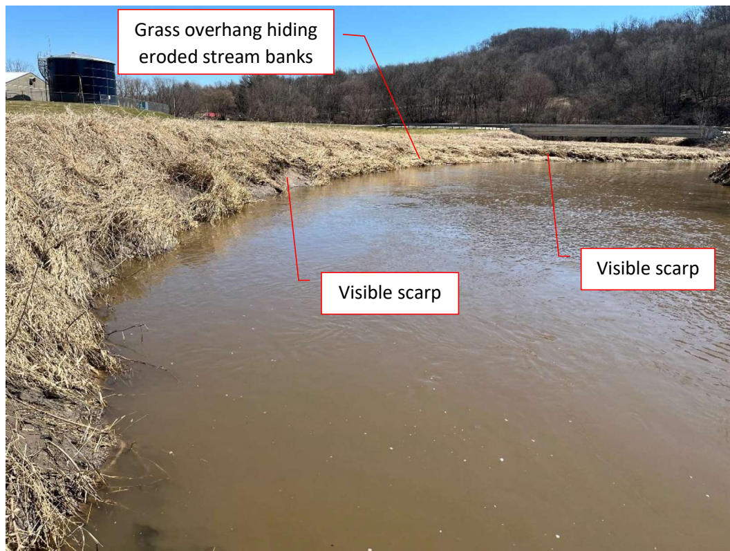
Image 10 – Severe undercut with vegetative overhang. Note that the grass overhang is hiding some of the eroded bank. Severe scarp areas are visible as noted.
