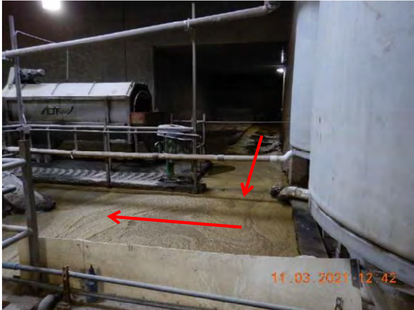
Photo 66. The flow path of manure through the sand separation building at Site 1, represented by the red arrows.
