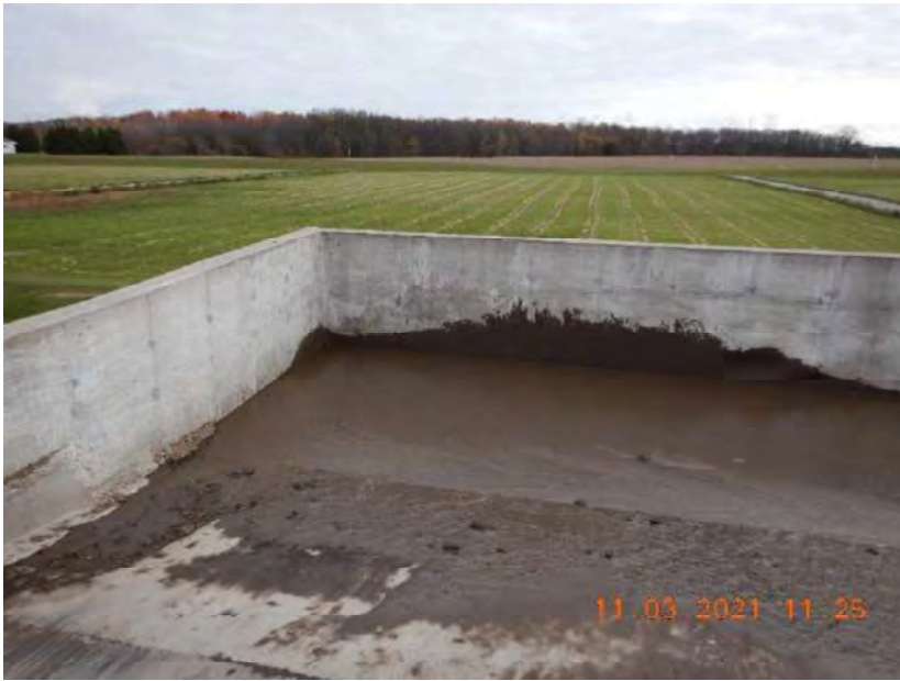
Photo 101. The concrete channel that captures runoff from the feed storage area and conveys it to the runoff collection system. This photo was taken facing south.
