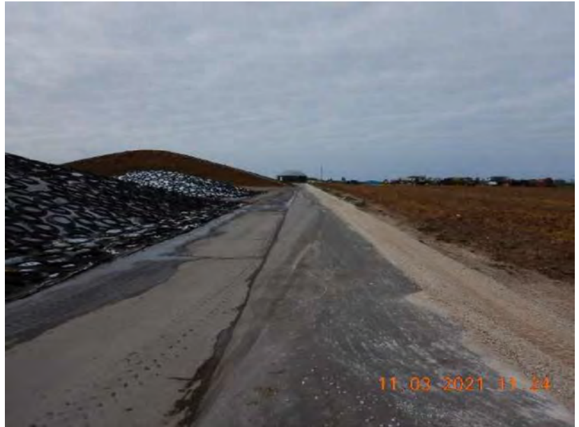
Photo 99. The concrete channel that captures runoff from the feed storage area and conveys it to the runoff collection system. This photo was taken facing south.
