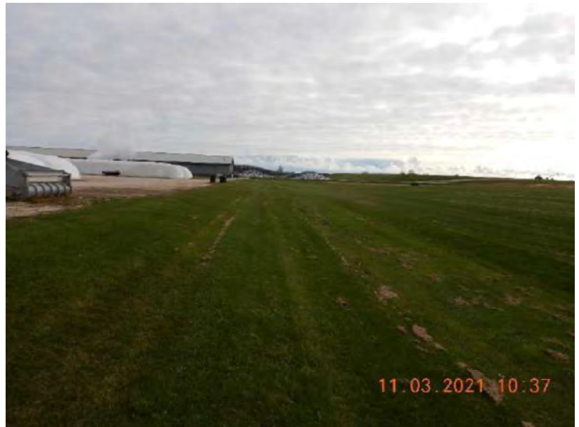
Photo 142. A grassed swale on the south side of the freestall barn at Site 2 that is used to convey stormwater through the production site.
