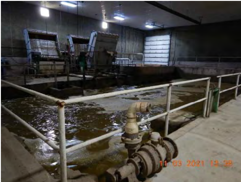
Photo 62. The sand separation building at Site 1. Sand bedding that enters the manure transfer system in the freestall barns at Site 1 is removed, cleaned, and stored in this building, which is located south of the freestall barns.
