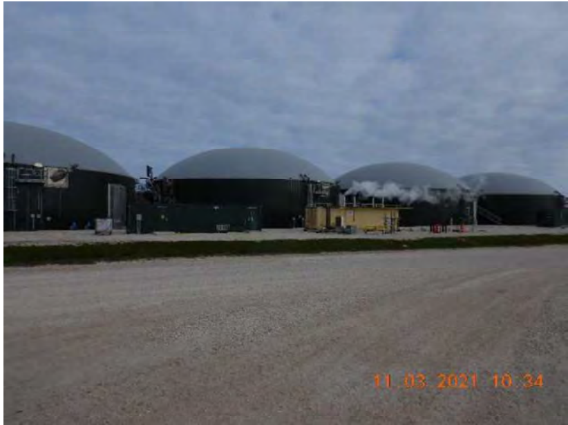
Photo 75. The four anaerobic digesters that are used to digest all manure generated at both sites at Kinnard Farms. The digesters are located on the north side of Site 2. This photo was taken facing west.
