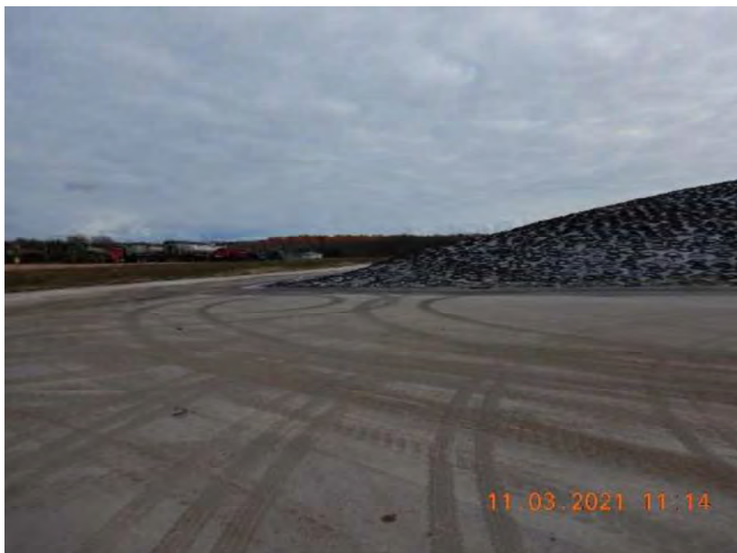
Photo 96. The north side of the feed storage area at Site 2. The concrete pad is pitched from northwest to southeast. This photo was taken facing east.
