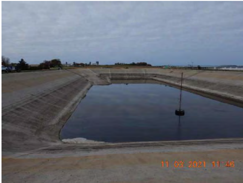
Photo 29. WSF 6 located at the southeast corner of Site 2. WSF 6 is located south of WSF 5 and west of WSF 7. The measuring pole that is used to take weekly measurements can be seen in the middle of the storage. This photo was taken facing southwest.
