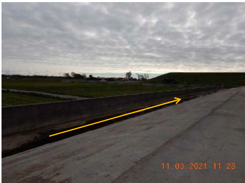
Photo 105. The concrete channel that captures runoff from the feed storage area and conveys it to the runoff collection system. The flow path of runoff is represented by the yellow arrow. This photo was taken facing southeast.
