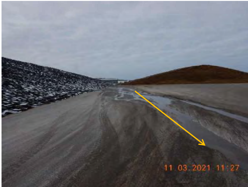
Photo 104. The concrete channel that captures runoff from the feed storage area and conveys it to the runoff collection system. The flow path of runoff is represented by the yellow arrow. This photo was taken facing north.
