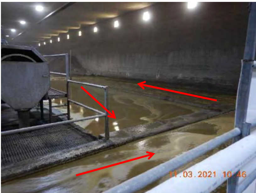
Photo 54. The flow path of manure within the sand separation building, represented by the red arrow.
