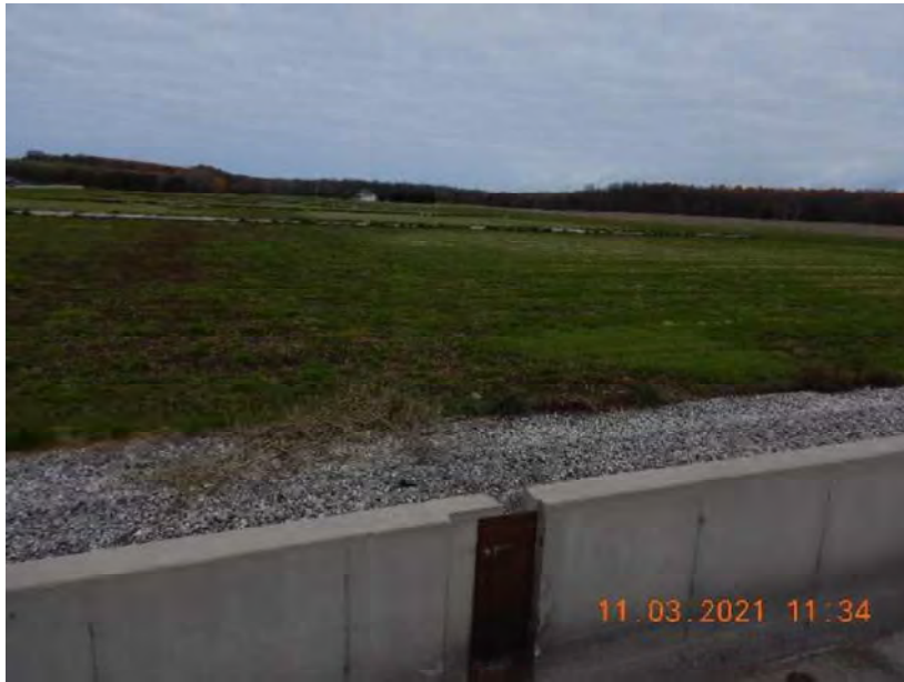
Photo 110. Slots in the concrete spreader bar that are blocked to prevent runoff from entering the VTA.
