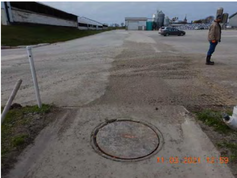
Photo 132. One of two collection inlets for the northern feed storage area at Site 1. This inlet is located at the southeast corner of the storage area. This photo was taken facing west. The inlet was covered to prevent stormwater collection.
