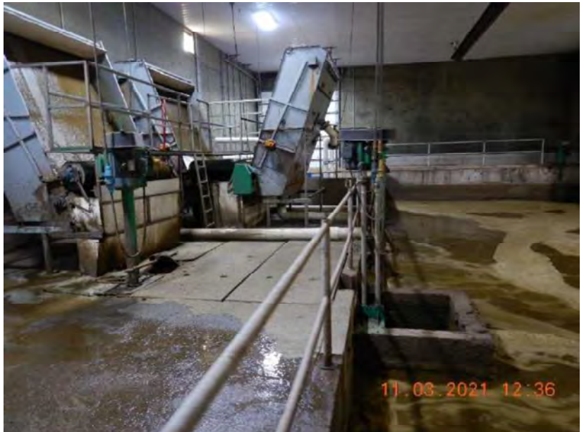
Photo 63. Spilled manure within the sand separation building at Site 1. Any spilled manure gravity flows back into the manure system.
