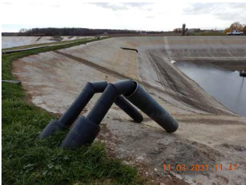
Photo 30. The outlets that discharge runoff into WSF 6 for long term storage. These outlets are located in the northeast corner of WSF 6. This photo was taken facing south.
