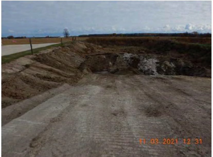
Photo 9. The weir that allows waste from WSF 1 to move to WSF 2, which is located directly south of WSF 1. The red arrow represents the flow path of manure from WSF 1 to WSF 2. This photo was taken facing southeast.
