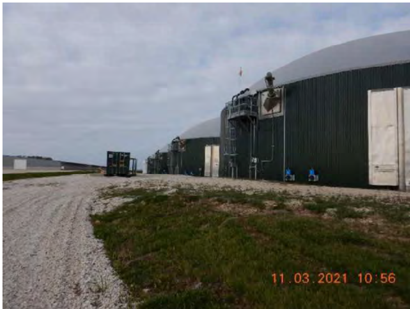
Photo 75. The four anaerobic digesters that are used to digest all manure generated at both sites at Kinnard Farms. The digesters are located on the north side of Site 2. This photo was taken facing west.
