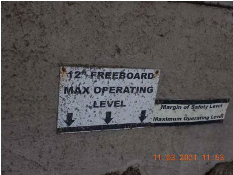
Photo 27. The permanent markers present within WSF 5 at Site 2. The markers do not account for the 25-year, 24-hour runoff collected from the feed storage area.
