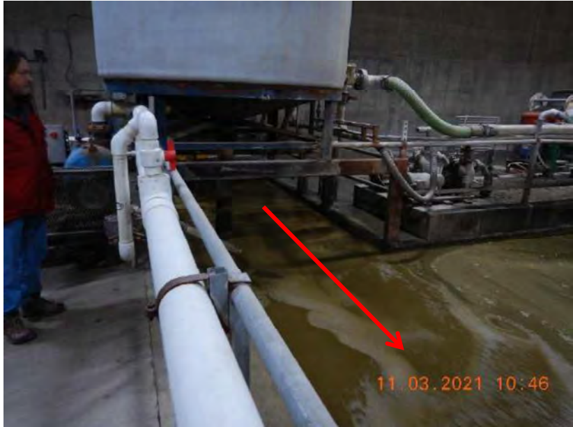
Photo 54. The flow path of manure within the sand separation building, represented by the red arrow.
