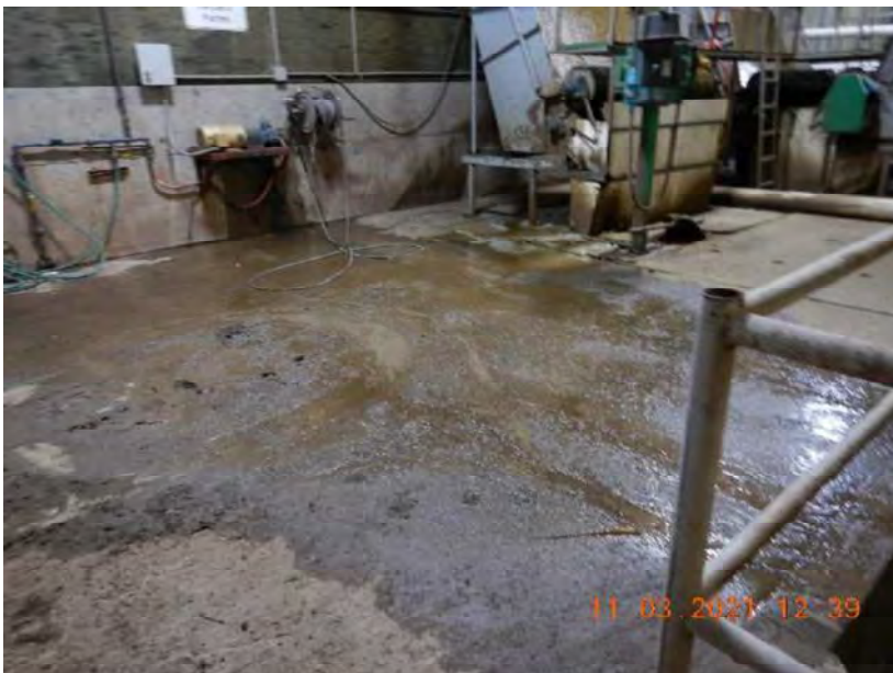
Photo 63. Spilled manure within the sand separation building at Site 1. Any spilled manure gravity flows back into the manure system.
