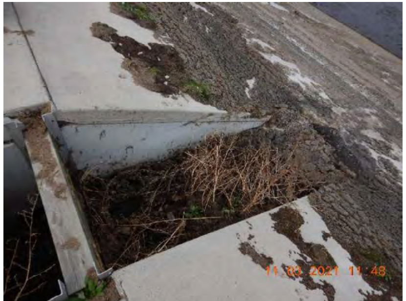
Photo 36. The concrete weir that connects WSF 5 and WSF 6. The weir is used as an emergency transfer system to allow manure to be transferred between the two WSFs. This photo was taken from WSF 6.
