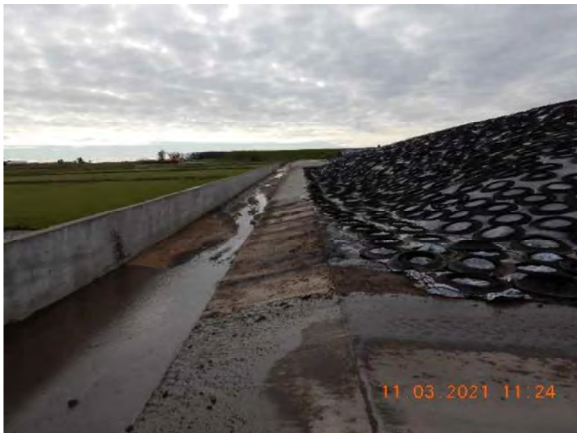
Photo 99. The concrete channel that captures runoff from the feed storage area and conveys it to the runoff collection system. This photo was taken facing south.
