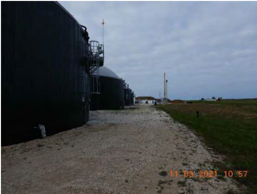
Photo 77. The four anaerobic digesters that are used to digest all manure generated at both sites at Kinnard Farms. The digesters are located on the north side of Site 2. This photo was taken facing south.
