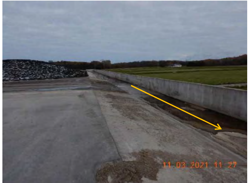
Photo 105. The concrete channel that captures runoff from the feed storage area and conveys it to the runoff collection system. The flow path of runoff is represented by the yellow arrow. This photo was taken facing southeast.
