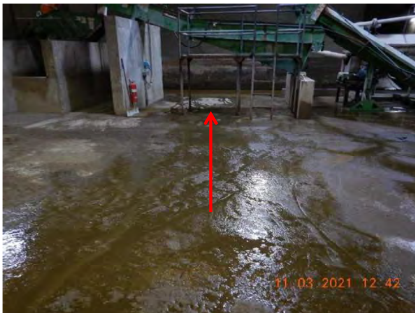
Photo 72. The flow path of runoff from the sand piles directly towards the manure transfer system. The flow path is represented by the red arrows.
