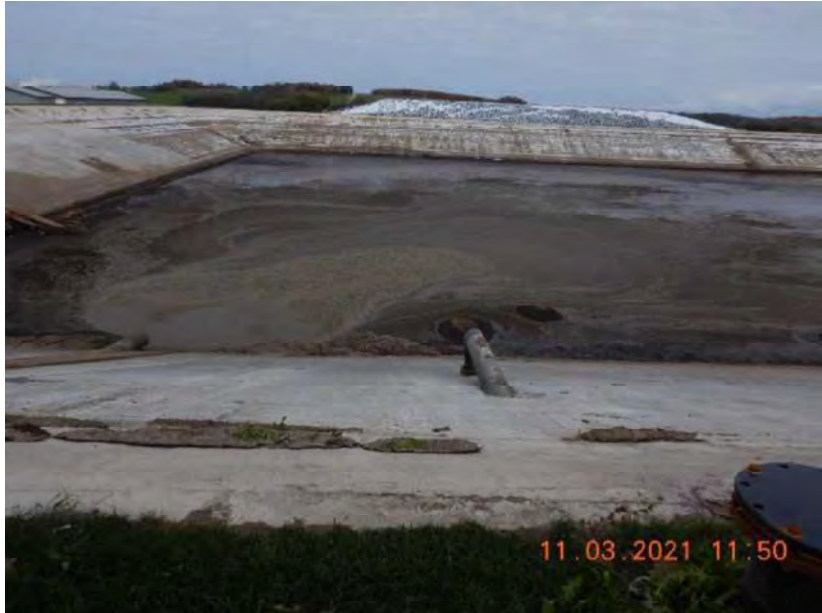
Photo 27. The permanent markers present within WSF 5 at Site 2. The markers do not account for the 25-year, 24-hour runoff collected from the feed storage area.
