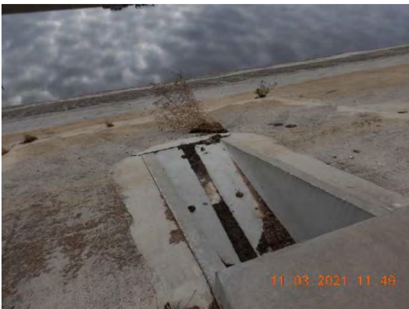
Photo 36. The concrete weir that connects WSF 5 and WSF 6. The weir is used as an emergency transfer system to allow manure to be transferred between the two WSFs. This photo was taken from WSF 6.
