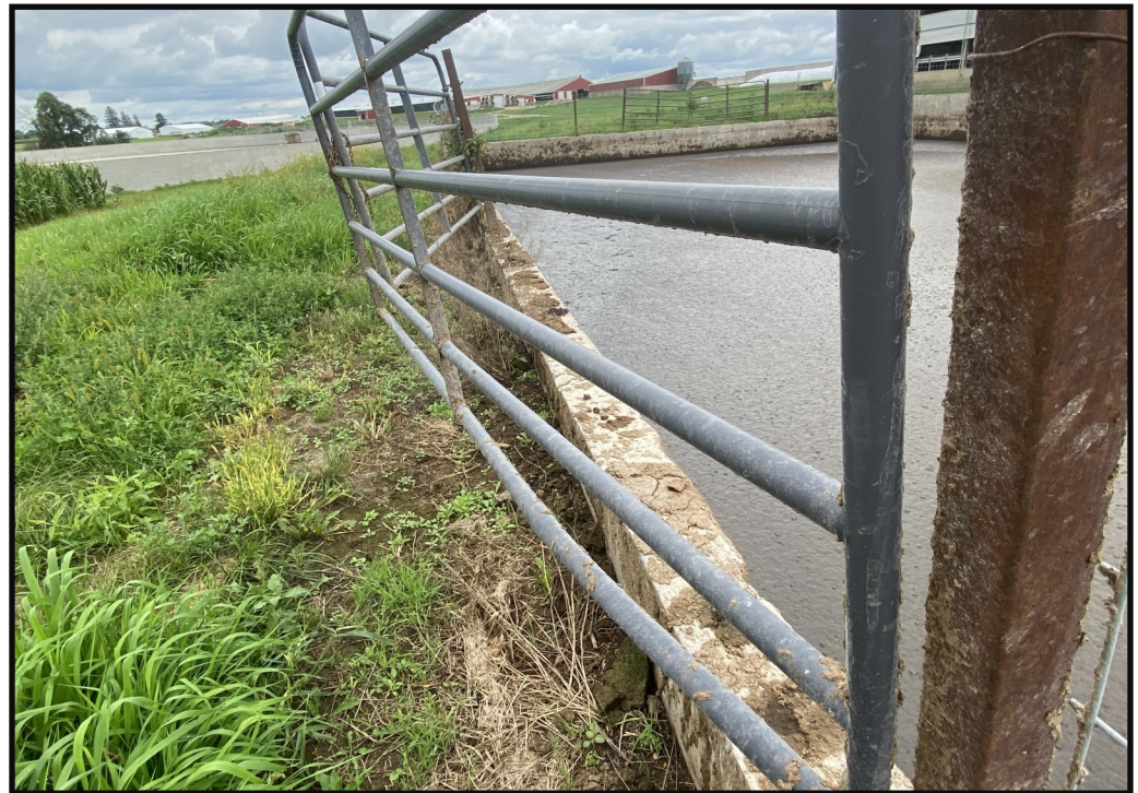
Photo 11 (Right): Looking east along the northern wall of WSF 4. Dried manure solids can be seen along the top edge of the waste storage facility.
