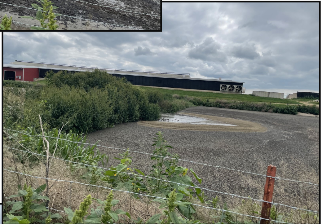
Photo 5 (Right): Looking south along the east end of WSF 2 toward the overflow channel where manure from WSF 1 flows into the waste storage facility. A safety fence was observed around the entire perimeter of WSF 2.
