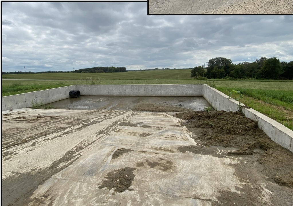
Photo 16 (Bottom Left): Looking south at the feed storage runoff collection basin located toward the center of the south end of the feed storage area. The contents of the runoff collection basin flow through the transfer system to WSF 3.
