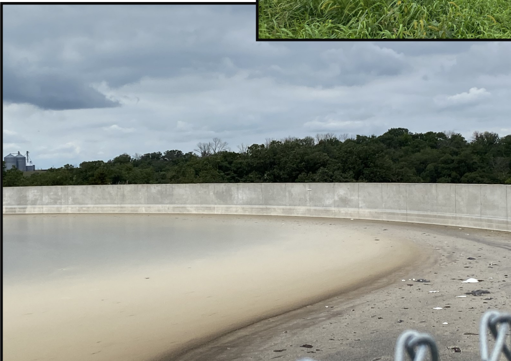
Photo 9 (Bottom Left): Looking north across WSF 3 toward the permanent maximum operating level marker. A permanent margin of safety marker was not present in WSF 3.
