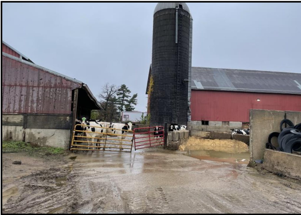
Photo 2 (Top Left): Looking north toward the western end of the outdoor feedlot at the main farm. The operation plans to construct the proposed covered feedlot over this portion of the existing lot which will extend north along the adjacent barn.
