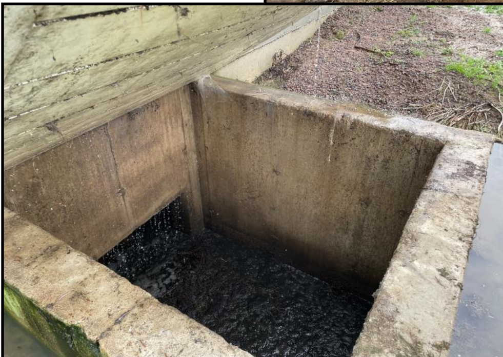
Photo 13 (Bottom Left): Looking into one of the access points to the underbarn storage tanks for the calf barns at the Rowekamp Farm. Liquid manure captured within the underbarn tanks is pumped out from these access points and then land applied.
