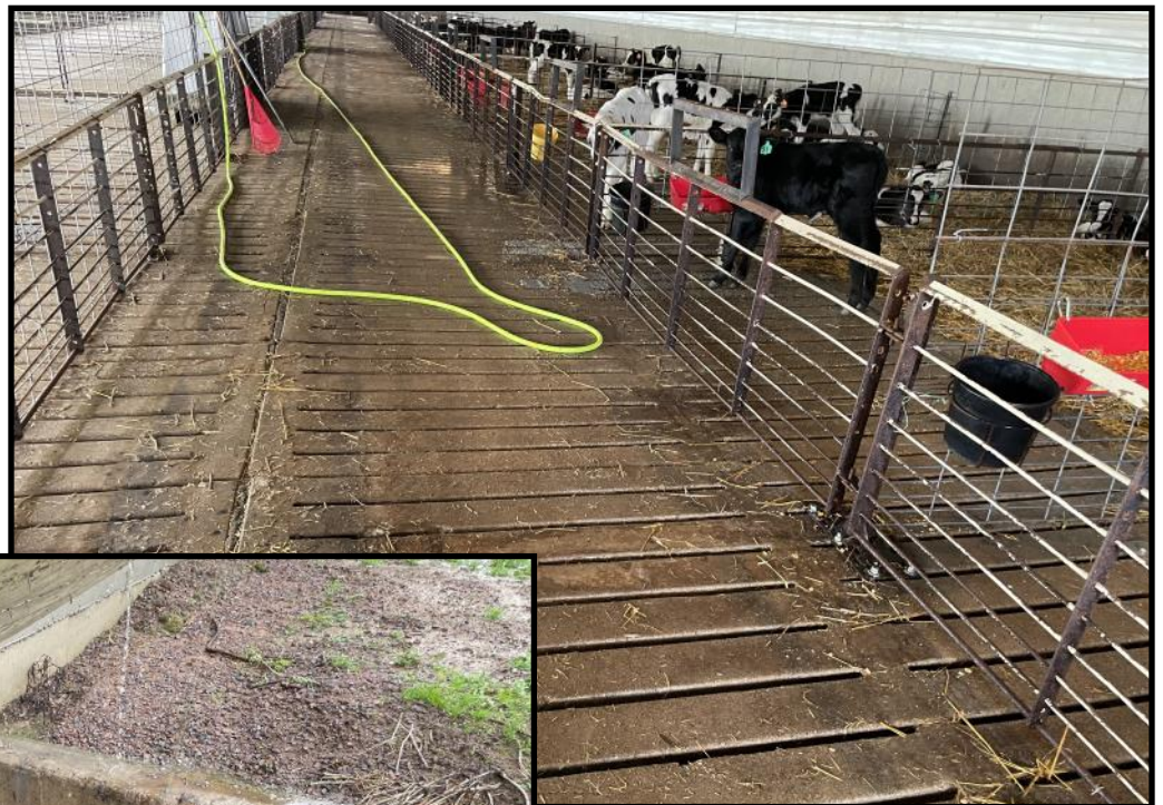
Photo 12 (Right): Looking inside one of the two calf barns at the Rowekamp Farm. The barns have slatted floors with concrete underbarn storage tanks.
