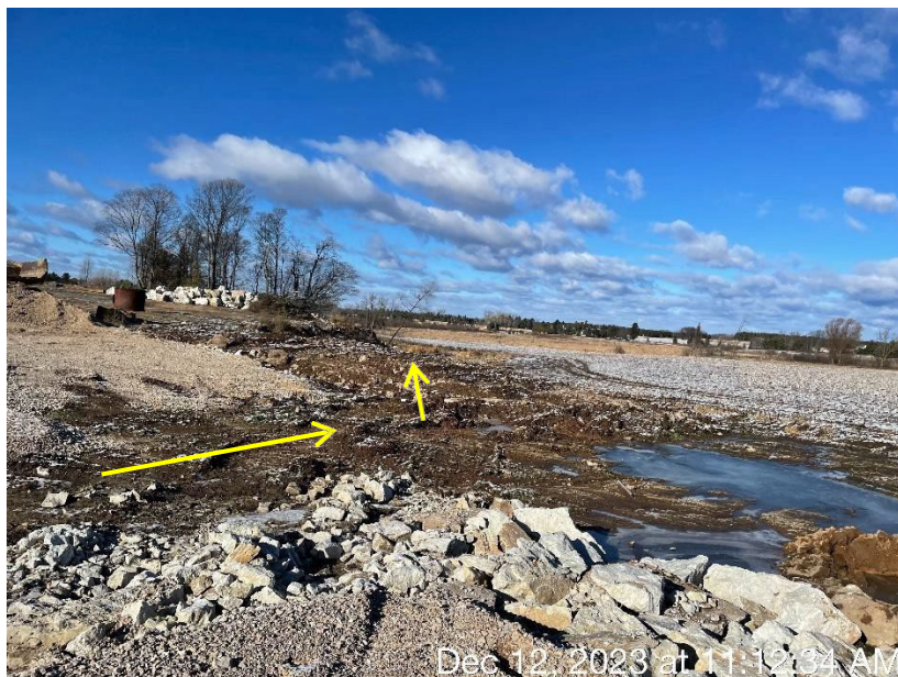
Photo 52. The flow path of runoff off the north side of the feed storage area. The yellow arrows represent the flow path.
