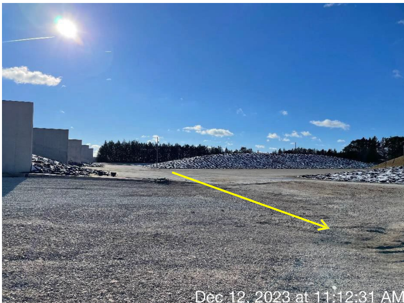
Photo 46. The flow path of runoff from the feed storage area. Runoff concentrates in the middle of the feed pad and flows north off the feed storage area. This photo was taken facing south.
