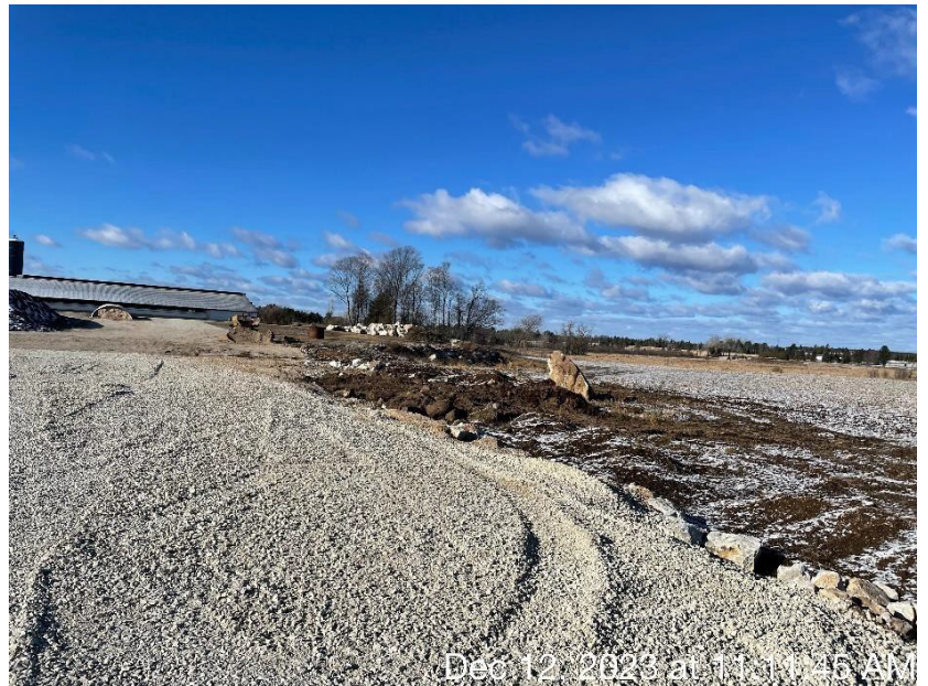
Photo 46. The flow path of runoff from the feed storage area. Runoff concentrates in the middle of the feed pad and flows north off the feed storage area. This photo was taken facing south.
