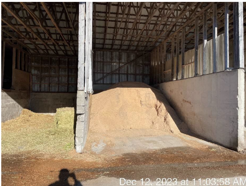
Photo 60. Commodity storage bays at Gilbert Farms.
