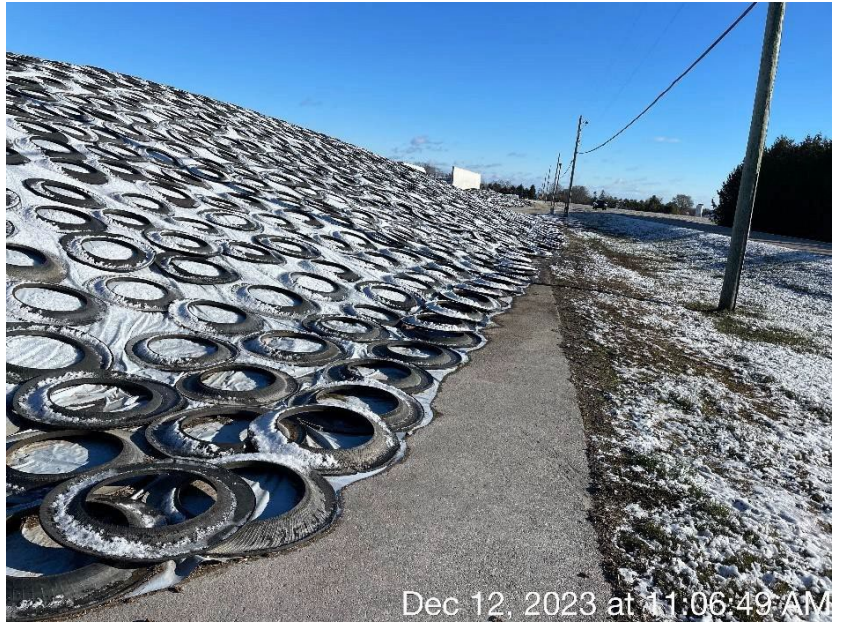
Photo 37. The south side of the feed storage area, where feed was piled along and over the edge of the concrete apron, preventing runoff from staying on the concrete pad.
