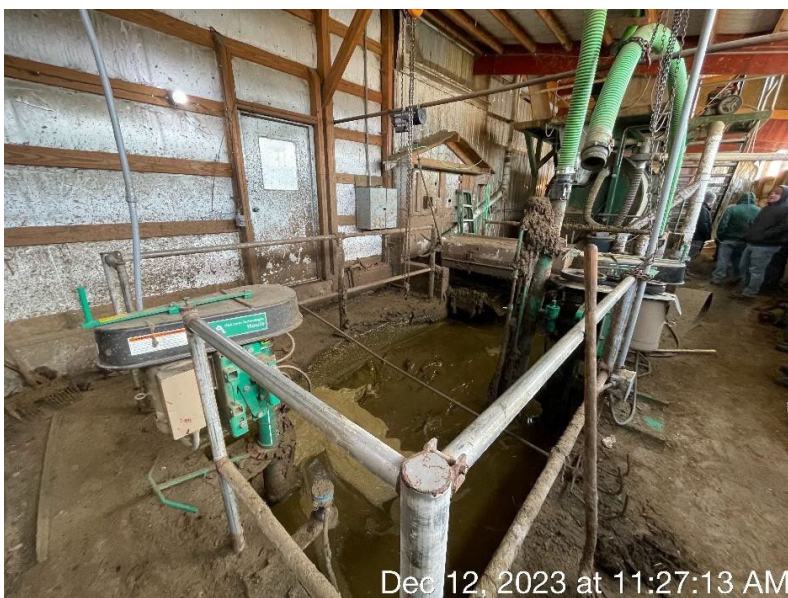
Photo 30. The manure reception tank that accepts manure and process wastewater generated in the freestall barns. Manure is pumped to WSF 1 from this reception tank.
