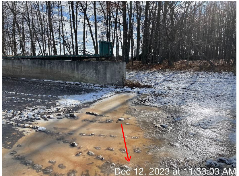
Photo 24. The flow path of runoff from the satellite stacking pad, represented by the red arrows. There are no runoff controls currently in-place.
