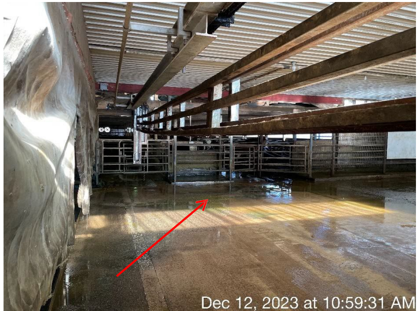
Photo 34. The flow path of process wastewater generated in the parlor. It is washed into the adjacent freestall barn and comingled with manure.
