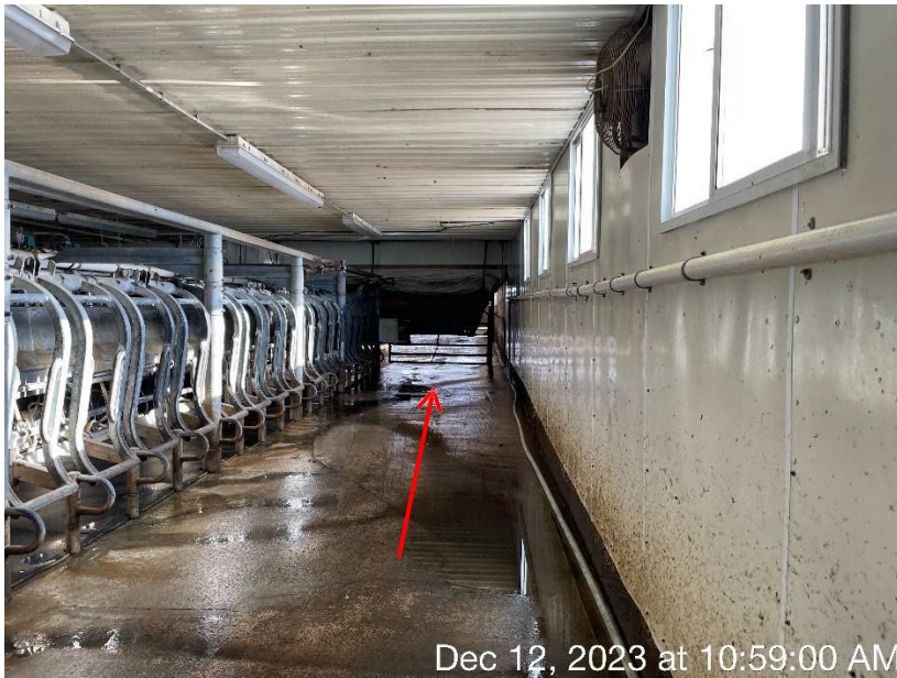
Photo 34. The flow path of process wastewater generated in the parlor. It is washed into the adjacent freestall barn and comingled with manure.
