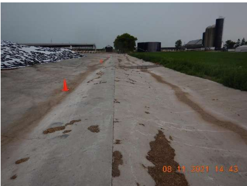
Photo 22. The concrete swale that conveys runoff from the calf hutch area to the vegetated treatment area. Runoff flows south on the swale towards the VTA. A concrete berm separates the feed storage area and the concrete swale. This photo was taken facing north.
