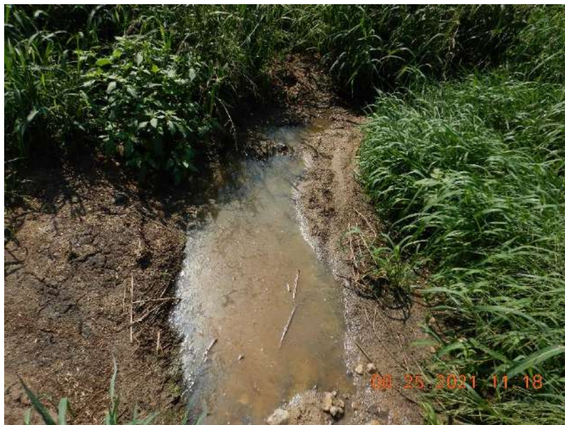
Photo 87. Runoff within the grassed swale that conveys wastewater to the detention basin.
