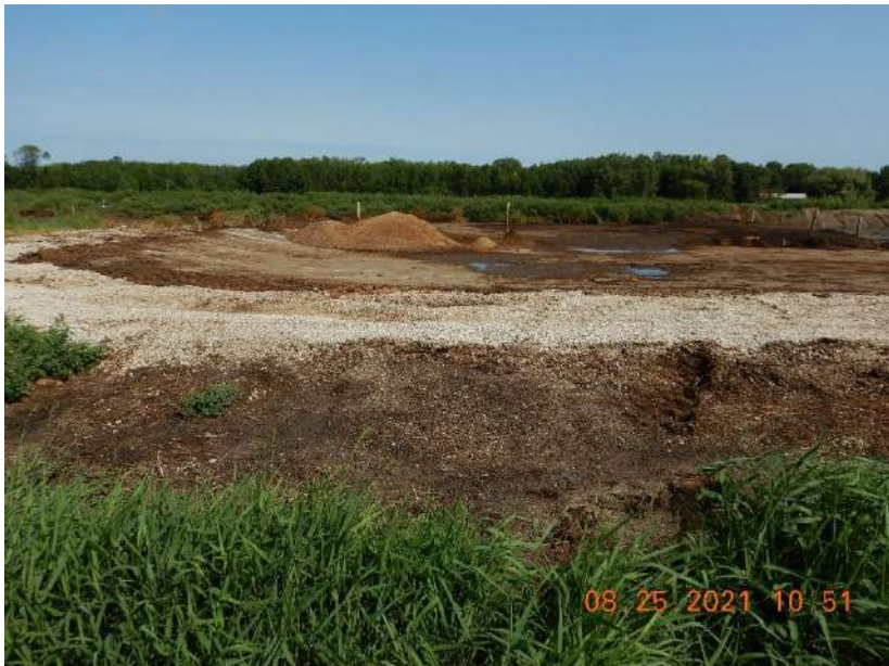
Photo 65. The south side of the solid manure stacking pad located south of WSF 2. Runoff and solids were present outside of the stacking area. This photo was taken facing north.
