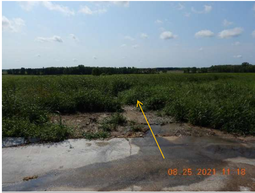
Photo 86. The grassed swale that conveys runoff from the east side of the feed storage area to the detention basin, located south of the FSA. The yellow arrows represent the flow path of runoff. This photo was taken facing southwest.
