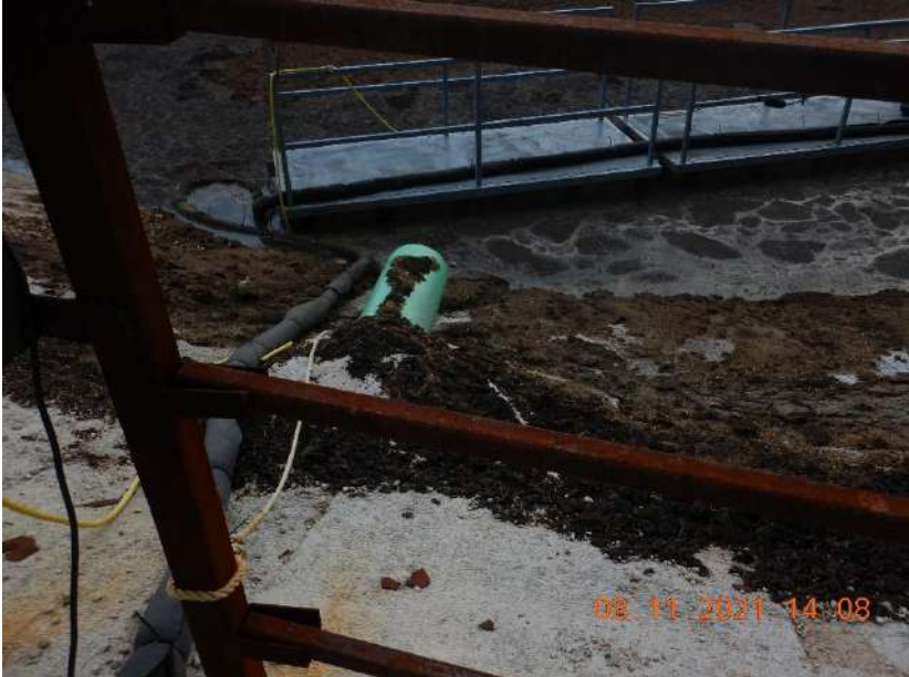
Photo 47. The outlet that discharges manure that is transferred from the sand separation building.
