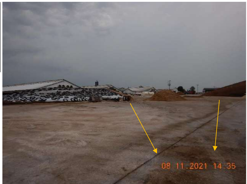
Photo 75. The feed storage area at the Main Site. Runoff flows from north to south and enters one of two runoff control systems. The yellow arrows represent the flow path of runoff. This photo was taken facing north.
