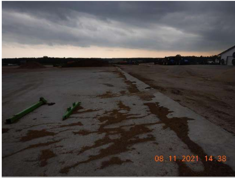
Photo 80. The feed storage area at the Main Site. The concrete pad was in good condition with no signs of degradation.
