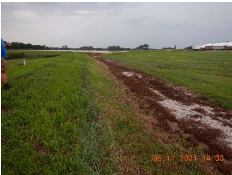
Photo 93. The detention basin located south of the leachate basin and feed storage area. The detention basin accepts overflow from the leachate basin and runoff from the east side of the feed storage area. This photo was taken facing east.
