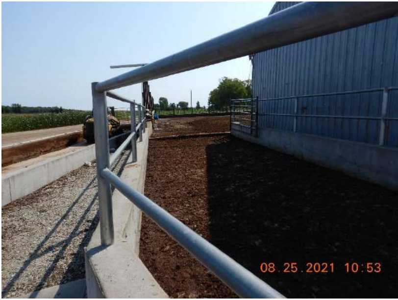
Photo 8. A concrete swale located north of the outdoor feedlot at the Heifer Site. Runoff from the feedlot gravity flows through the swale and into the onsite liquid waste storage facility. This photo was taken facing east.
