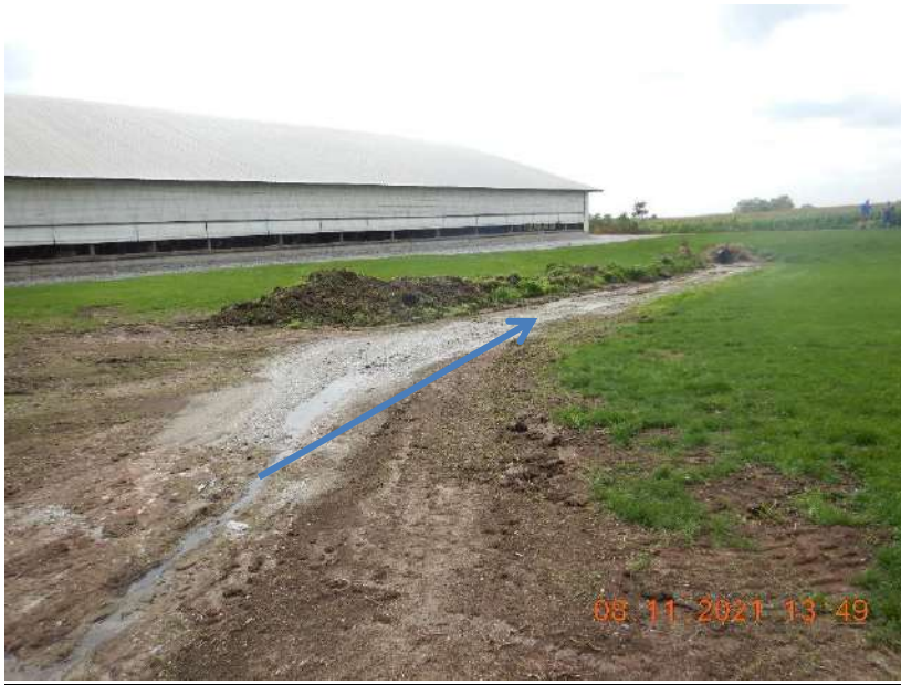
Photo 114. A grassed stormwater swale at the Heifer Site that conveys clean water off-site. The blue arrow represents the flow path of stormwater through the swale. This photo was taken facing west.
