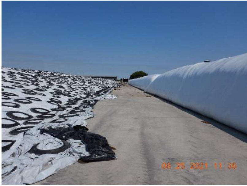
Photo 84. The east side of the feed storage area at the Main Site, where runoff flows from north to south and enters a grassed swale that conveys runoff to the detention basin, located south of the FSA.
