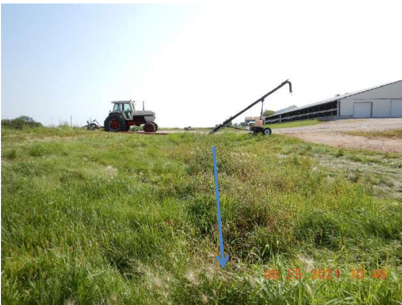
Photo 115. A grassed stormwater swale at the Heifer Site that conveys clean water off-site. The blue arrow represents the flow path of stormwater through the swale. This photo was taken facing east.
