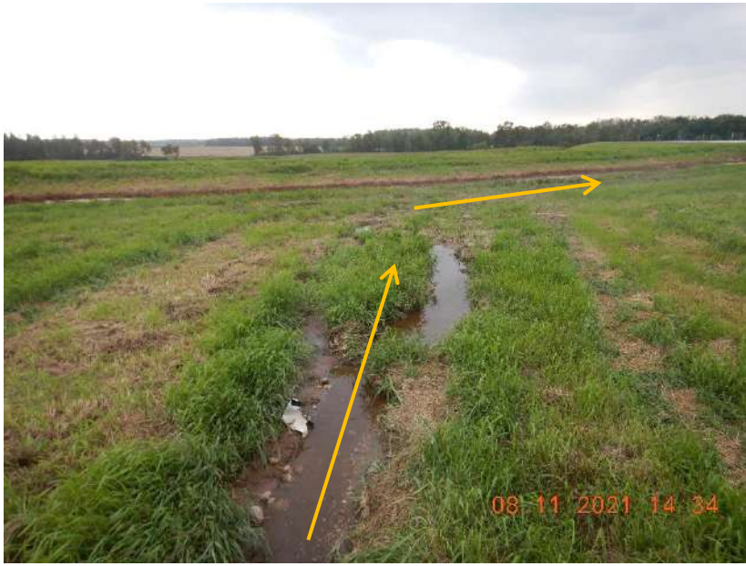
Photo 92. The detention basin located south of the leachate basin and feed storage area. The detention basin accepts overflow from the leachate basin and runoff from the east side of the feed storage area. This photo was taken facing east.
