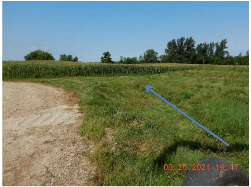
Photo 115. A grassed stormwater swale at the Heifer Site that conveys clean water off-site. The blue arrow represents the flow path of stormwater through the swale. This photo was taken facing east.
