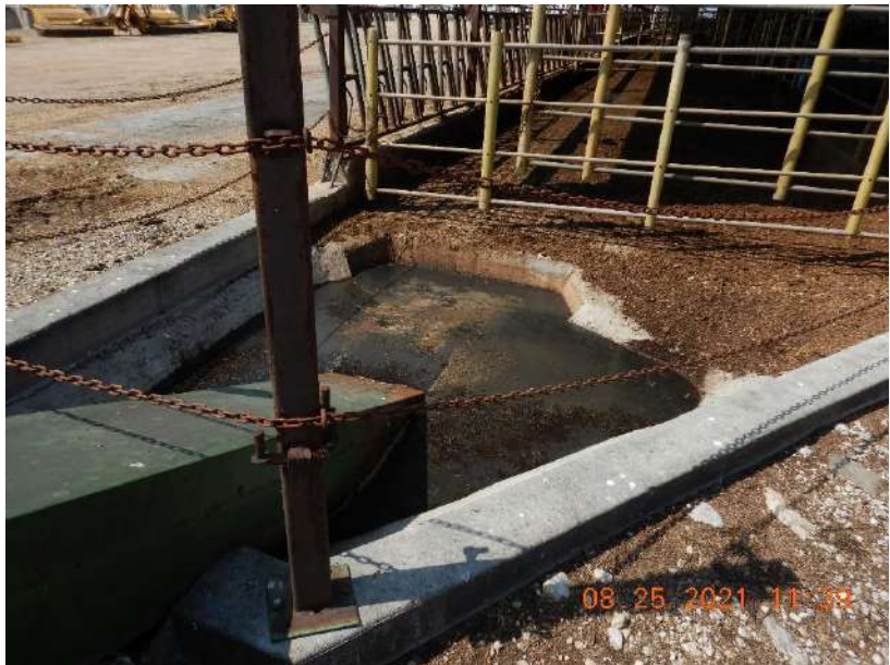
Photo 73. A reception basin at the east end of the heifer barn at the Main Site. Runoff enters the basin and is pumped directly to a manure tanker.
