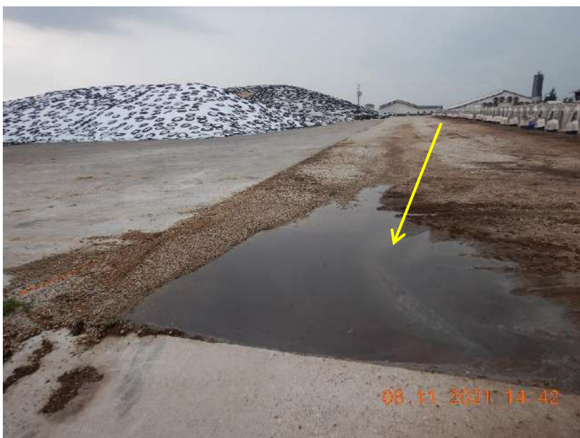
Photo 19. The outdoor calf hutch area located north of the feed storage area at the Main Site. Runoff from the calf hutch area flows east and south towards the runoff collection system. This photo was taken facing west. The yellow arrow represents the flow path of runoff towards the runoff control system. The ponded area in the foreground allows sediment to settle out prior to entering the concrete swale.
