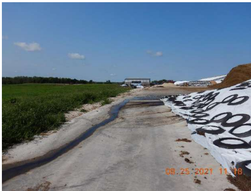
Photo 84. The east side of the feed storage area at the Main Site, where runoff flows from north to south and enters a grassed swale that conveys runoff to the detention basin, located south of the FSA.
