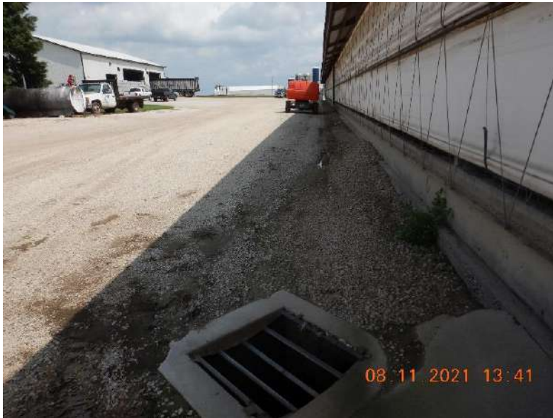
Photo 108. A stormwater inlet that accepts clean water from a driveway at the Main Site and diverts the water off-site. A tile line discharges roof runoff to the inlet.
