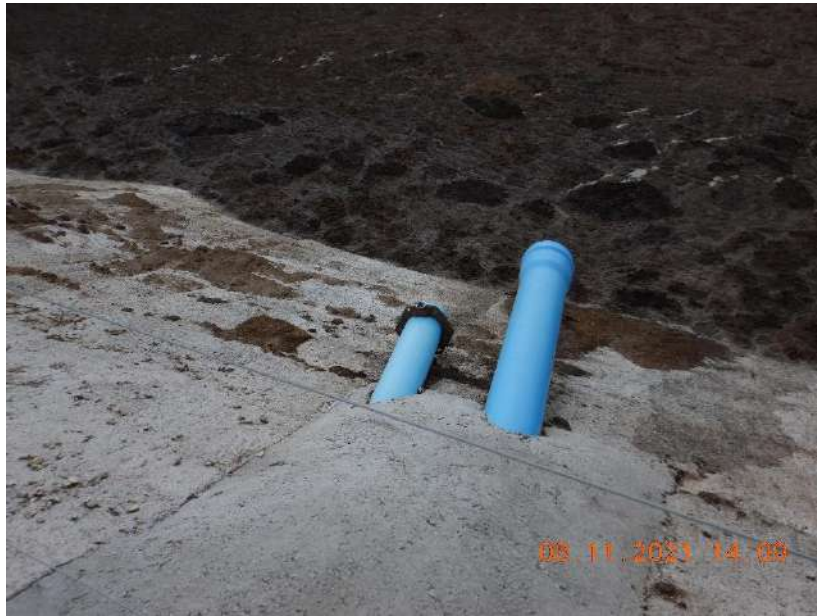
Photo 46. The outlet of the overflow transfer pipe from WSF 1.
