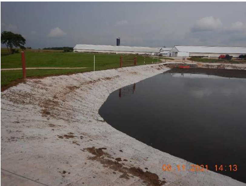
Photo 41. WSF 3 at the Main Site, located on the south side of the production site. WSF 3 is a concrete structure built in 2020. This photo was taken facing north.
