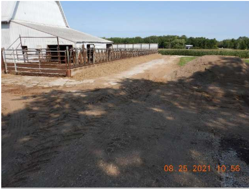
Photo 13. The outdoor feedlot at the Heifer Site. Runoff flows north towards the runoff control system, represented by the yellow arrows. This photo was taken facing north.
