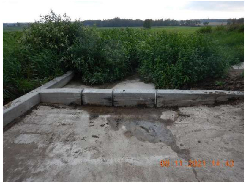
Photo 25. The end of the concrete swale where runoff from the calf hutch area enters the VTA.
