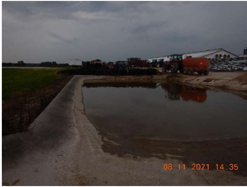
Photo 89. The leachate basin that is located on the south side of the feed storage area. The leachate basin accepts leachate and first flush from the west side of the FSA. Runoff overflows via the toe drain on the southeast corner of the basin and flows to the detention basin. The VAC truck that transfers waste to the onsite WSFs can be seen in the photo. This photo was taken facing west.
