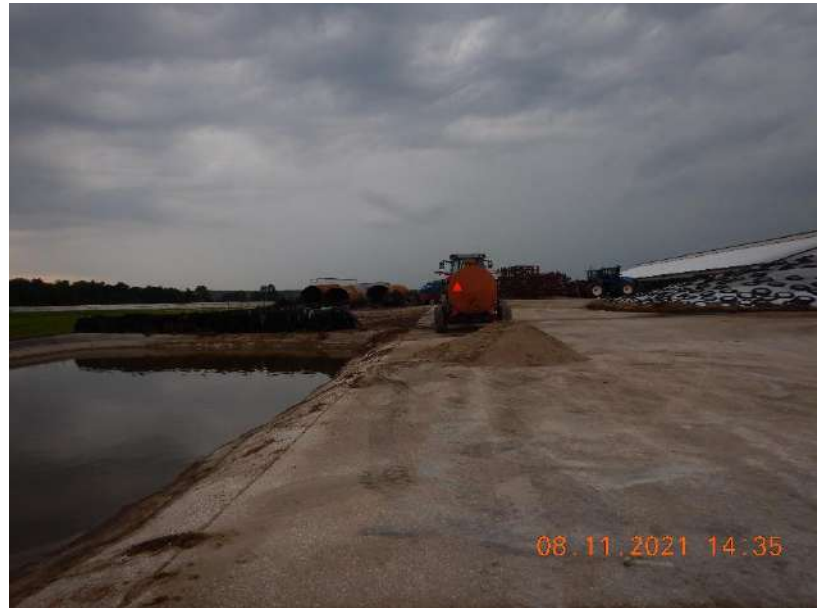
Photo 89. The leachate basin that is located on the south side of the feed storage area. The leachate basin accepts leachate and first flush from the west side of the FSA. Runoff overflows via the toe drain on the southeast corner of the basin and flows to the detention basin. The VAC truck that transfers waste to the onsite WSFs can be seen in the photo. This photo was taken facing west.
