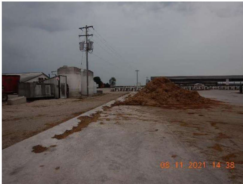
Photo 78. The feed storage area at the Main Site. Concrete curbing on the west side of the FSA prevents runoff from discharging and conveys the runoff to the runoff control system. This photo was taken facing north.
