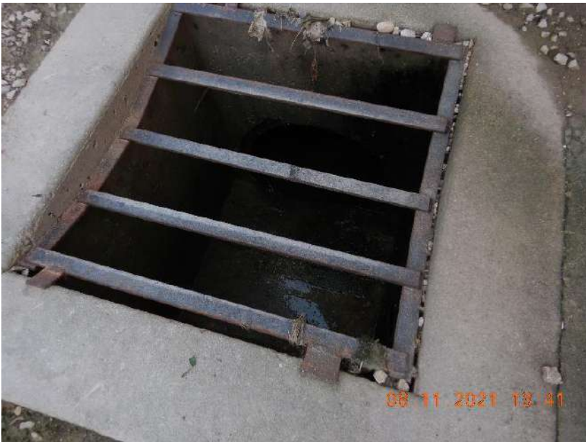
Photo 106. A stormwater inlet that accepts clean water from a driveway at the Main Site and diverts the water off-site.
