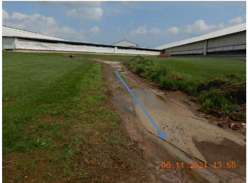
Photo 112. A stormwater culvert that discharge clean water to the grassed channel pictured in Photo 106. The blue arrow represents the flow path of stormwater.
