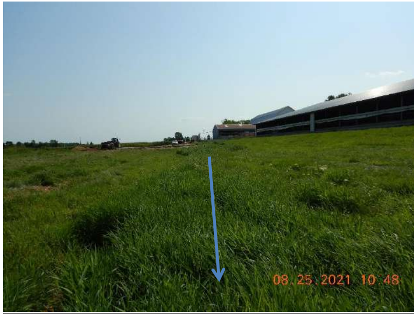
Photo 117. A grassed stormwater swale at the Heifer Site that conveys clean water off-site. The blue arrow represents the flow path of stormwater through the swale. This photo was taken facing west.
