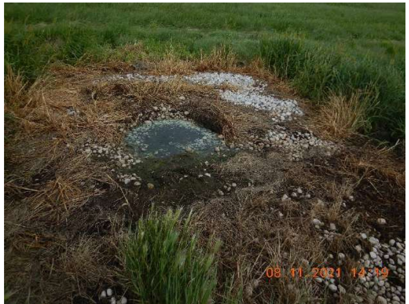
Photo 96. One of five bubblers that are used to evenly distribute runoff across the vegetate treatment area.
