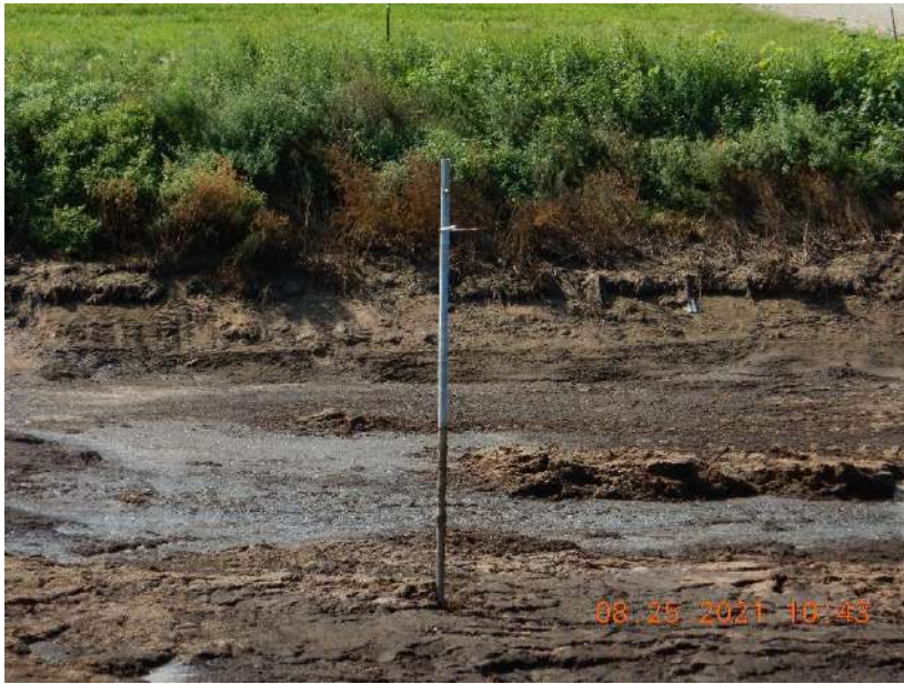
Photo 61. The west side of the solid manure stacking pad located south of WSF 2. Runoff from the stacking pad flows north directly into WSF 2. This photo was taken facing east.
