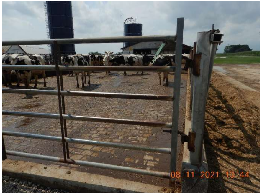
Photo 2. The outdoor concrete feedlot located at the Main Site. The feedlot is located on the north side of the production site. Runoff from the feedlot gravity flows to the center, where it collected until it is augered into equipment to transfer the waste. This photo was taken facing west.
