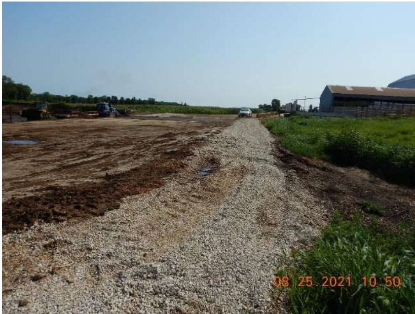
Photo 64. The solid manure stacking pad located south of WSF 2. Runoff from the stacking pad flows north directly into WSF 2. This photo was taken facing north.
