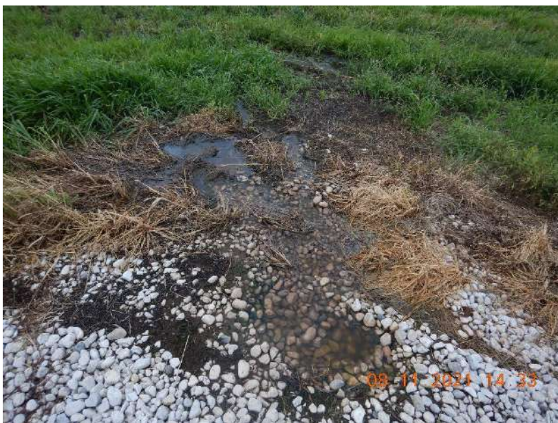
Photo 96. One of five bubblers that are used to evenly distribute runoff across the vegetate treatment area.
