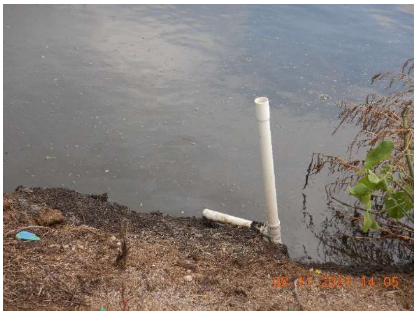
Photo 38. The maximum operating level (MOL) marker present within WSF 1 at the Main Site. The marker is present within the western berm.
