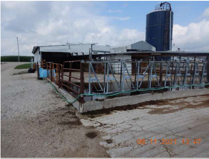
Photo 7. The outdoor feedlot at the Heifer Site. Runoff from the feedlot gravity flows through a series of concrete swales and into the onsite liquid waste storage facility. This photo was taken facing east.
