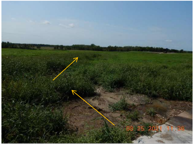
Photo 87. Runoff within the grassed swale that conveys wastewater to the detention basin.
