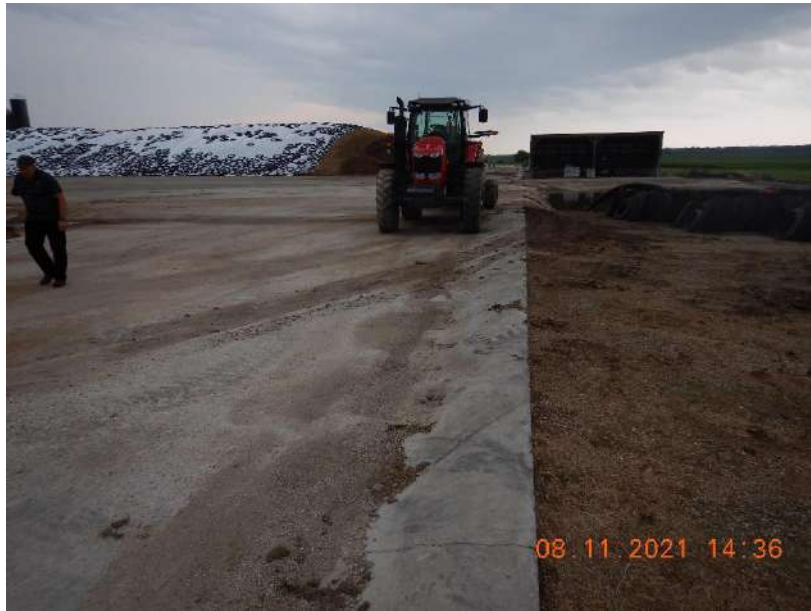
Photo 77. The feed storage area at the Main Site. The concrete pad was in good condition with no signs of degradation.
