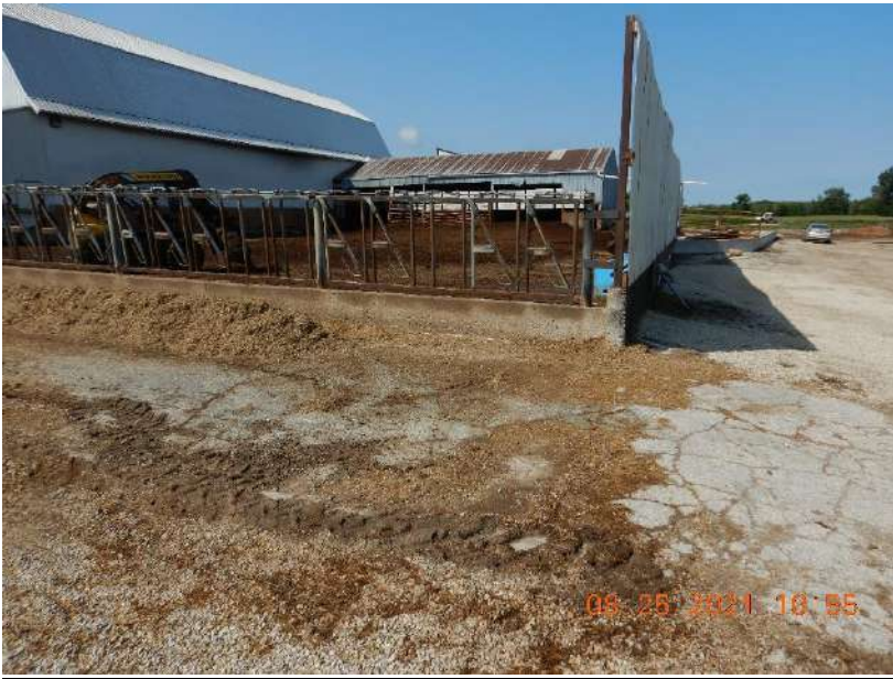
Photo 10. The outdoor concrete feedlot at the Heifer Site. Runoff from the feedlot flows northwest through a series of concrete swales that gravity flow to the onsite liquid waste storage facility. This photo was taken facing west.
