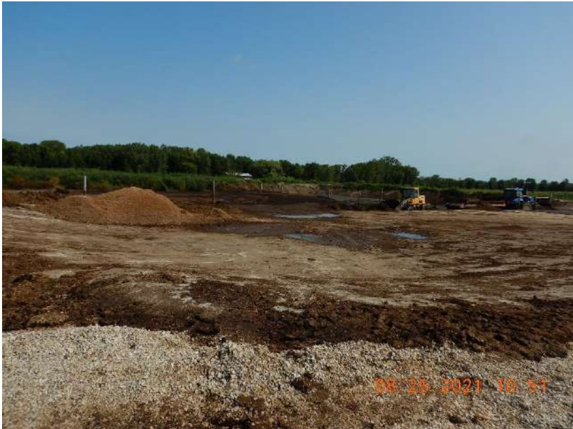
Photo 65. The south side of the solid manure stacking pad located south of WSF 2. Runoff and solids were present outside of the stacking area. This photo was taken facing north.
