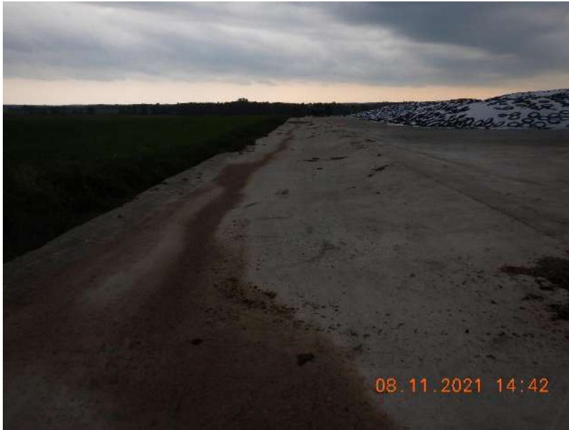
Photo 21. The concrete swale that conveys runoff from the calf hutch area to the vegetated treatment area. A concrete bar allows solids to settle out and liquid to continue south towards the VTA. This photo was taken facing south.
