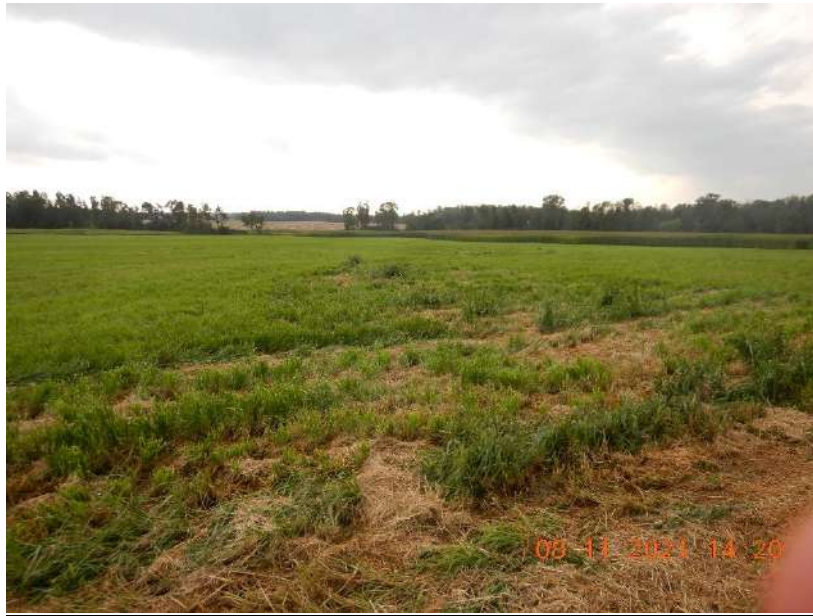
Photo 98. The vegetated treatment area located south of the detention basin. One concentrated flow channel was present from one of the bubblers, as its elevation is lower than the rest resulting in more runoff being discharged from the bubbler. This photo was taken facing south.
