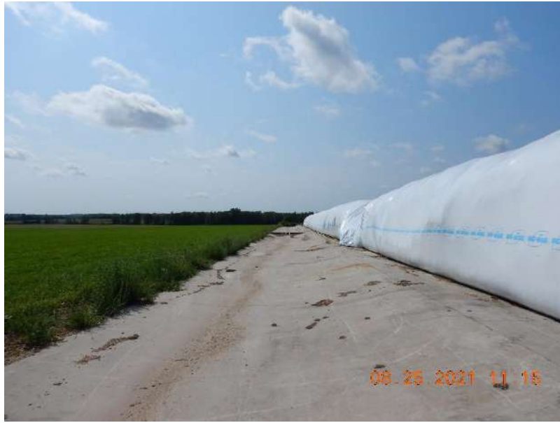
Photo 83. The east side of the feed storage area at the Main Site. The concrete pad was in good condition with no signs of degradation.
