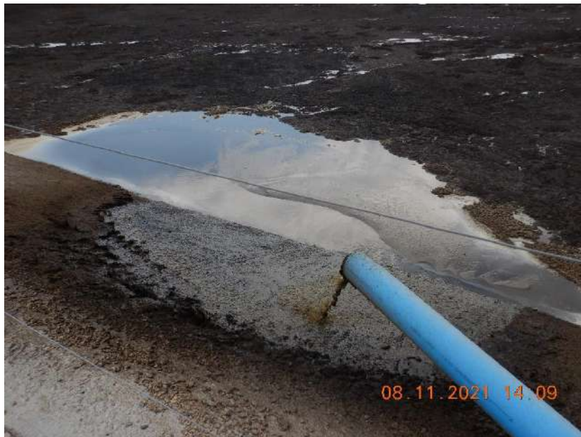
Photo 47. The outlet that discharges manure that is transferred from the sand separation building.
