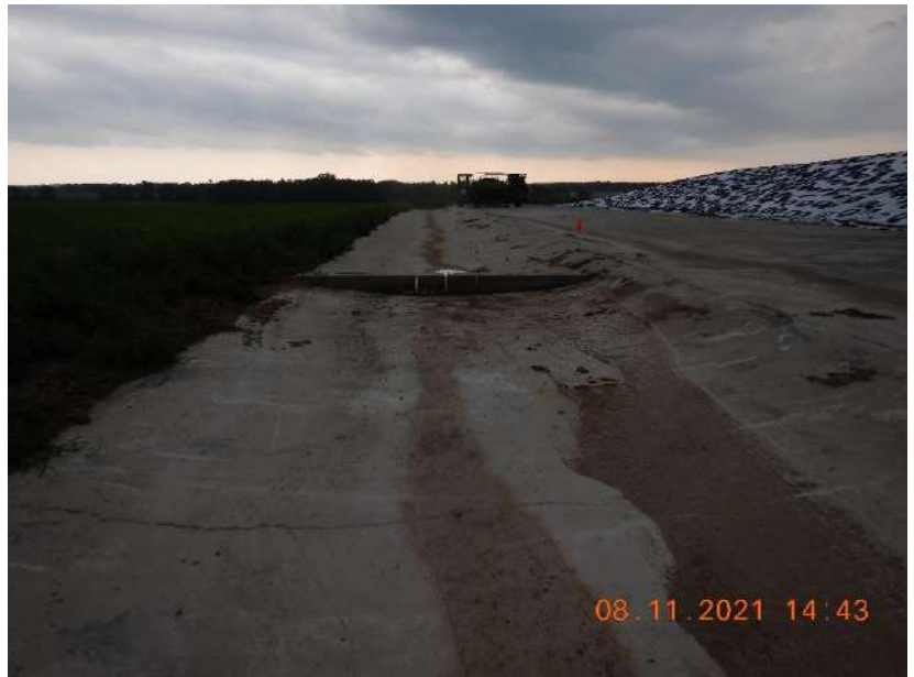
Photo 22. The concrete swale that conveys runoff from the calf hutch area to the vegetated treatment area. Runoff flows south on the swale towards the VTA. A concrete berm separates the feed storage area and the concrete swale. This photo was taken facing north.
