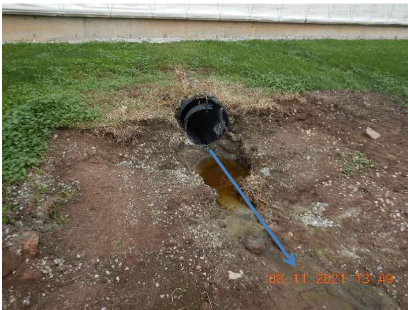
Photo 112. A stormwater culvert that discharge clean water to the grassed channel pictured in Photo 106. The blue arrow represents the flow path of stormwater.
