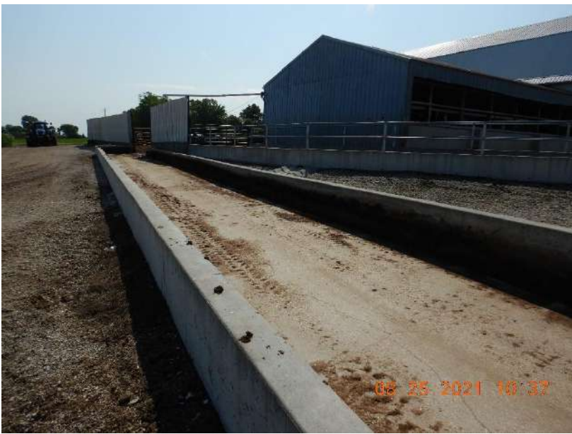
Photo 8. A concrete swale located north of the outdoor feedlot at the Heifer Site. Runoff from the feedlot gravity flows through the swale and into the onsite liquid waste storage facility. This photo was taken facing east.
