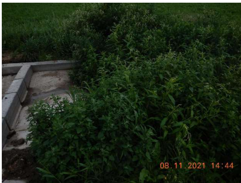
Photo 25. The end of the concrete swale where runoff from the calf hutch area enters the VTA.
