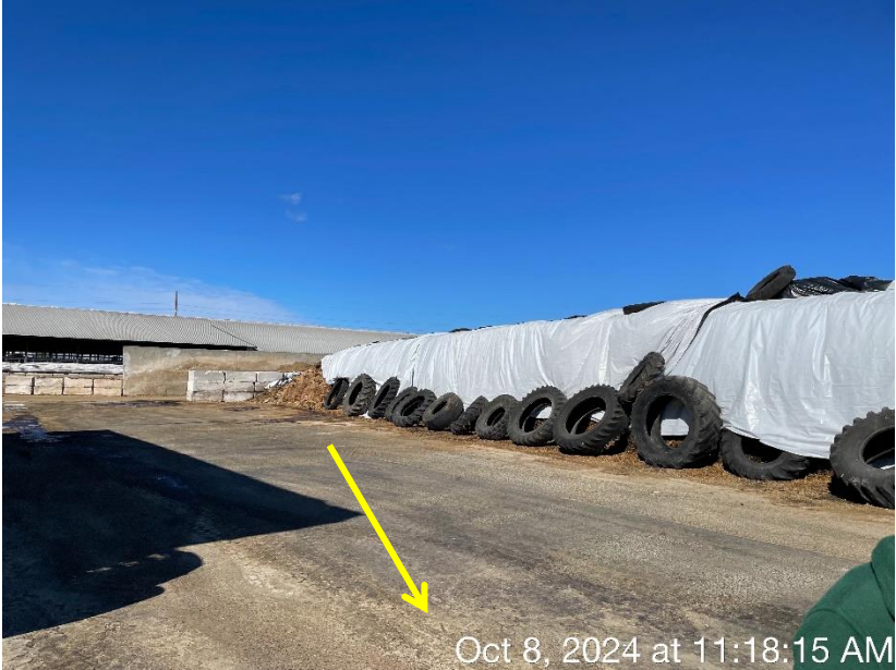
Photo 84. The flow path of runoff on the feed storage area at the Longfellow Site. Runoff gravity flows east towards the collection system.
