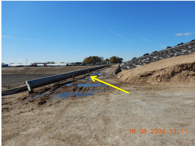
Photo 77. The flow path of runoff towards the collection system, located on the south side of the feed storage area.
