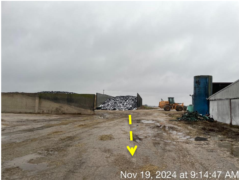
Photo 38. The flow path of runoff on the feed storage area towards the collection inlet located on the east side of the storage area.
