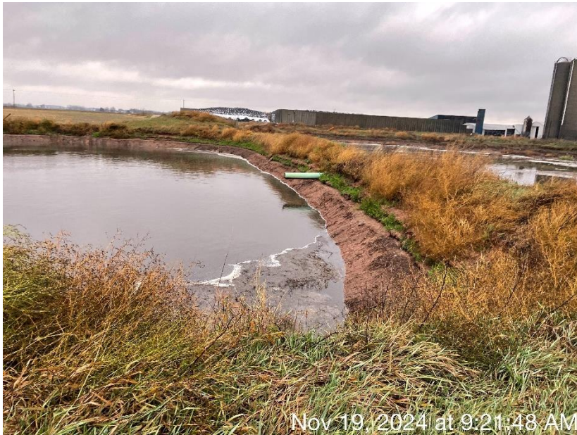
Photo 13. The solid stacking area located on the south side of WSF 2 at the East Site. Runoff from the stacking area gravity flows into WSF 2.
