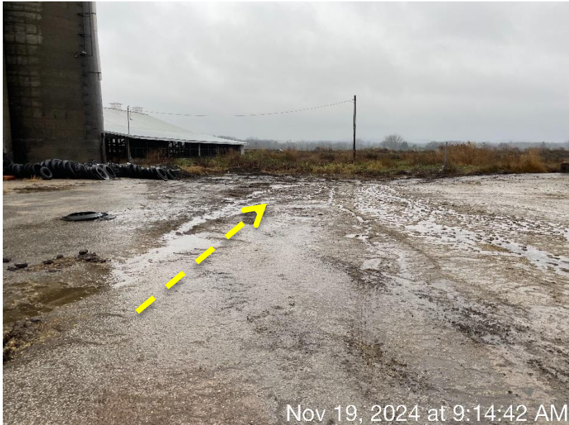
Photo 39. The collection inlet that accepts runoff from the feed storage area and conveys the runoff to WSF 3.
