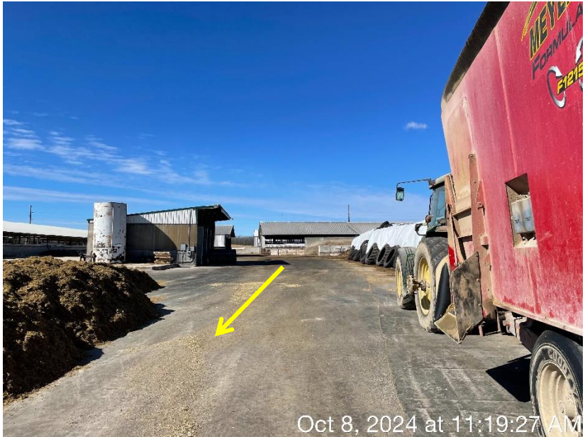
Photo 84. The flow path of runoff on the feed storage area at the Longfellow Site. Runoff gravity flows east towards the collection system.
