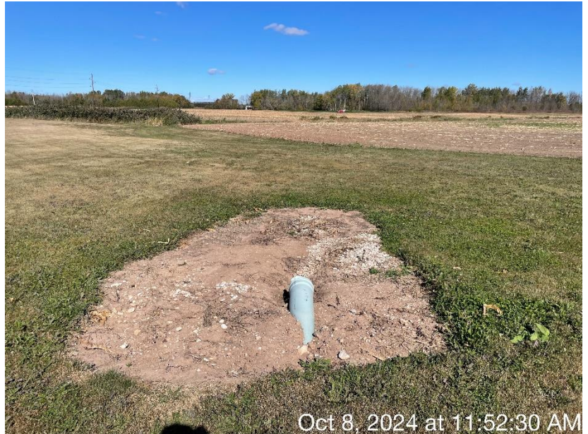
Photo 109. A stormwater outlet located between the calf barns on the south side of the production site at the Main Site. The inlet accepts runoff from the driveway and barn roofs and conveys the runoff to the southern stormwater pond.
