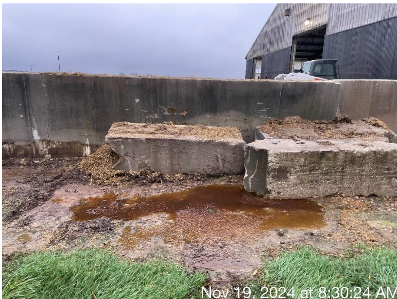
Photo 47. A small amount of process wastewater present on the back side of the push wall pictured in Photo 46.
