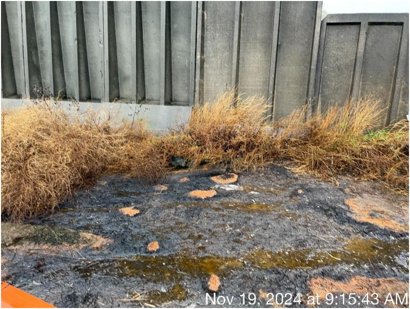
Photo 42. Leachate that seeped through the concrete wall on the east side of the feed storage area.
