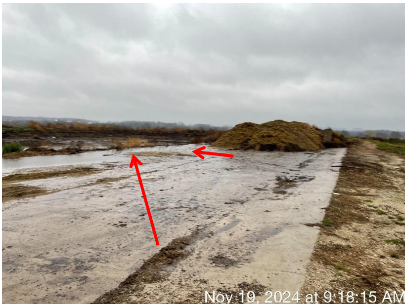
Photo 14. The flow path of runoff from the stacking area into WSF 2. This photo was taken facing east.
