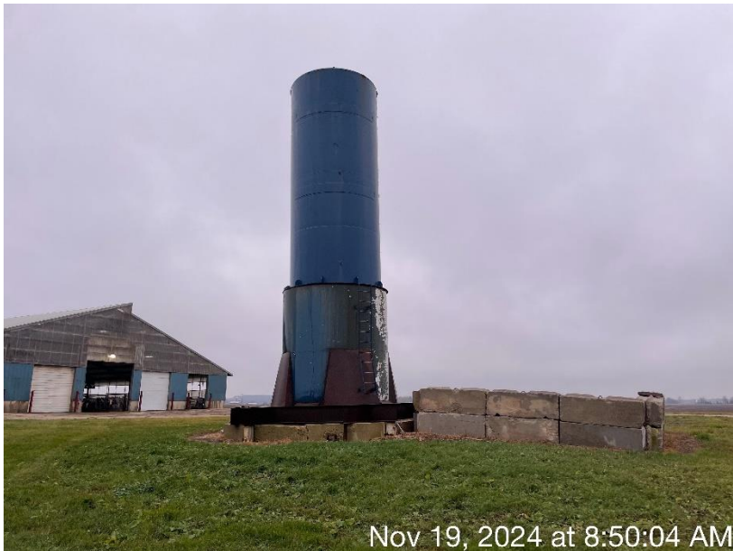
Photo 26. A silo that stores liquid manure for the flush system at the West Site.
