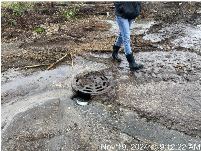
Photo 39. The collection inlet that accepts runoff from the feed storage area and conveys the runoff to WSF 3.
