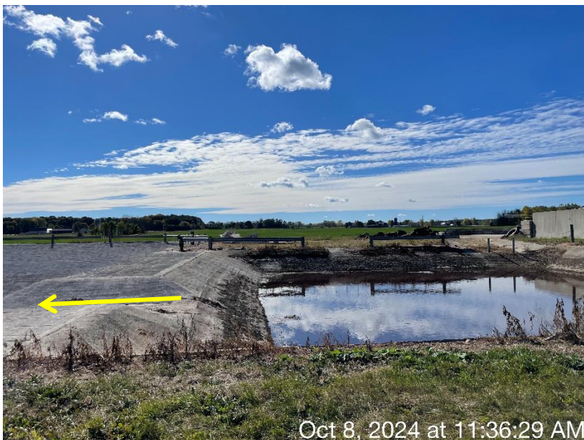
Photo 93. The concrete berm and weir that conveys runoff from the detention basin to WSF 2 at the Longfellow Site. The yellow arrow represents the flow path of process wastewater through the weir.
