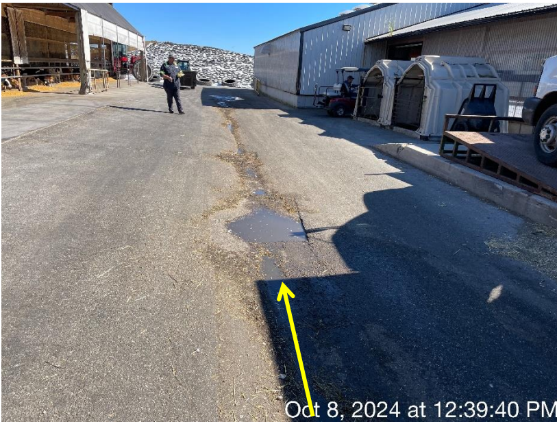
Photo 111. The flow path of stormwater through bedding debris (sawdust) on the driveway between the calf barns.
