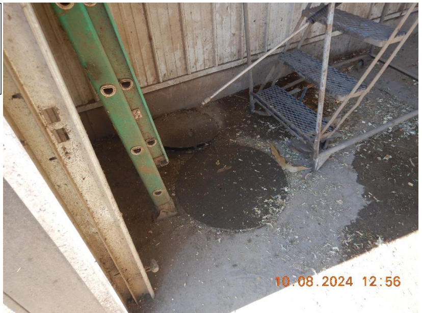
Photo 59. The manhole/pump station associated with the machinery washing center. Wastewater is transferred to WSF 1.
