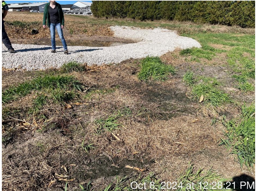
Photo 72. A gravel spreader bar located downslope of the initial gravel spreader bar. Herbicide was used to kill vegetation on the gravel spreader bar.
