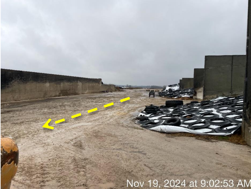
Photo 30. The wall along the west side of the feed storage area at the East Site. The wall was in poor repair, with areas that had cracked or missing concrete.
