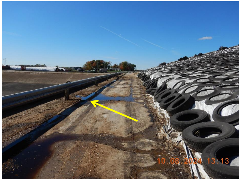
Photo 78. The flow path of runoff within the concrete conveyance channel towards WSF 4.
