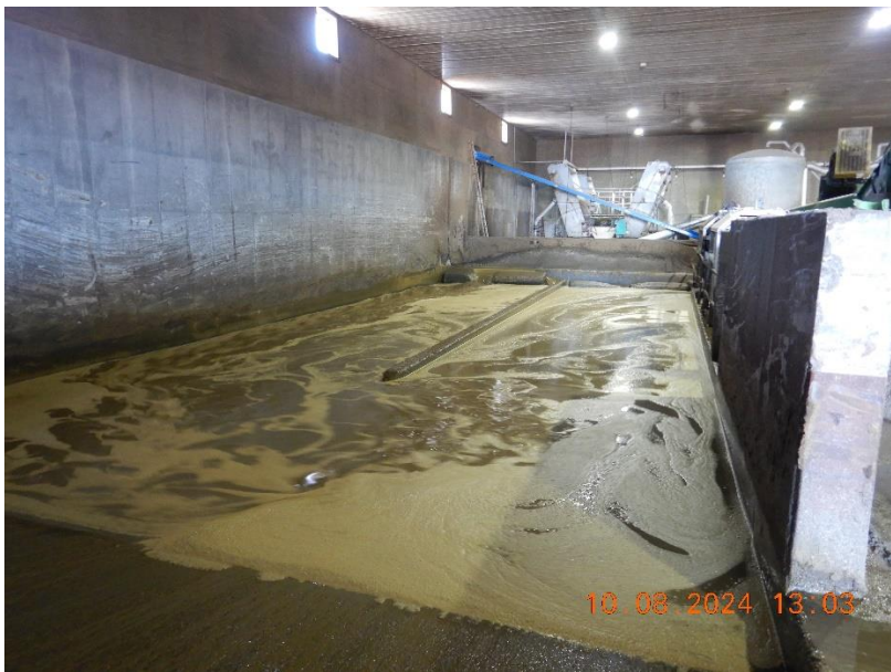
Photo 33. The sand separation system that handles all manure generated in the freestall barns at the Main Site.
