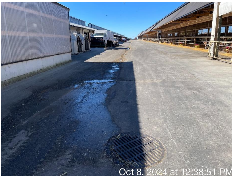
Photo 109. A stormwater outlet located between the calf barns on the south side of the production site at the Main Site. The inlet accepts runoff from the driveway and barn roofs and conveys the runoff to the southern stormwater pond.
