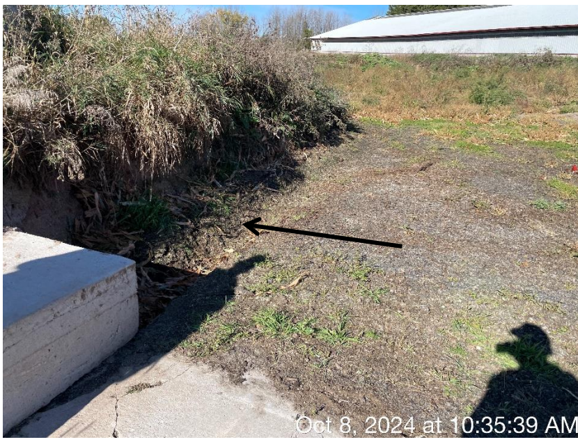
Photo 57. Erosion present along the concrete ramp leading into WSF 1 at the S Farm, identified by the black arrow.
