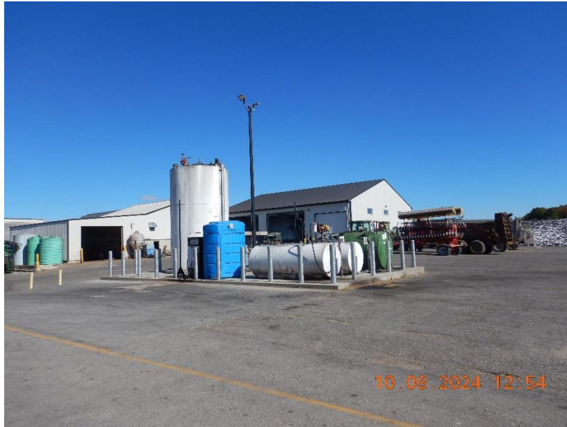
Photo 122. Fuel storage at the Main Site, located near the southern feed storage area.
