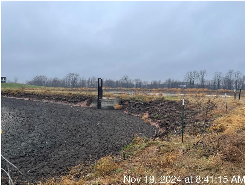
Photo 19. The concrete ladder weir that conveys manure from WSF 4 to WSF 5. The weir is located on the west side of WSF 4.
