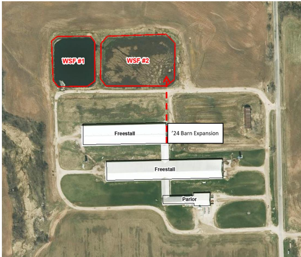
Aerial Map 2. The aerial map above illustrates the west production site at Tonet Dairy. The site consists of two animal barns, a milking parlor, and two liquid waste storage facilities.
