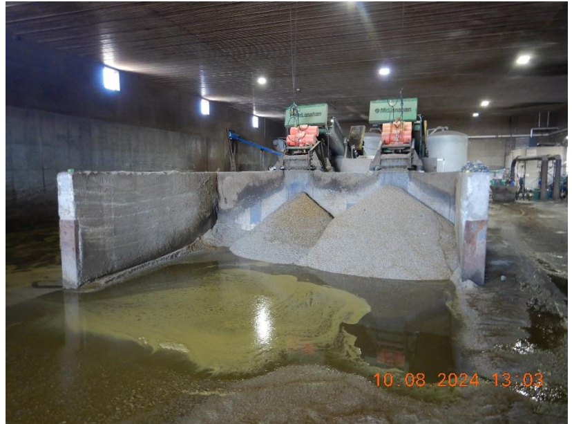
Photo 33. The sand separation system that handles all manure generated in the freestall barns at the Main Site.
