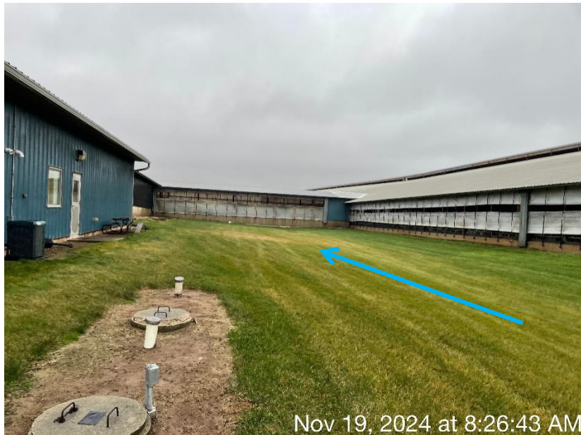
Photo 44. A grassed swale located between the milking parlor and a freestall barn at the West Site. The blue arrow represents the flow path of stormwater to a collection inlet.
