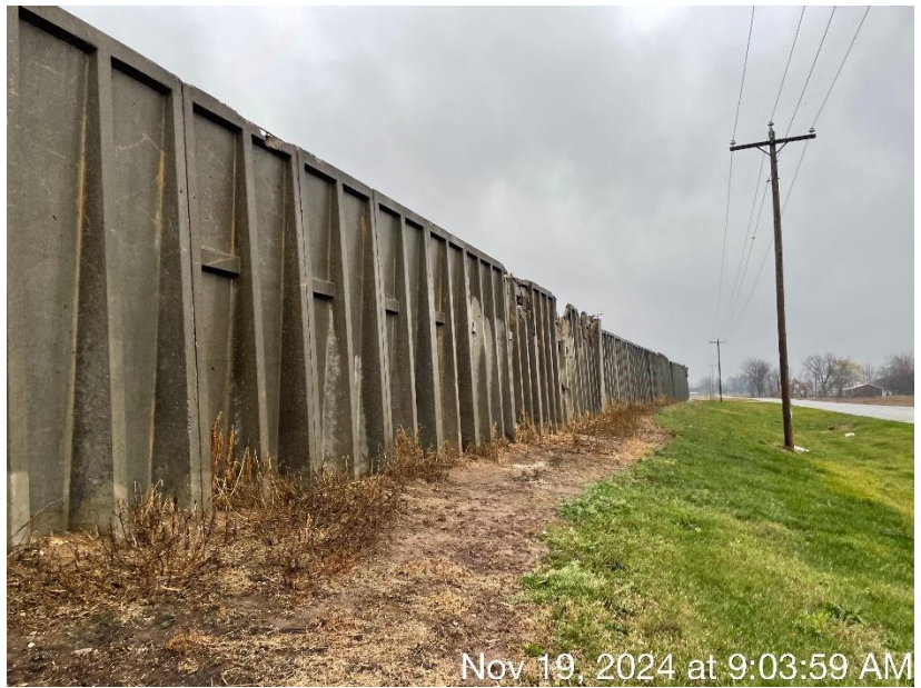
Photo 30. The wall along the west side of the feed storage area at the East Site. The wall was in poor repair, with areas that had cracked or missing concrete.
