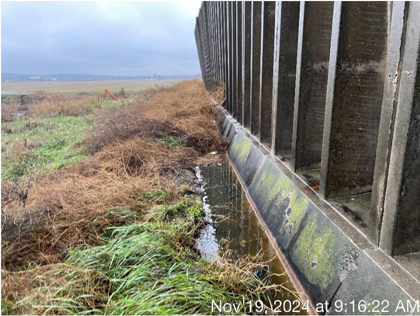
Photo 41. Ponded leachate and process wastewater in a grassed area between the feed storage area and WSF 2. Leachate seeped through the wall along the east side of the feed storage area.
