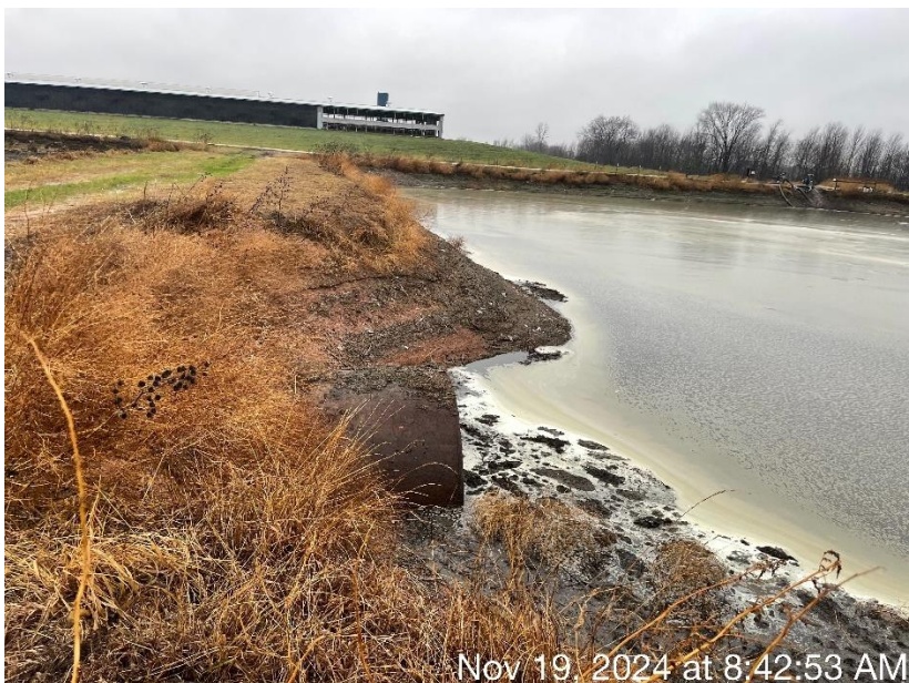
Photo 20. The outfall from the ladder weir into WSF 5. Significant erosion was present around the outfall on the east side of WSF 5.
