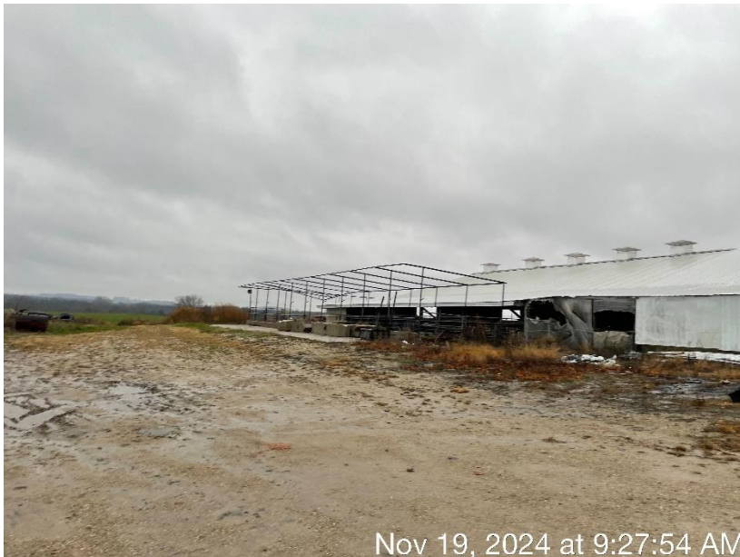
Photo 1. The abandoned feedlot located at the East Site. Animals are no longer housed at the East Site.
