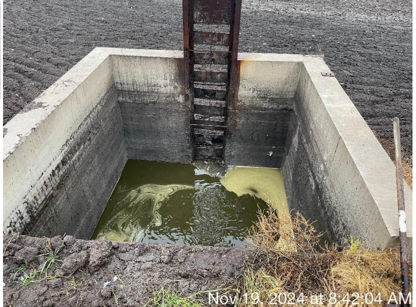
Photo 20. The outfall from the ladder weir into WSF 5. Significant erosion was present around the outfall on the east side of WSF 5.
