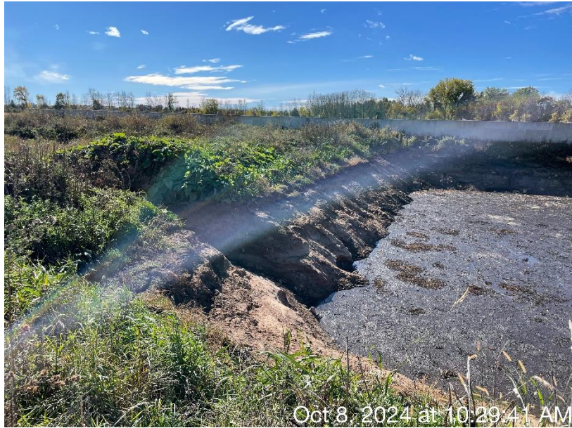
Photo 53. The weir that allows manure to flow from WSF 1 to WSF 2 at the S Farm. Significant erosion was present in the weir.
