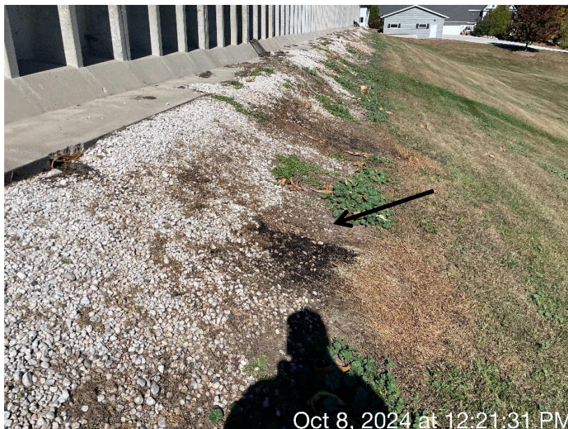
Photo 66. Evidence of seepage of leachate from the perimeter tile line around the southern feed storage area.
