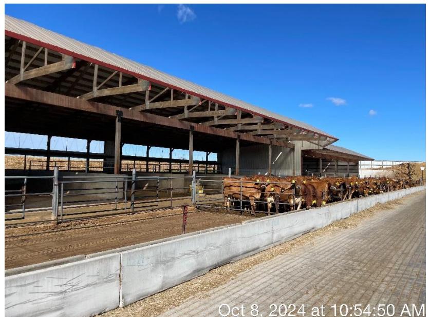
Photo 2. The western outdoor concrete feed lot at the K Farm. Runoff flows north where it then flows into the northwest corner of the liquid waste storage facility at the K Farm.
