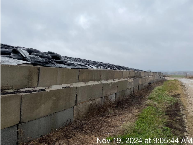
Photo 33. An area where leachate and process wastewater seeps through the southern wall along the feed storage area at the East Site.
