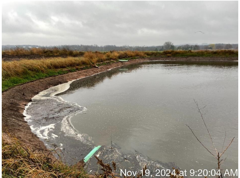
Photo 11. WSF 3, located at the East Site. WSF 3 is located south of WSF 2 and accepts runoff from the feed storage area. This photo was taken facing west.
