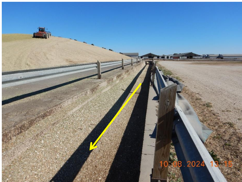
Photo 78. The flow path of runoff within the concrete conveyance channel towards WSF 4.
