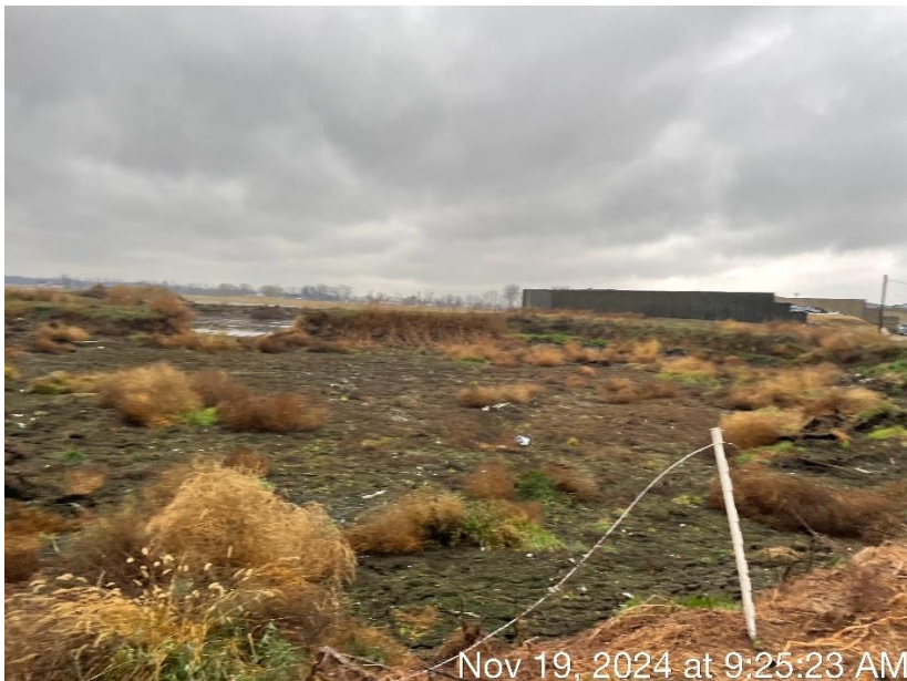
Photo 2. WSF 1, located at the East Site. WSF 1 is located on the east side of the production area, north of WSF 2. Fencing around the storage was in poor repair.
