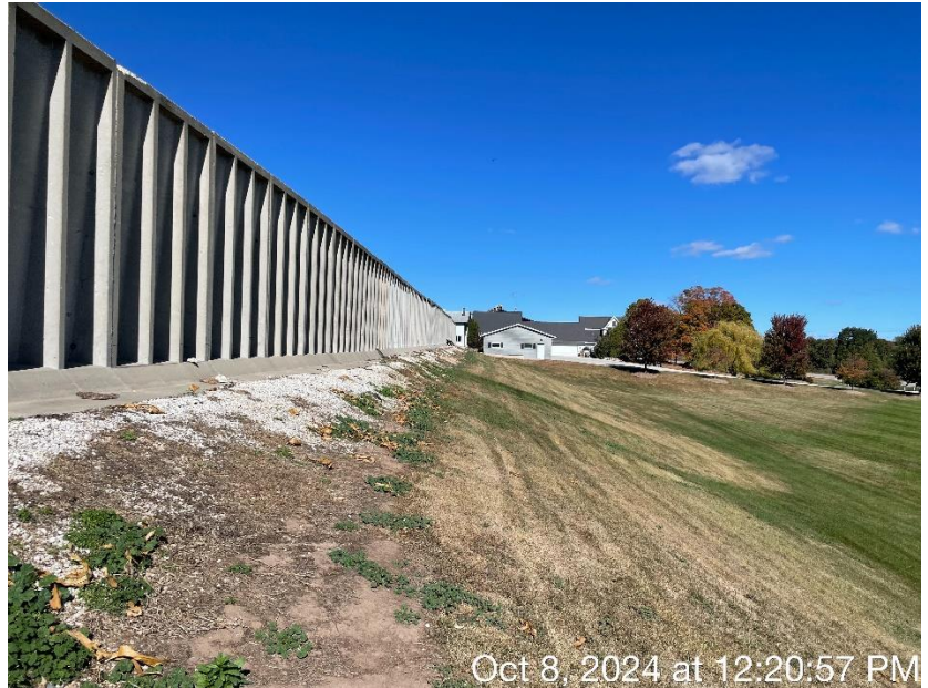
Photo 66. Evidence of seepage of leachate from the perimeter tile line around the southern feed storage area.
