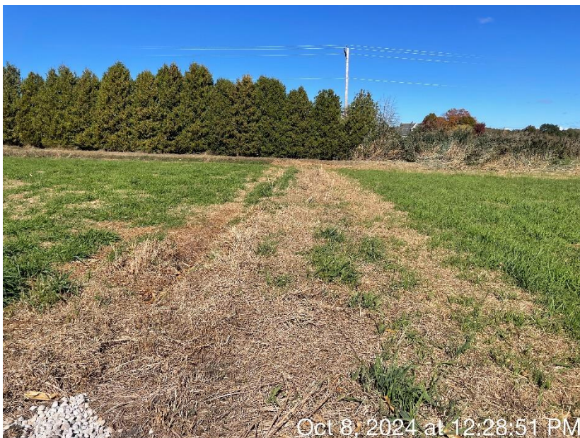
Photo 72. A gravel spreader bar located downslope of the initial gravel spreader bar. Herbicide was used to kill vegetation on the gravel spreader bar.
