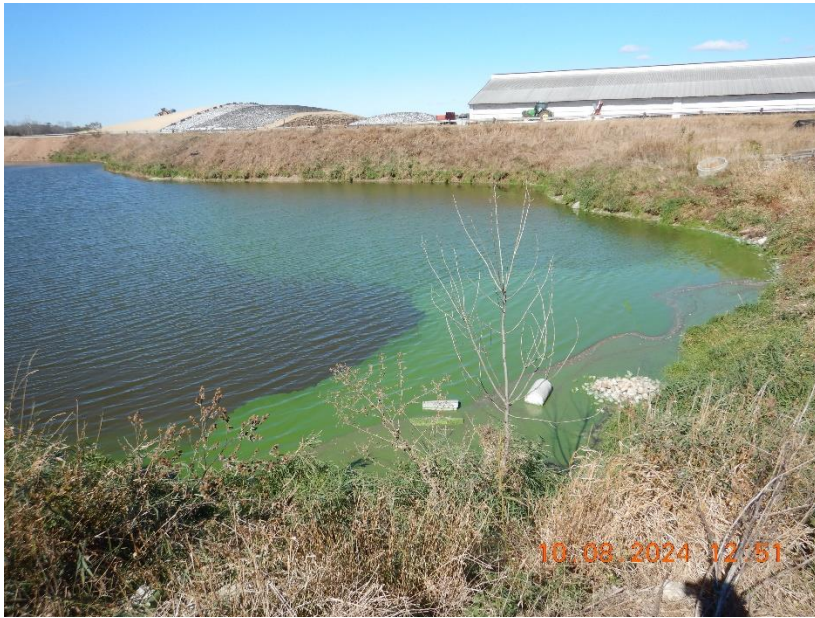
Photo 114. The outlet associated with the stormwater inlet pictured in Photo 108. The outlet discharges stormwater in the southeast corner of the large stormwater pond.
