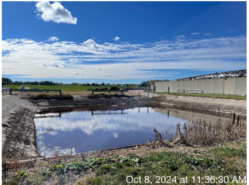
Photo 93. The concrete berm and weir that conveys runoff from the detention basin to WSF 2 at the Longfellow Site. The yellow arrow represents the flow path of process wastewater through the weir.
