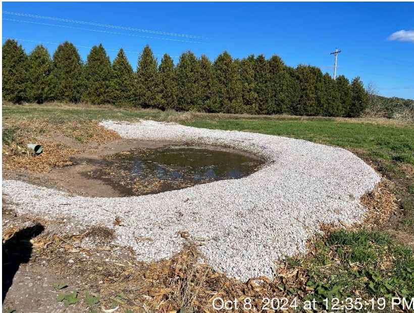
Photo 71. Burnout present adjacent to the gravel spreader bar.
