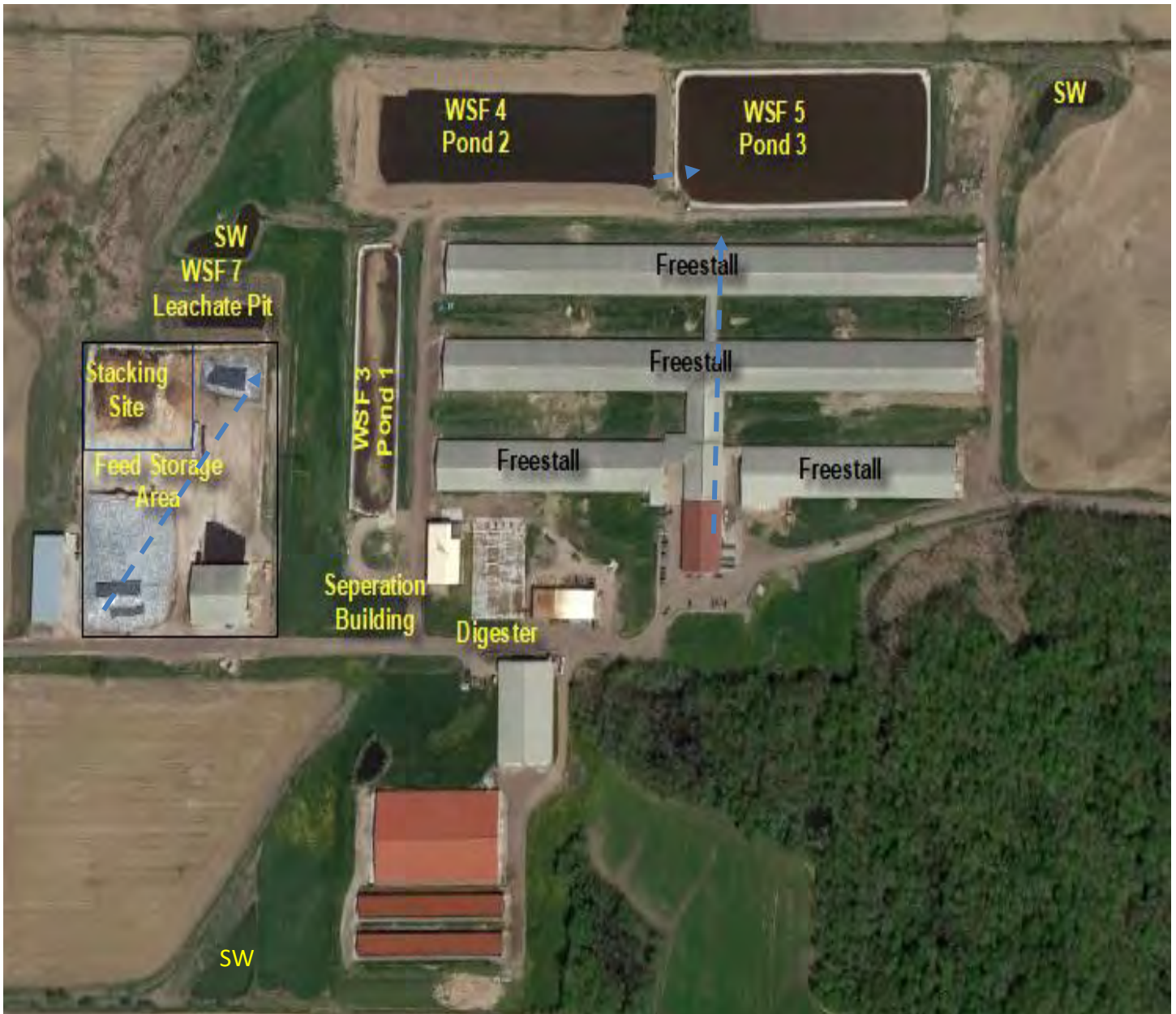
Figure 2. Aerial overview of Holsum Dairy: Holsum Elm Site. Blue arrows indicate flow paths for manure or leachate.
