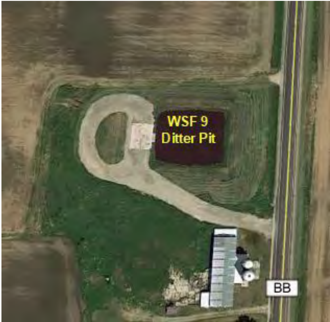
Figure 4. Aerial overview of Holsum Dairy: Ditter Farm Satellite Pit.
