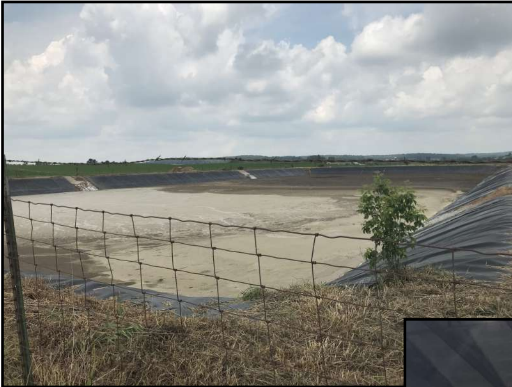
Photo 1 (left): Looking south east across WSF 1. A safety fence was observed around the entire perimeter of the storage.
