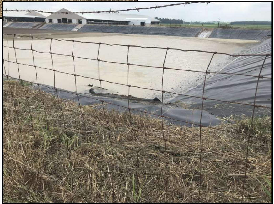
Photo 4 (right): Looking at the south west corner of WSF 1. Some splitting was observed at the seam where the HDPE liner overlaps in this corner of the storage.
