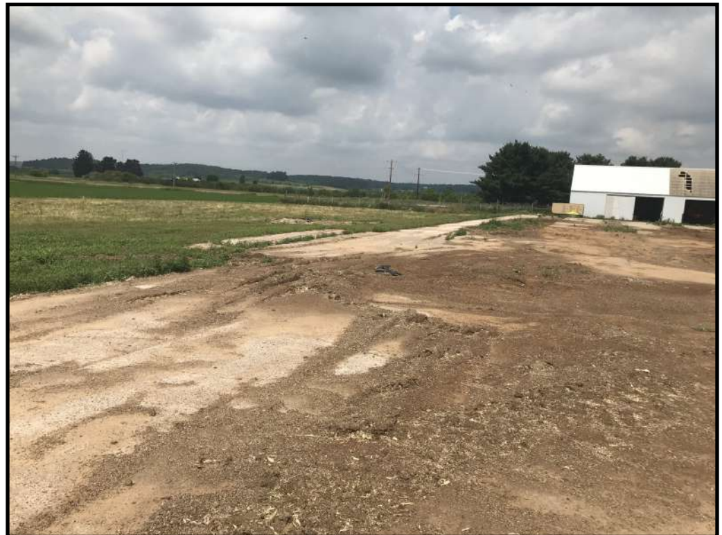
Photo 6 (right): Looking north west across the area where the demolished barns, outdoor lots, and solid manure stacking area were once located.
