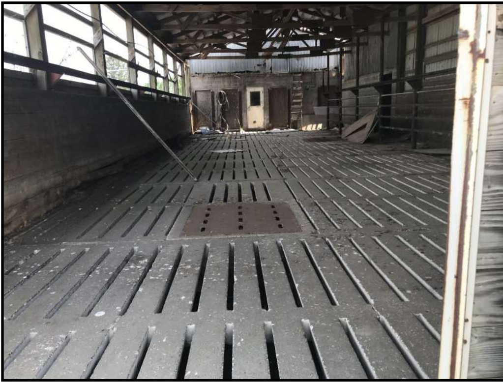
Photo 5 (left): Looking inside the barn with an underbarn storage facility. Use of the barn has been discontinued and remaining manure has been removed from the underbarn storage. Full abandonment of the underbarn storage facility is still needed.
