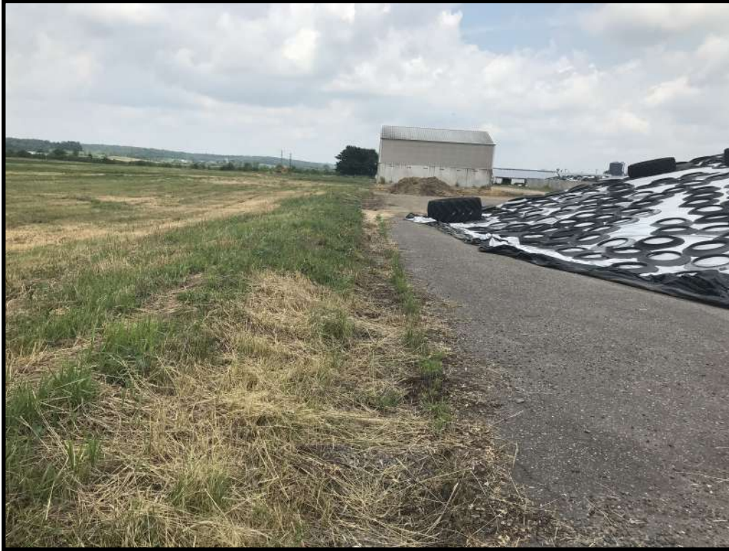
Photo 7 (left): Looking north along the western edge of the feed storage area. The earthen berm that was installed as part of the interim runoff controls can be seen along this edge of the feed storage area.
