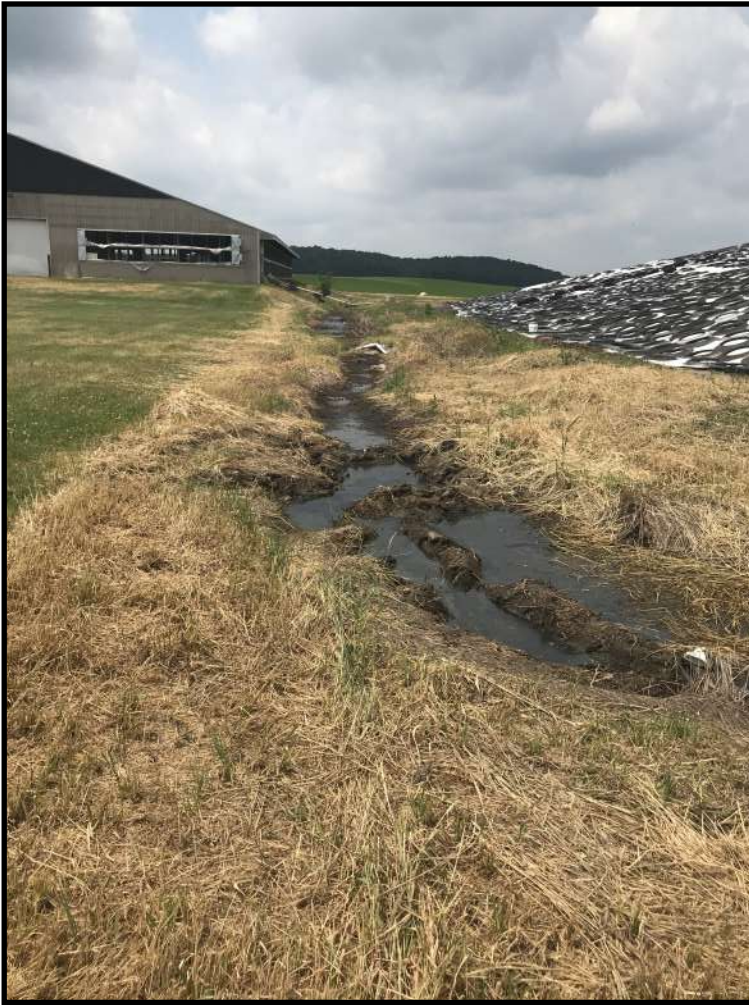
Photo 11 (top left): Looking west where the channel pictured in photo 10 proceeds west along the southern edge of the feed pad toward a culvert that runs under the adjacent driveway. Dark cloudy water can be seen within the channel along the entire length of the pad.
