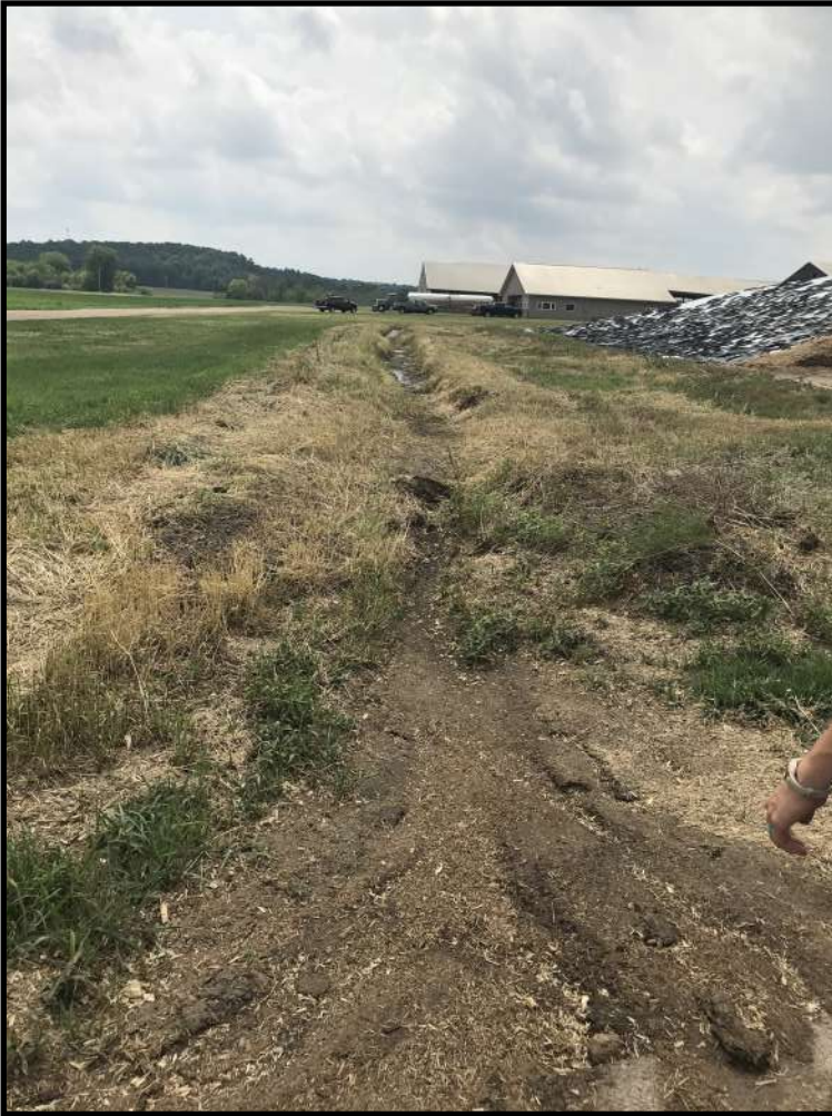
Photo 9 (left): Looking south at the beginning of the channel that runs south along the eastern edge of the feed pad. Dried debris containing waste feed can be seen accumulating at the beginning of the channel.
