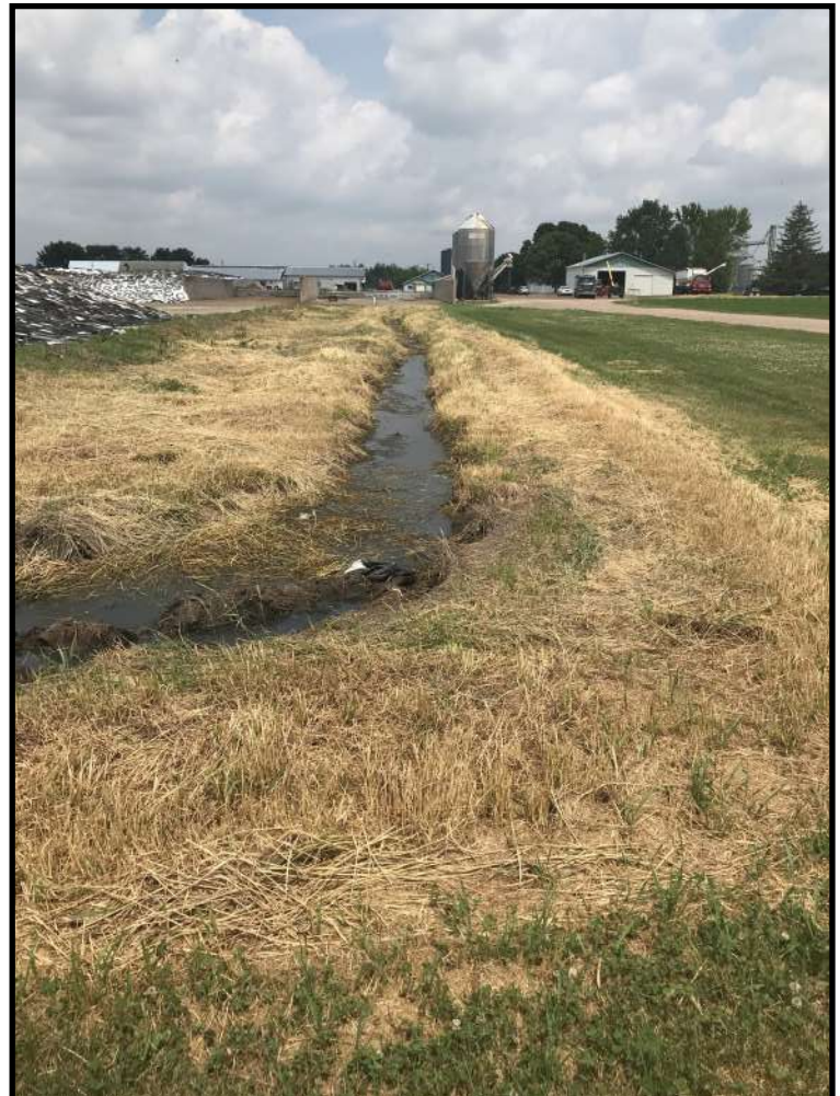
Photo 10 (right): Looking north at the point where the channel pictured in photo 9 diverts west along the southern edge of the feed pad. Dark cloudy water can be seen filling the channel.
