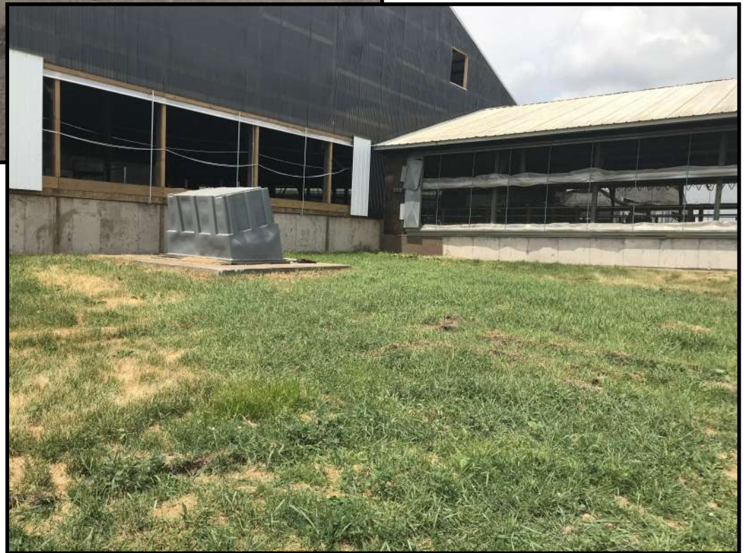
Photo 15 (right): Looking at the grassy area surrounding the pump tank for the freestall barns. The pump tank had issues with overflowing in the past which have since been resolved. No evidence of manure overflow was observed in the area surrounding the pump tank.
