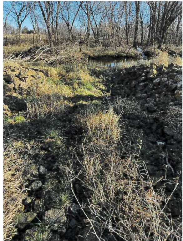
Seventh Day Waterway rock chute 12/9/24
