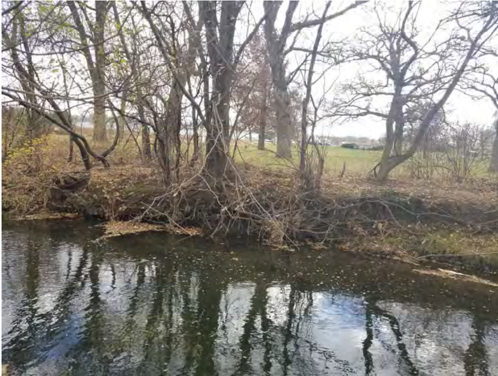
SEGMENT 9- Exposed roots, bare banks in some location, slumping soil in other locations.
