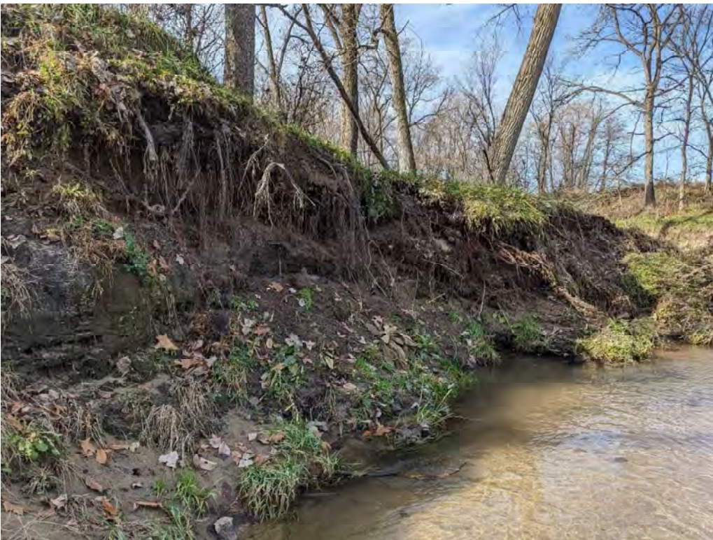
Figure 32: Bank 8 – South Side Looking Down Stream
