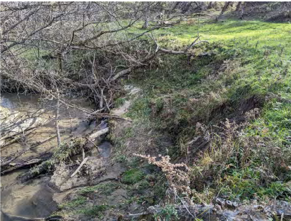
Figure 25: Bank 6 – South Side On Top of Bank Looking Up Stream
