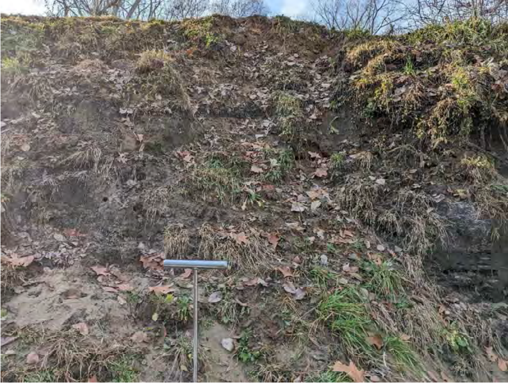
Figure 31: Bank 8 – Straight On View
