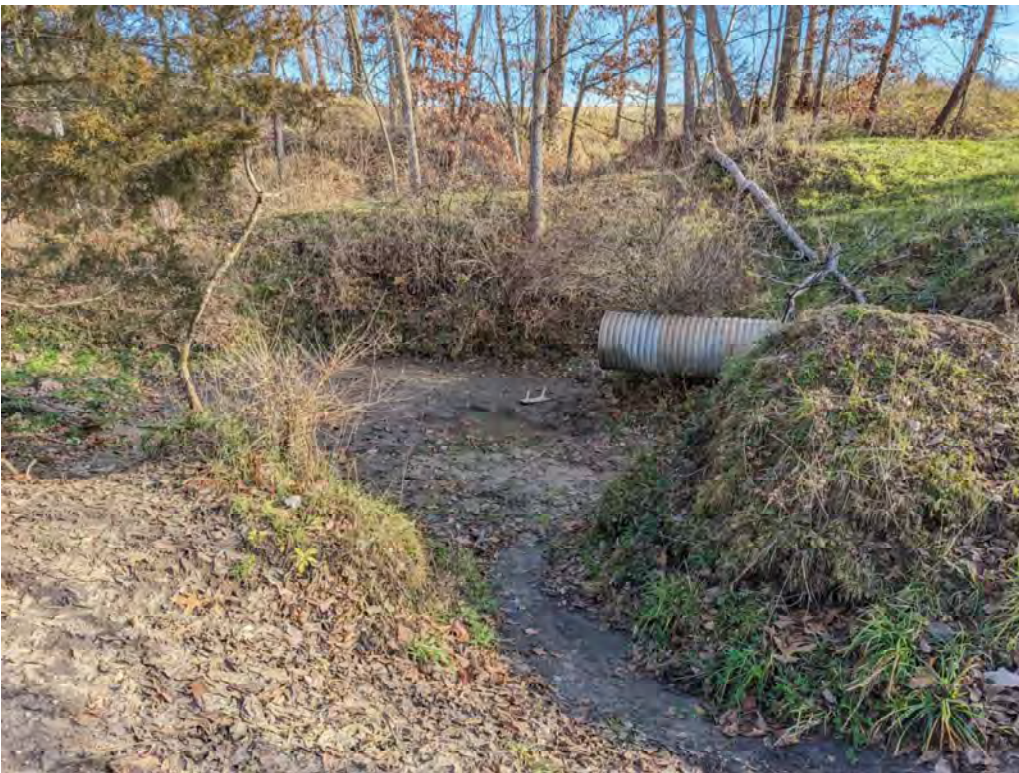
Figure 6: Crossing/Grade Stabilization of existing pipe outlet
