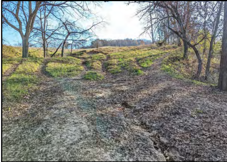
Figure 7: Upstream Spring Area Erosion.
