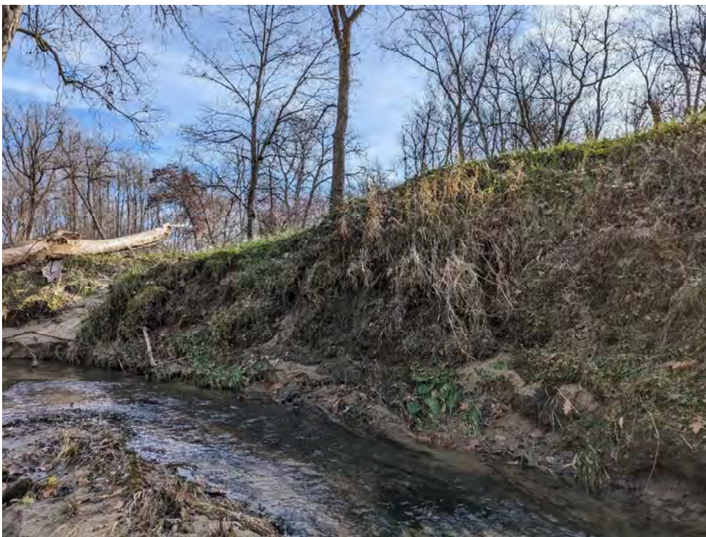
Figure 30: Bank 7 – South Side Looking Up Stream
