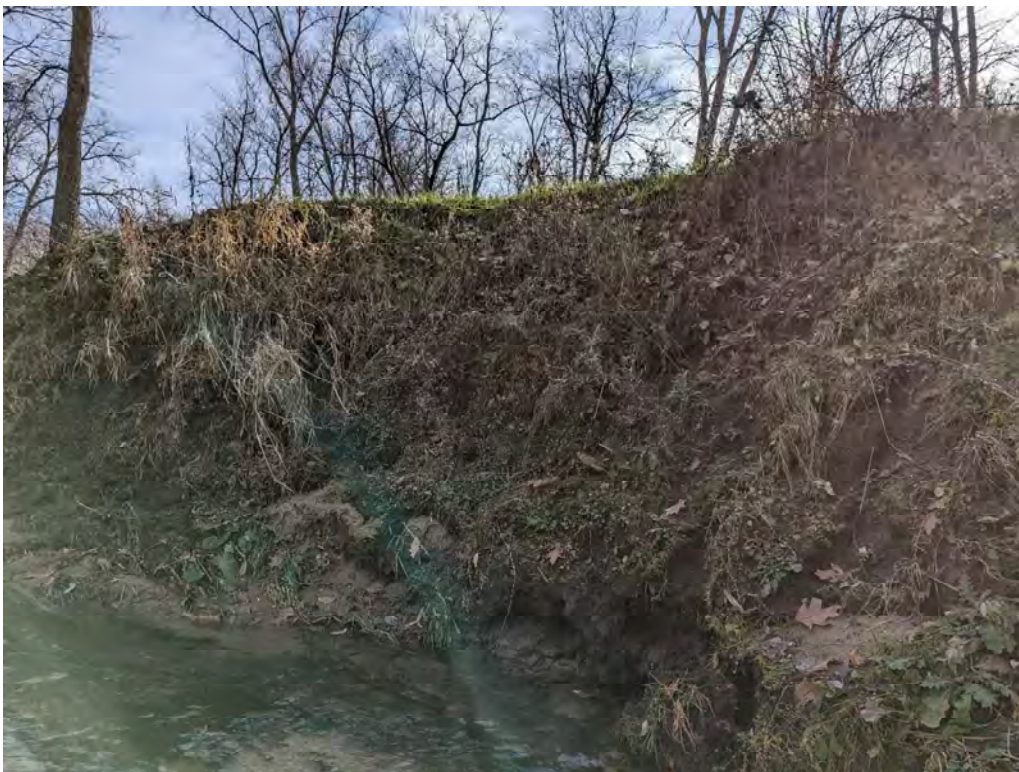
Figure 29: Bank 7 - South Side Looking Up Stream
