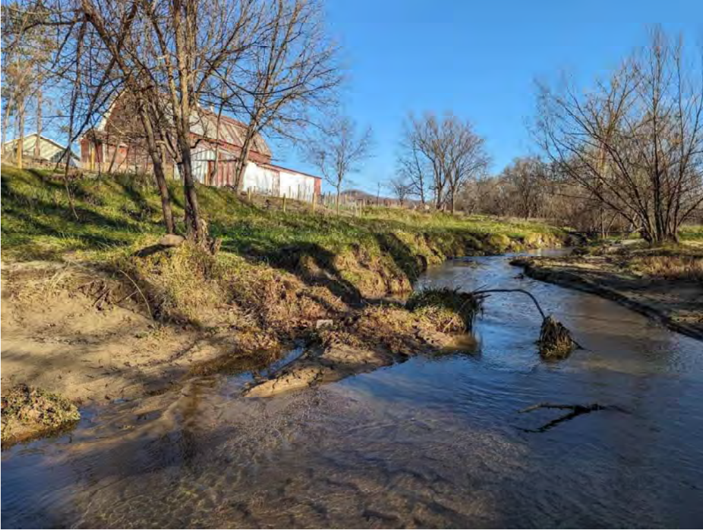
Figure 12: Section 3/Bank 3 - North Side Looking Up Stream
