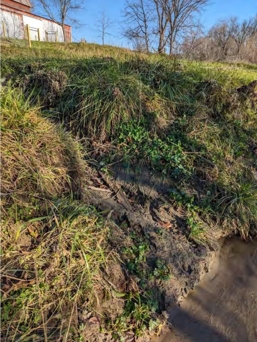
Figure 17: Section 3/Bank 3 - North Side Looking Up Stream
