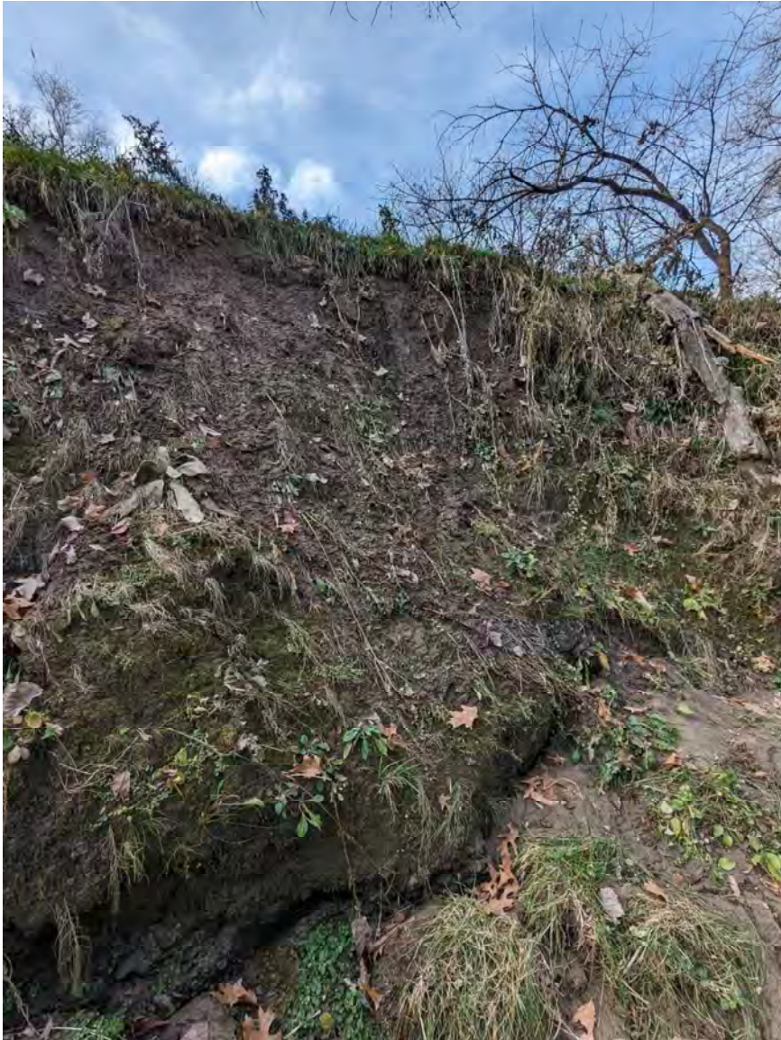
Figure 28: Bank 7 - South Side Looking Down Stream
