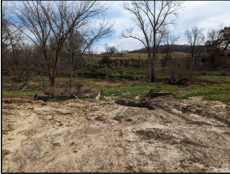
Figure 4: Dutch Creek Stream Crossing Erosion.
