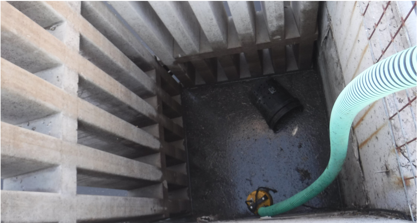
Photo #: 5765 Photo Description: North feed storage area northeast runoff collection sump utilizing portable pump and transfer line Date/Time of Photo: 8-26-21 / AM Photo Location: Calf Source Photo By: Uvaas
