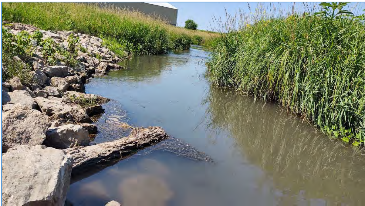
Figure 7: Photograph of an escape log (aquatic habitat) installed along bank W34. A total of six (6) escape logs and two (2) root wad log revetments were installed at Site A.
