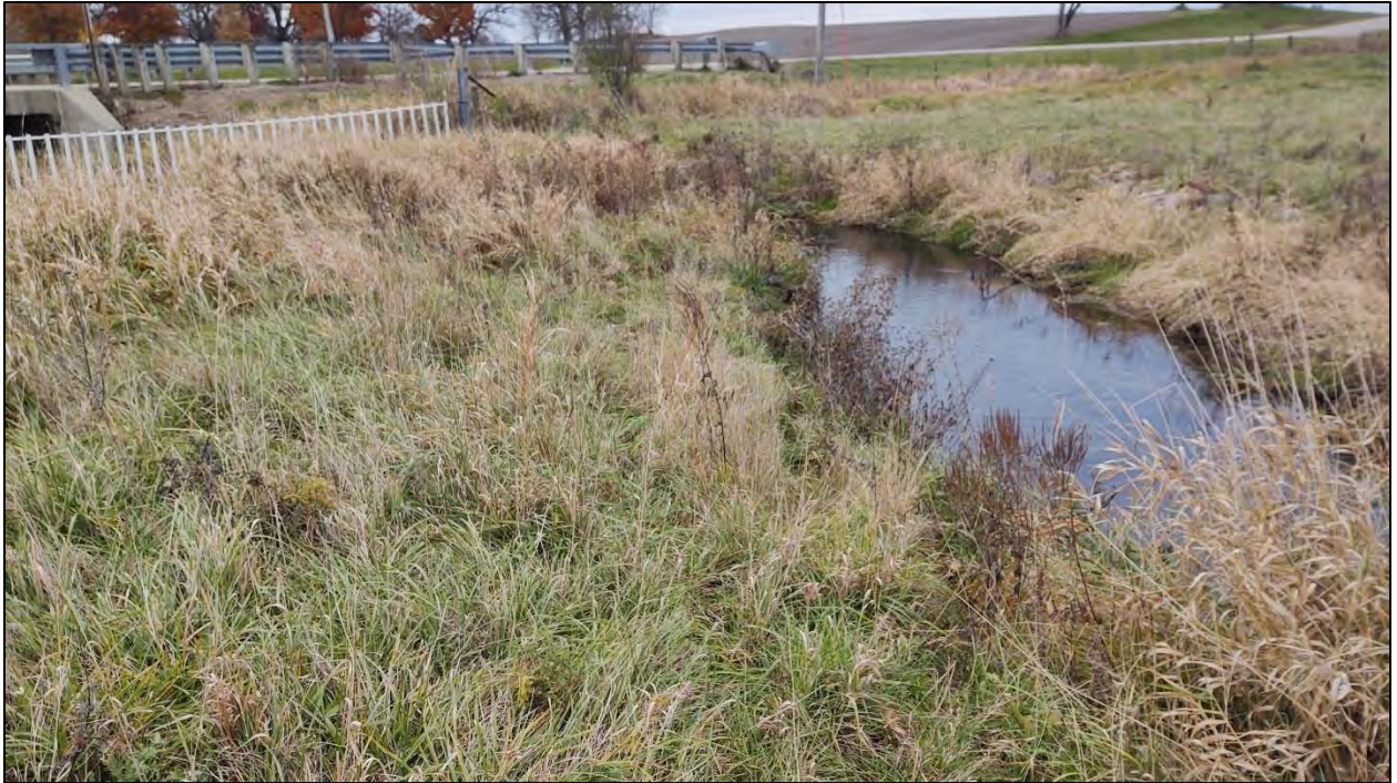
Figure 13: Photograph of Streambank W36 on November 15, 2021
