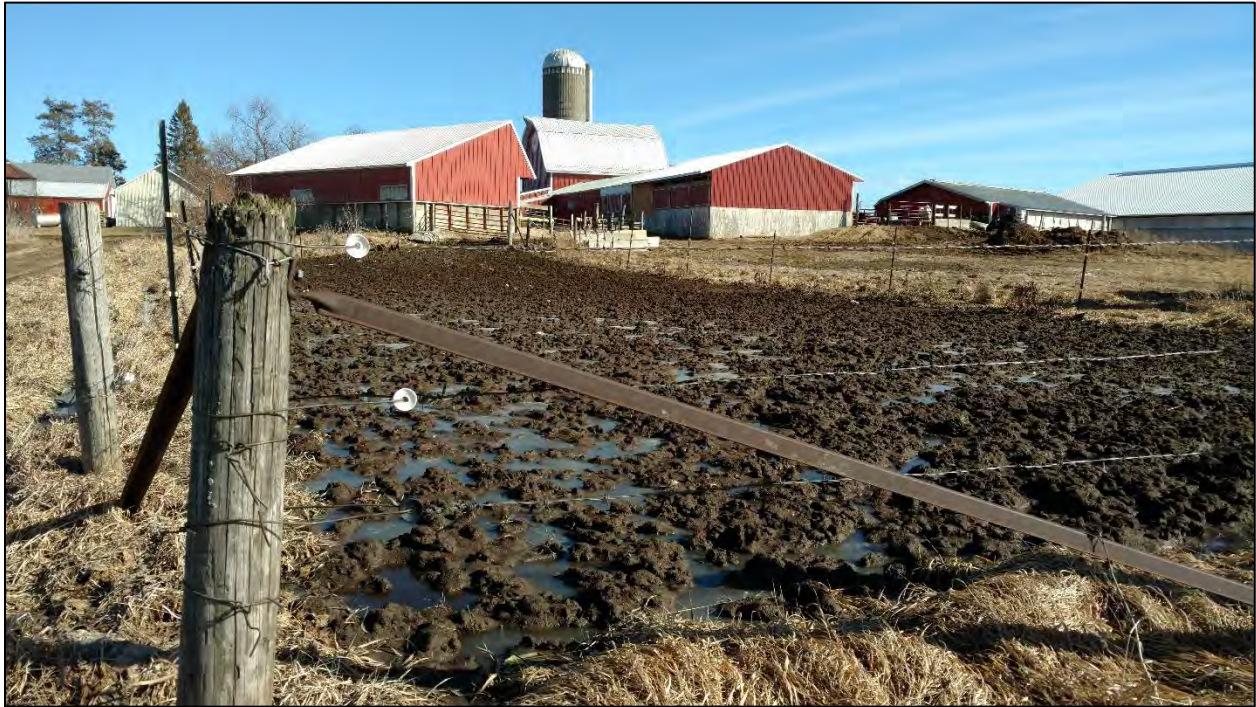
Figure 3: Photograph of Lot #1 (pre-construction)
