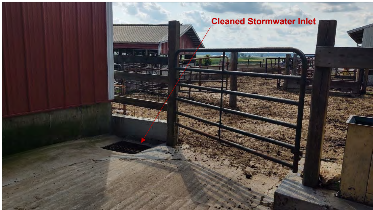
Figure 31: Photograph of cleaned stormwater inlet Lot #3 taken on September 8, 2022
