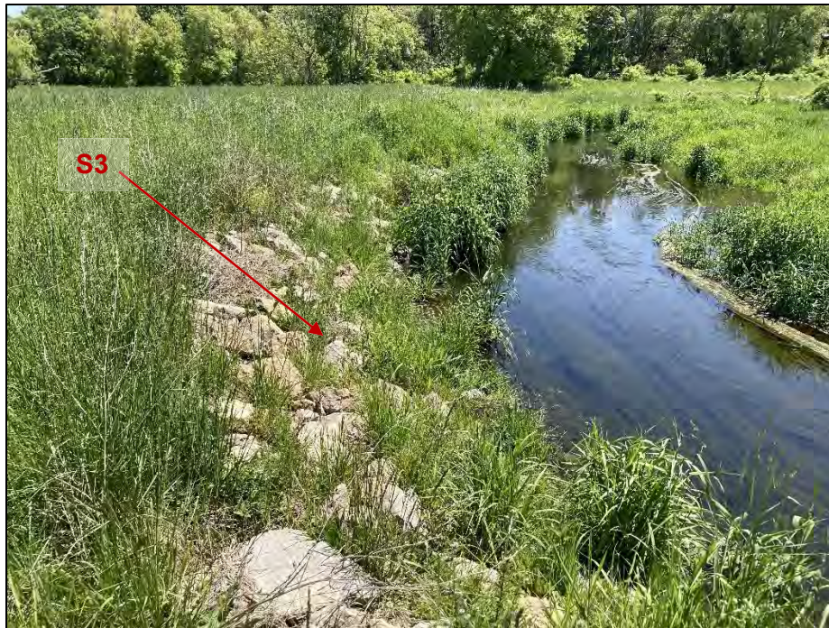
Figure 18: Photograph of Streambank S3 on May 26, 2023
