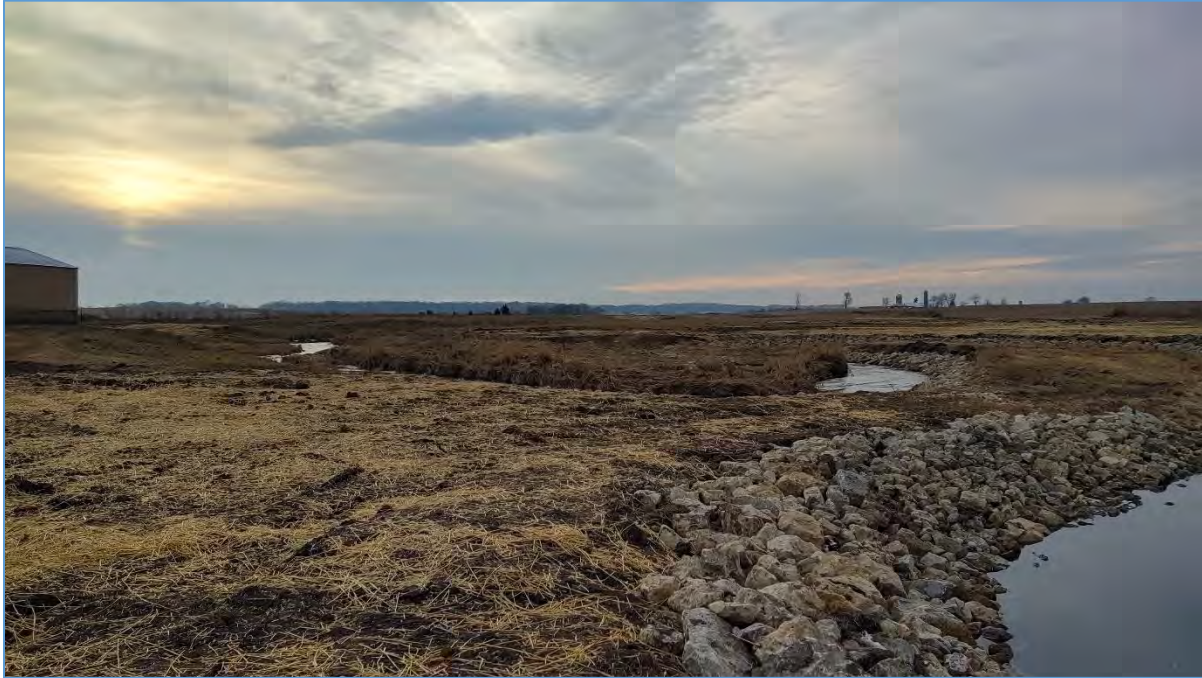
Figure 4: Photograph from December 2019 of banks W34, W35, and W37. All three sites were stabilized with riprap.
