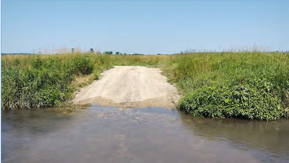
Figure 8: Photograph of a stream crossing (ford) installed near bank W25. A total of four (4) rock crossings were installed at Site A to allow safe crossing of the stream by agricultural equipment and livestock.
