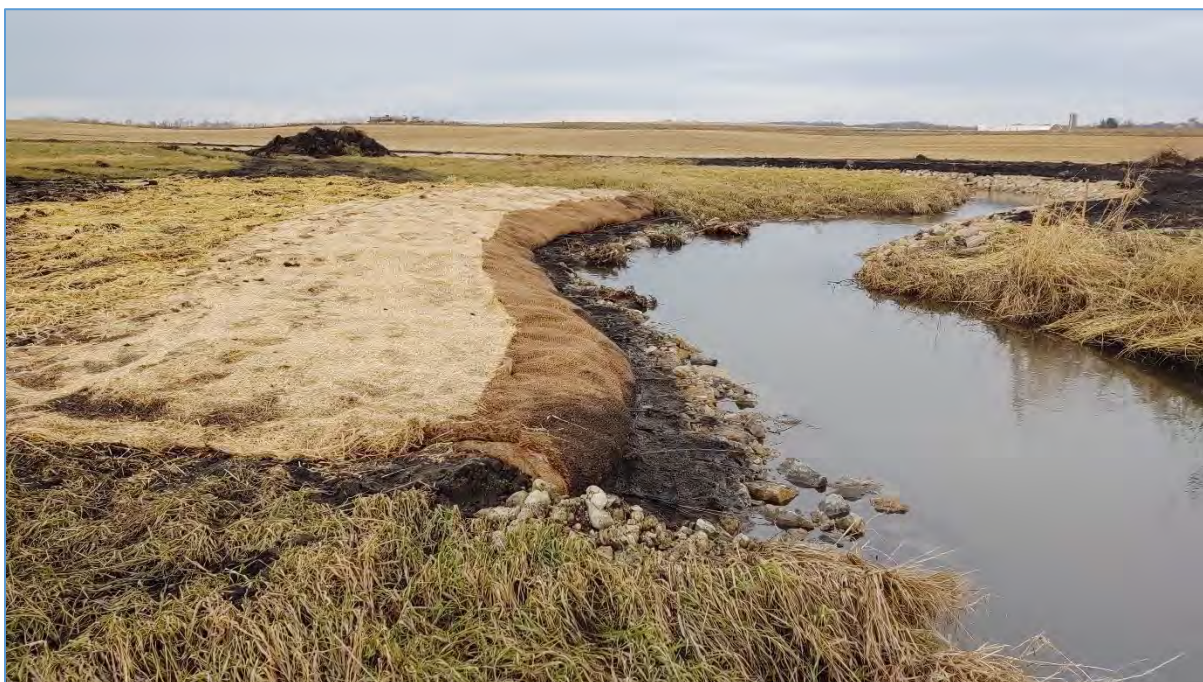
Figure 3: Photograph from December 2019 of bank W32. This site was also stabilized using riprap, vegetated reinforced soil (VRSS) lifts, willow live cuttings, and root wads.
