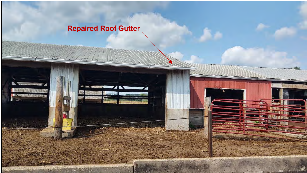
Figure 29: Photograph of repaired roof gutter for Lot #3 taken on September 8, 2022
