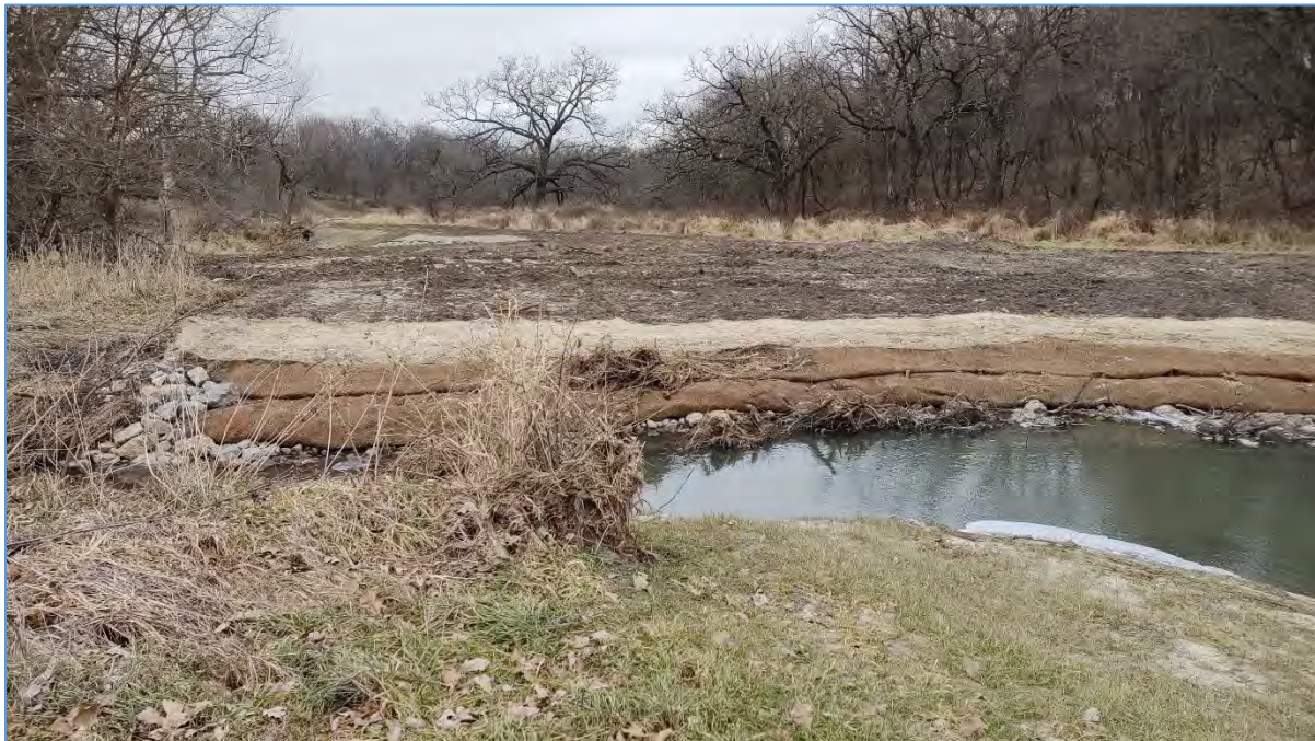
Figure 6: Photograph from December 2019 of bank S14. This site was stabilized using riprap, vegetated reinforced soil (VRSS) lifts, willow live cuttings, and root wads. Top of bank has since been seeded and mulched.
