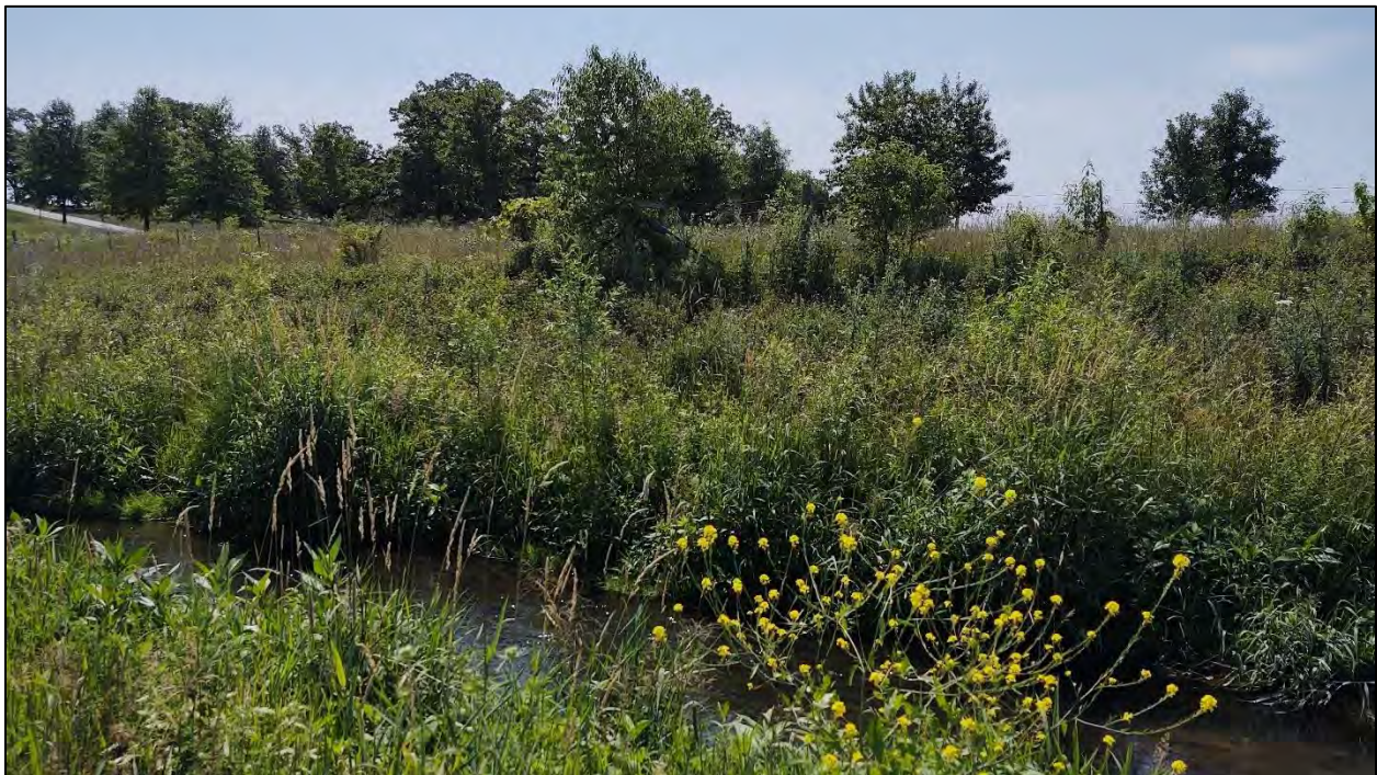
Figure 17: Photograph of Streambank S1 on July 2, 2021
