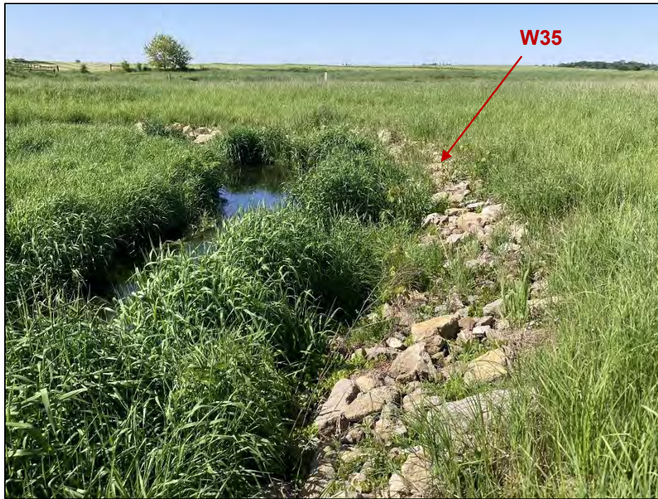
Figure 8: Photograph of Streambank W35 on May 26, 2023
