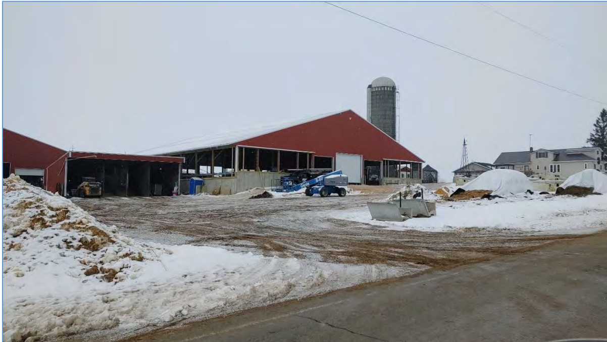
Figure 10: Photograph of the newly constructed building (roof cover) for Lot #4 Landowner C.
