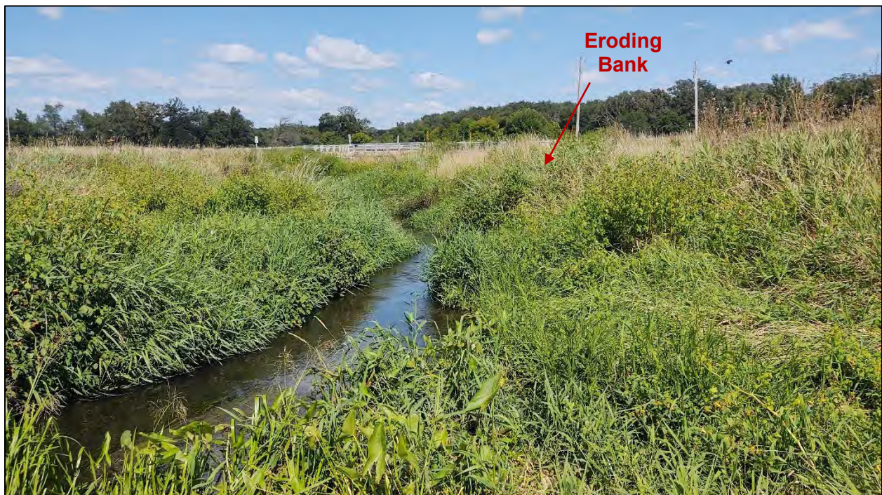
Figure 11: Photograph of new eroding streambank between banks W33 and W34 taken on August 23, 2022
