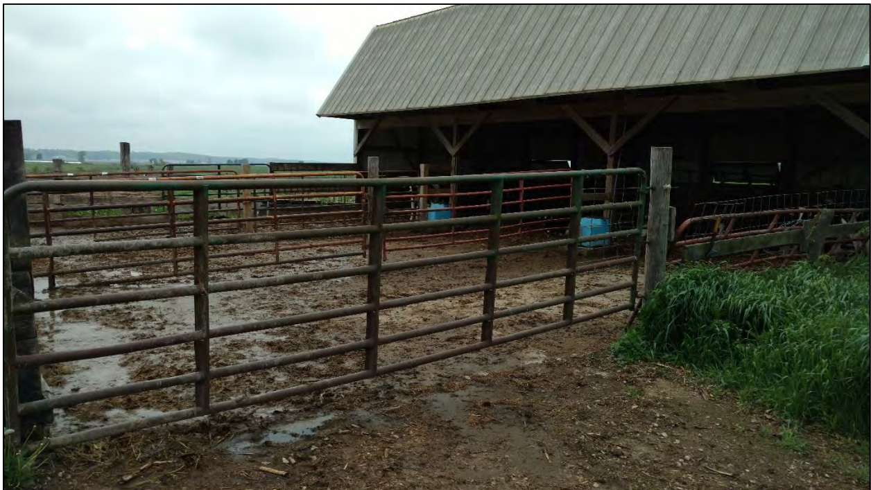
Figure 4: Photograph of Lot #2 (pre-construction)
