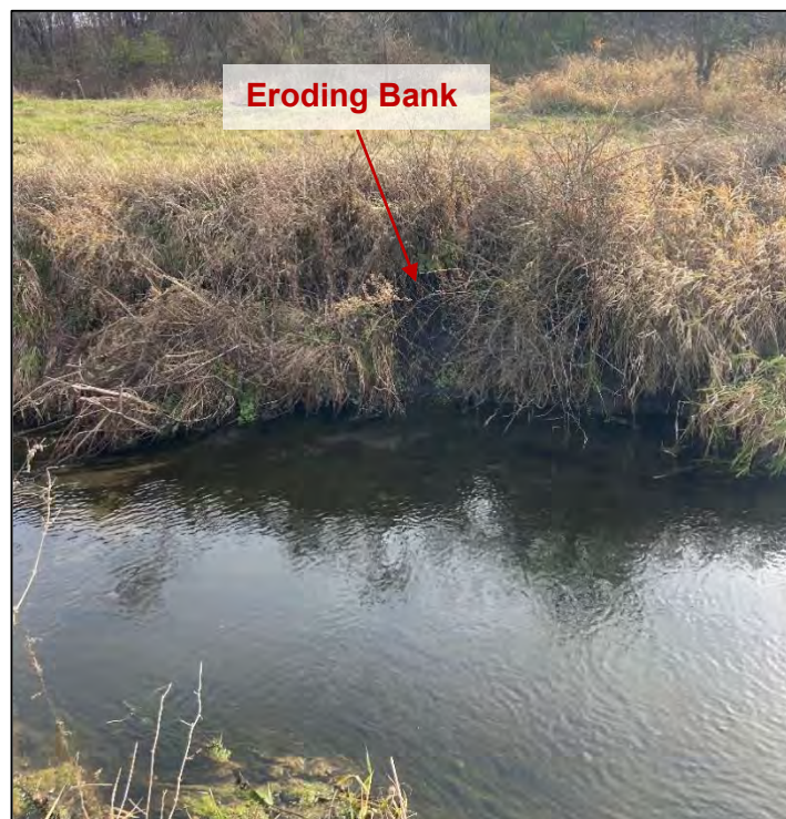
Figure 4-14: Photograph of eroding streambank between banks S19 and S20 (RBFD) taken on November 20, 2023
