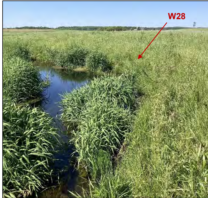
Figure 6: Photograph of Streambank W28 on May 26, 2023
