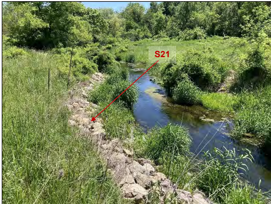
Figure 22: Photograph of Streambank S21 on May 26, 2023
