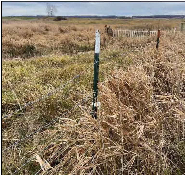
Figure 4-8: Photograph of leaning fence posts on west side of property taken on November 20, 2023
