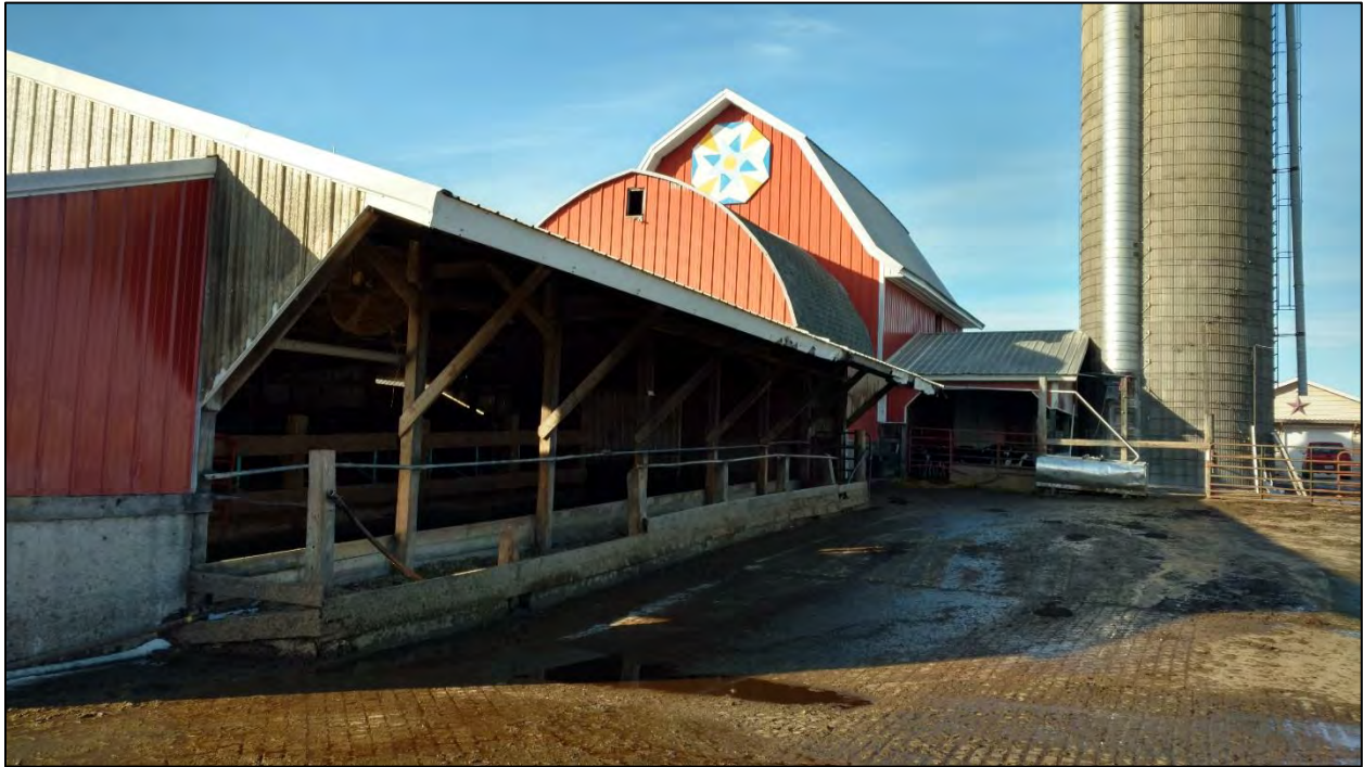
Figure 7: Photograph of Lot #4 (pre-construction)
