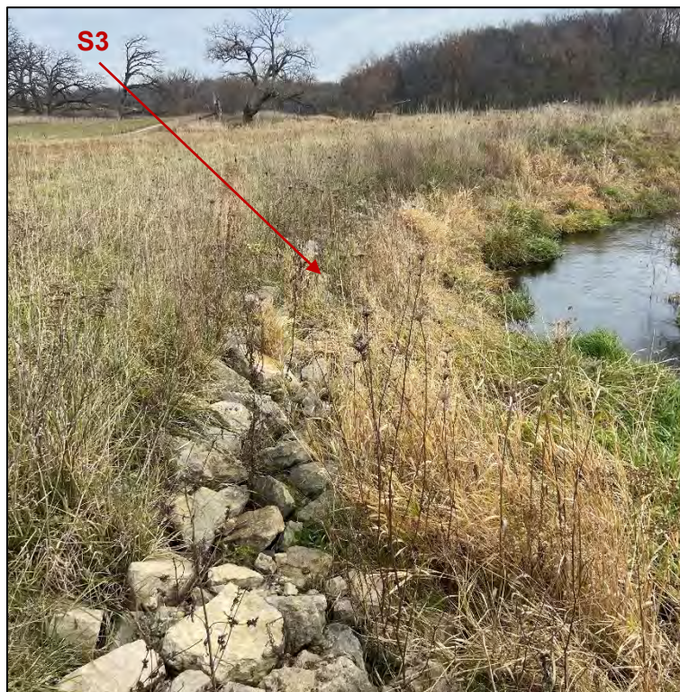
Figure 19: Photograph of Streambank S3 on November 20, 2023
