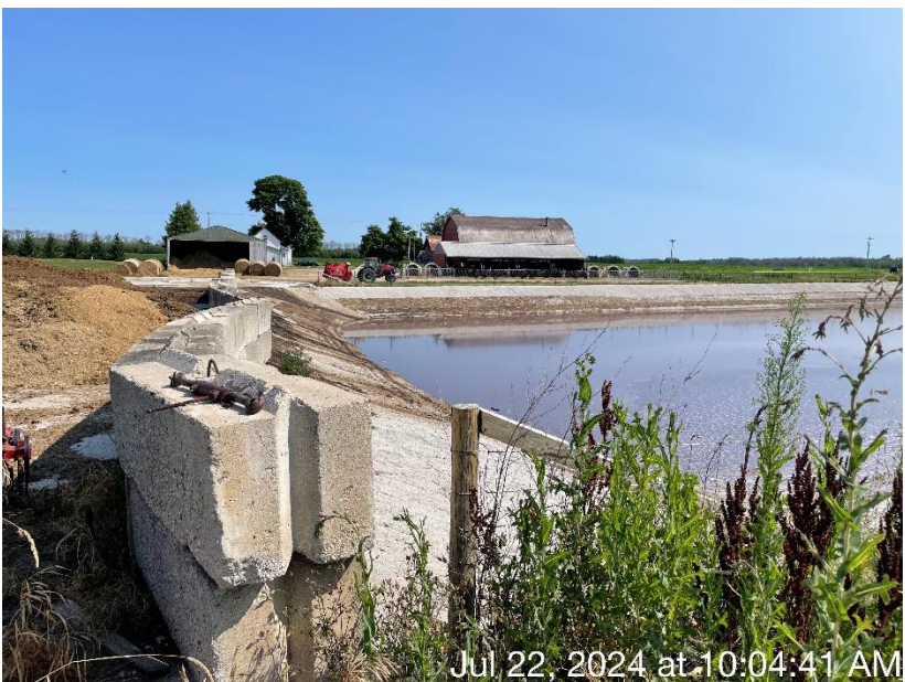
Photo 19. WSF 2 at Augustian Farms LLC located on the northeast portion of the production site. WSF 2 accepts runoff from the feed storage area and manure stacking area. This photo was taken facing north.
