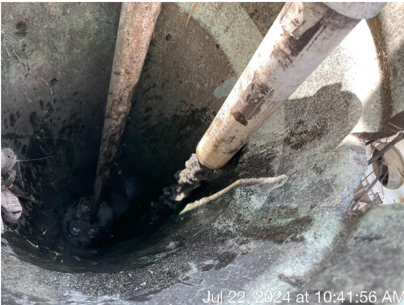
Photo 29. The sump located adjacent to the milking parlor. The sump collects clean water from a gravel layer and pumps the water to a tile line located west of the milking parlor.
