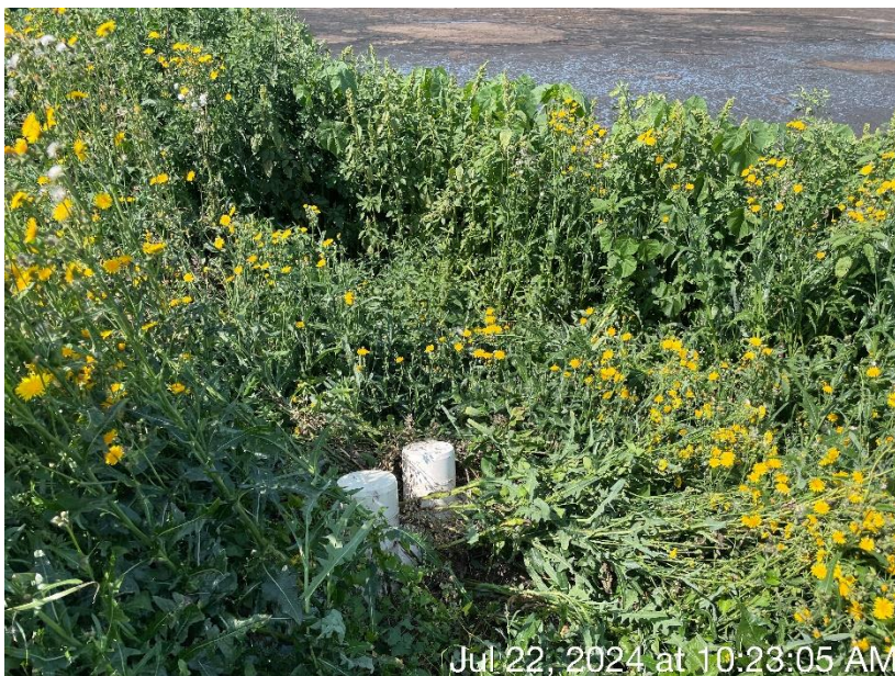
Photo 13. Permanent markers present on the east berm of WSF 1. Salscheider recommended killing off the vegetation so that the markers are more visible.
