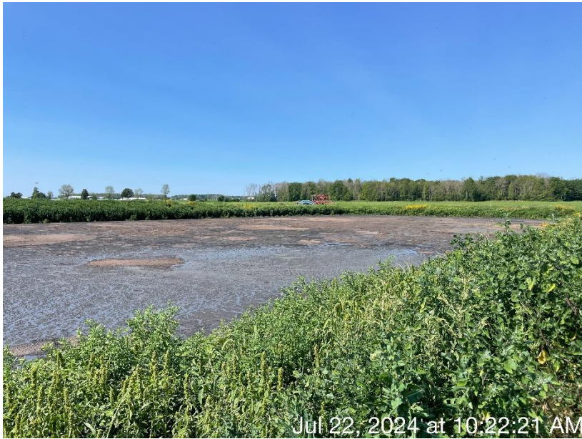
Photo 12. WSF 1 at Augustian Farms LLC, located on the south side of the production site. WSF 1 accepts manure and process wastewater from the freestall barns and milking parlor. This photo was taken facing west.
