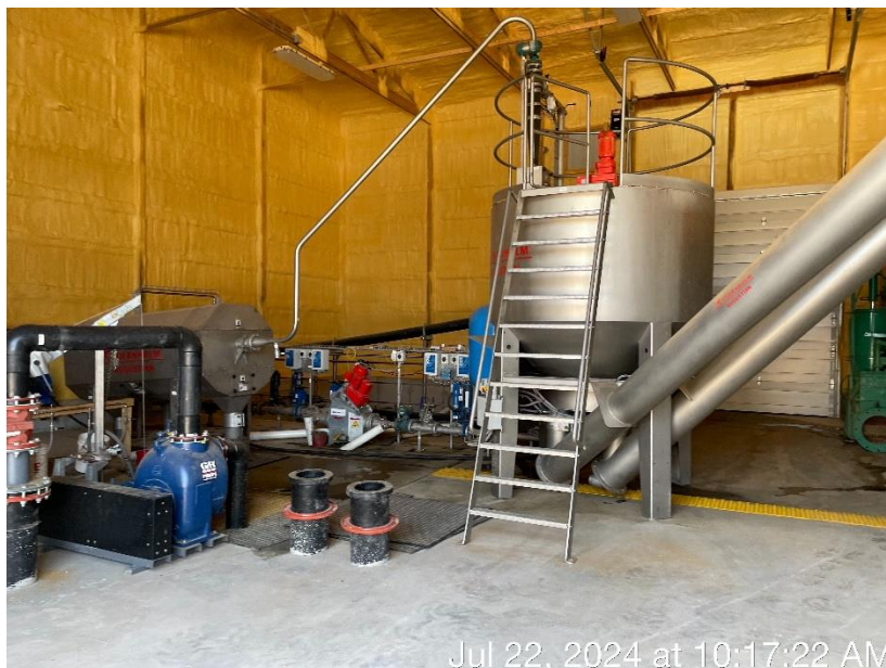
Photo 25. The sand separation equipment that removes sand bedding material from liquid manure prior to transferring manure to existing storage.
