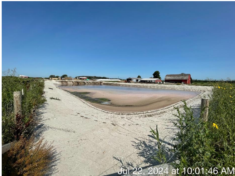
Photo 19. WSF 2 at Augustian Farms LLC located on the northeast portion of the production site. WSF 2 accepts runoff from the feed storage area and manure stacking area. This photo was taken facing north.
