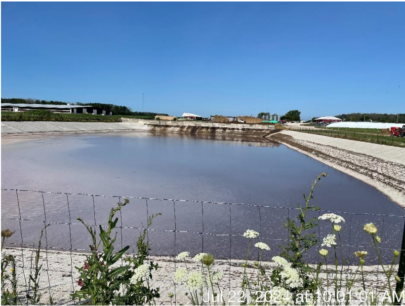
Photo 18. WSF 2 at Augustian Farms LLC located on the northeast portion of the production site. WSF 2 accepts runoff from the feed storage area and manure stacking area. This photo was taken facing northwest.
