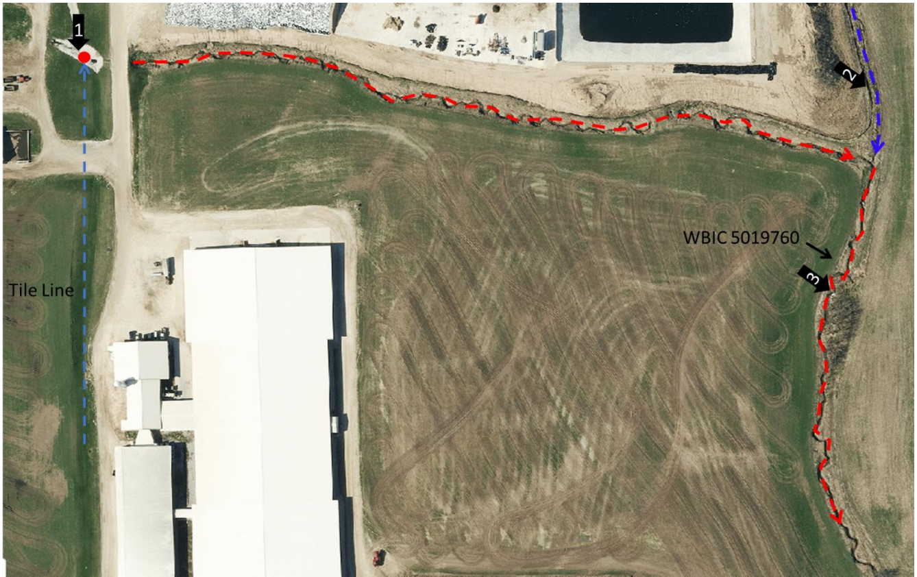
Aerial Map 4. The aerial map above illustrates the flow path of process wastewater that discharged from a tile outlet to the stormwater drainage ditch that runs through the production site. The red dashed arrows represent the flow path of process wastewater through the drainage ditch and through WBIC 5019760. The dashed blue line represented the flow path of WBIC 5019760 before the confluence with the drainage ditch.
