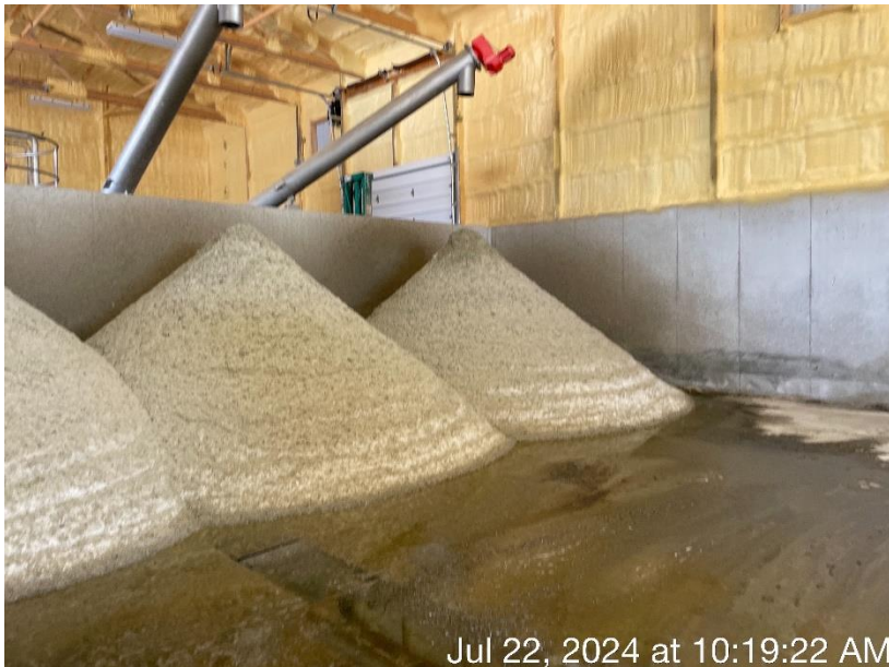
Photo 27. The sand stacking area located in the sand separation building. Leaching from the stacking piles gravity flows to a collection system identified by the black arrow.
