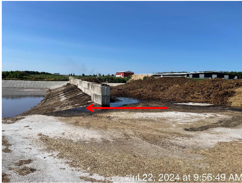
Photo 24. The flow path of runoff from the solid manure stacking area located on the east side of the feed storage area.
