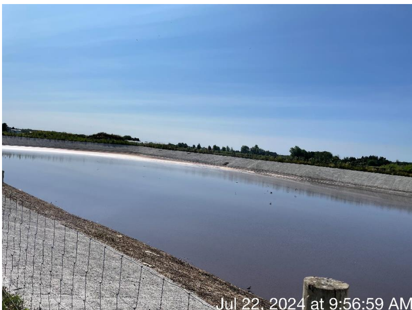
Photo 16. WSF 2 at Augustian Farms LLC located on the northeast portion of the production site. WSF 2 accepts runoff from the feed storage area and manure stacking area. This photo was taken facing southeast.
