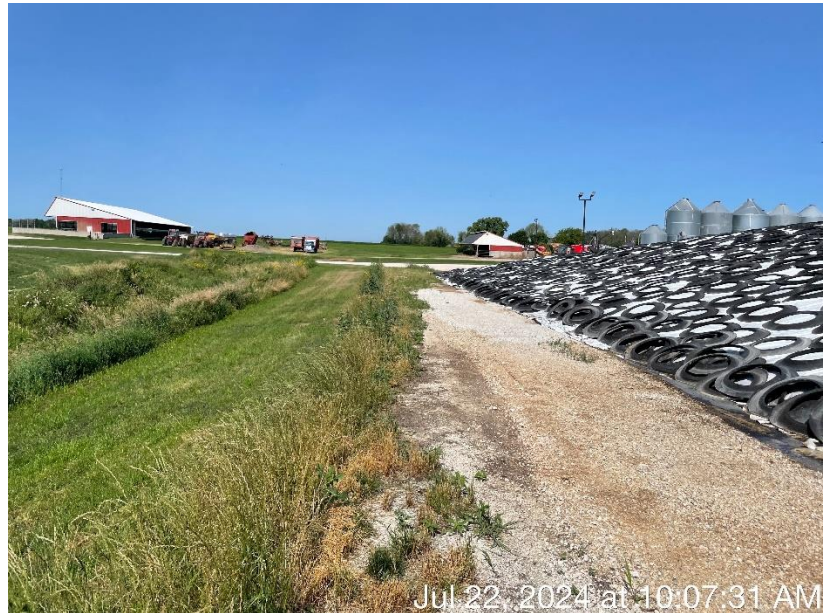
Photo 50. Staining in the gravel along the south side of the feed pad, indicating that leachate and process wastewater had left the concrete apron and flows through the adjacent driveway.
