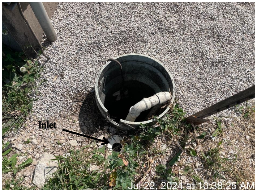
Photo 29. The sump located adjacent to the milking parlor. The sump collects clean water from a gravel layer and pumps the water to a tile line located west of the milking parlor.
