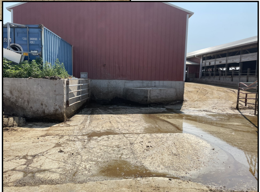
Photo 2 (Right): Looking at the inlet to the runoff collection tank located at the east end of the outdoor concrete feedlot pictured in photo 1. The contents of the collection tank flow into the manure transfer system within the freestall barns where it is then pumped to WSF 1.
