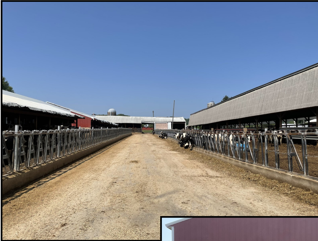
Photo 1 (Left): Looking west across the center of the outdoor concrete feedlot from the east end of the lot. Majority of contaminated lot runoff flows east across the lot where it then enters the collection tank pictured in photo 2.
