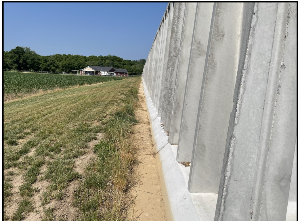
Photo 10 (Right): Looking west along the southern end of the feed storage area where concrete calls were recently installed in 2022. Concrete walls were also installed along the east and western end of the feed pad.
