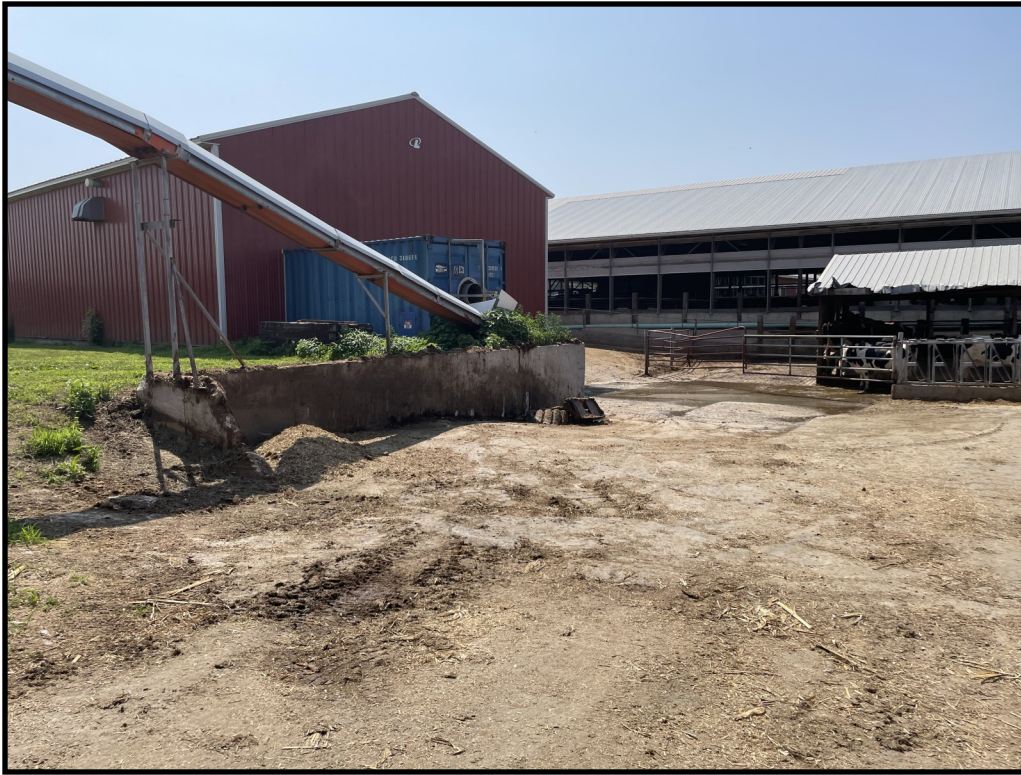
Photo 9 (Left): Looking at the solid manure stacking area located directly north of the runoff collection tank (pictured in photo 2) at the east end of the outdoor concrete lot. Contaminated runoff from the stacking area flows south into the adjacent collection tank.
