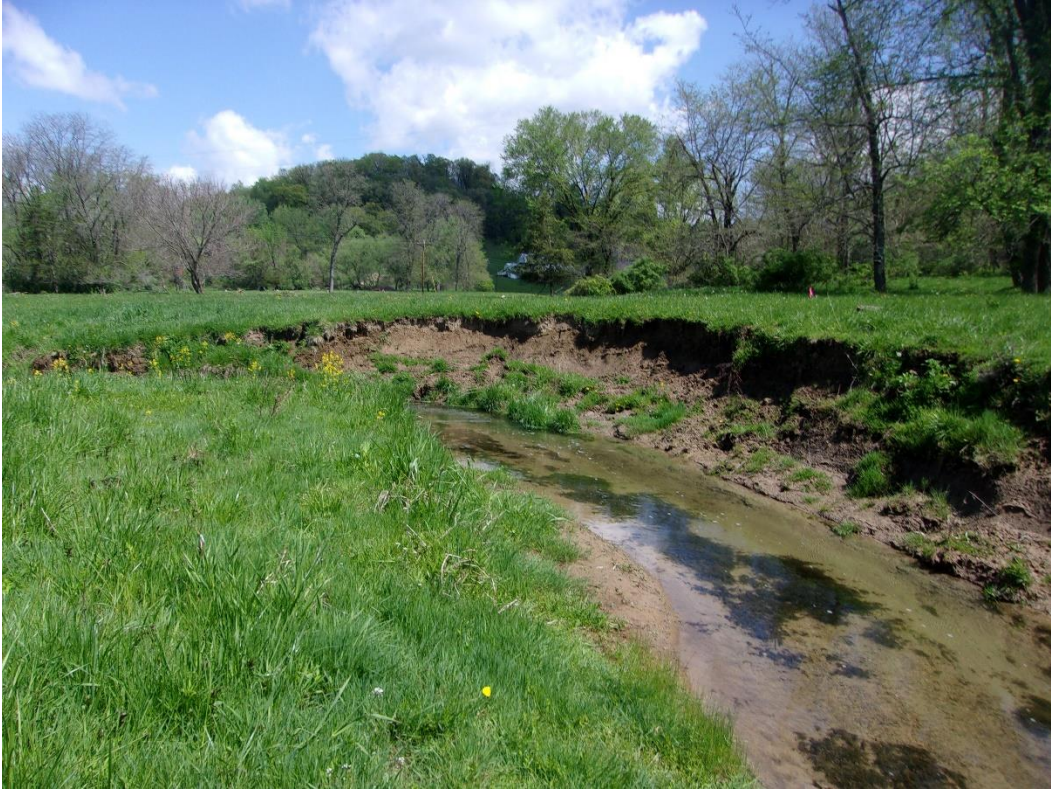
Image 17 – Severe undercut with slump and vegetative overhang
