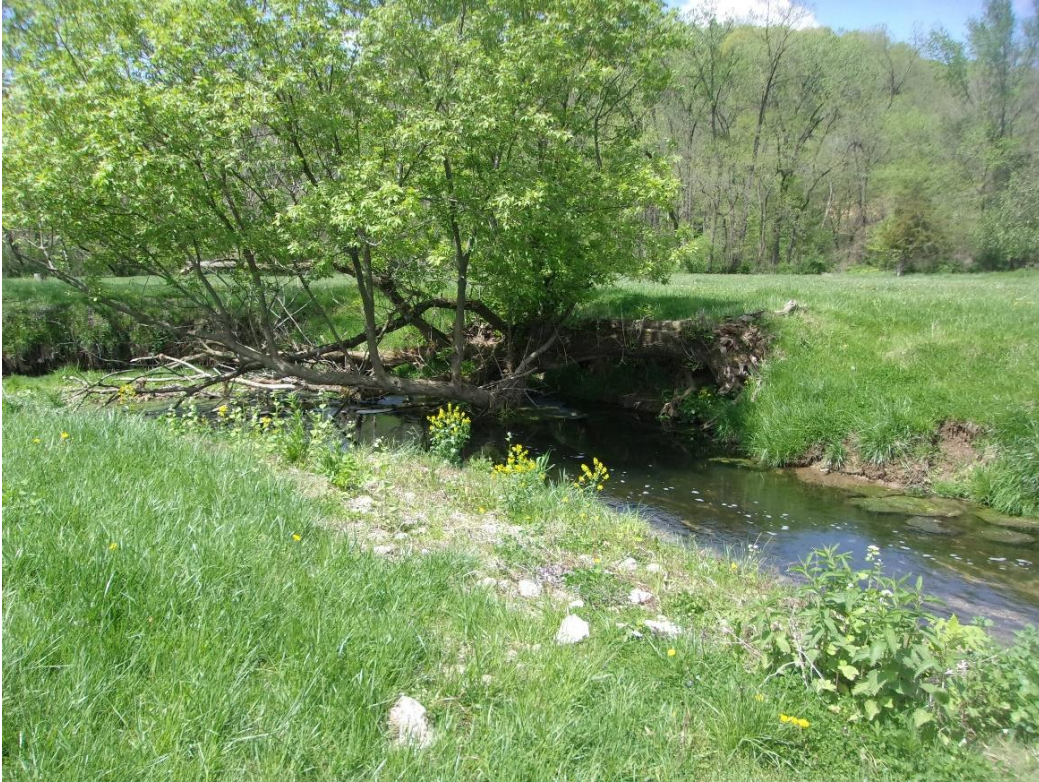
Image 14A – Severe undercut with fallen trees
