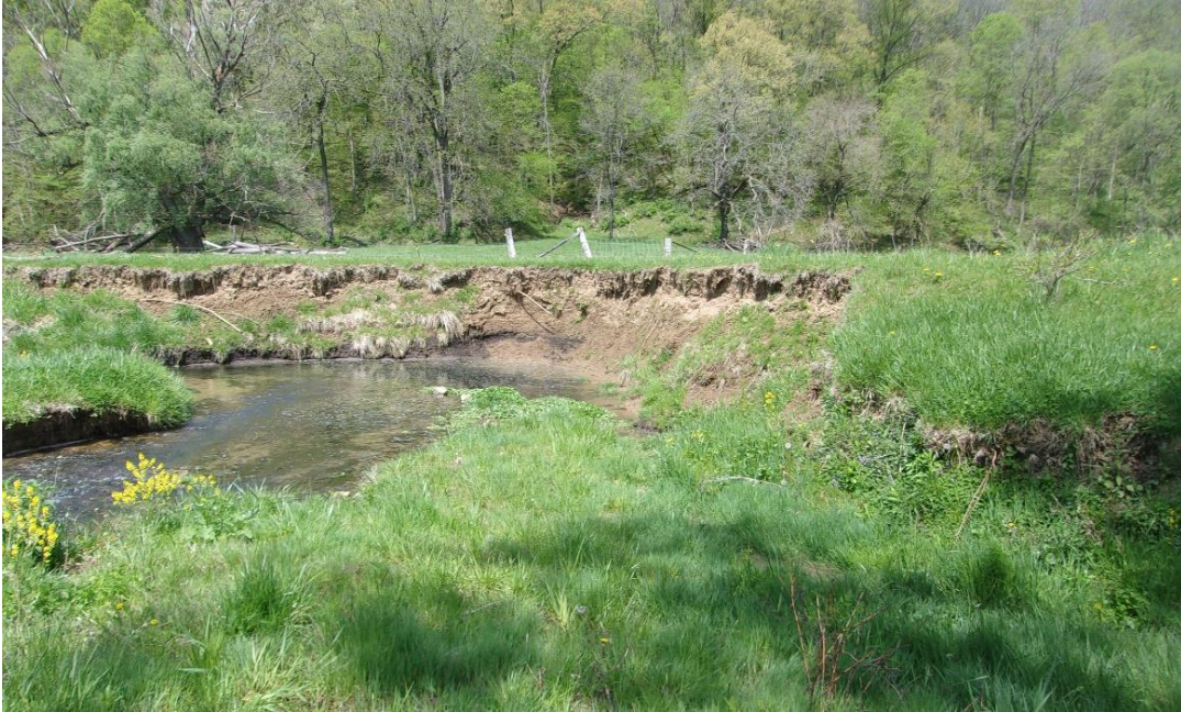
Image 19 – Severe undercut with slump and vegetative overhang
