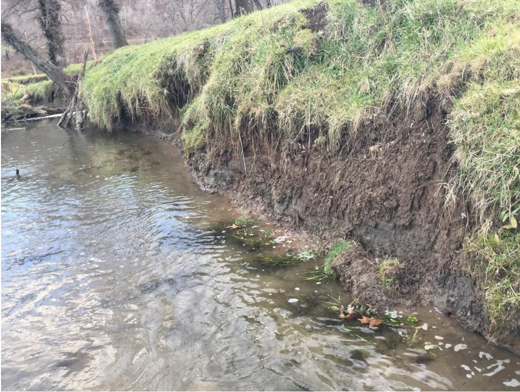
Image 3B – Undercut with vegetative overhang and fallen trees
