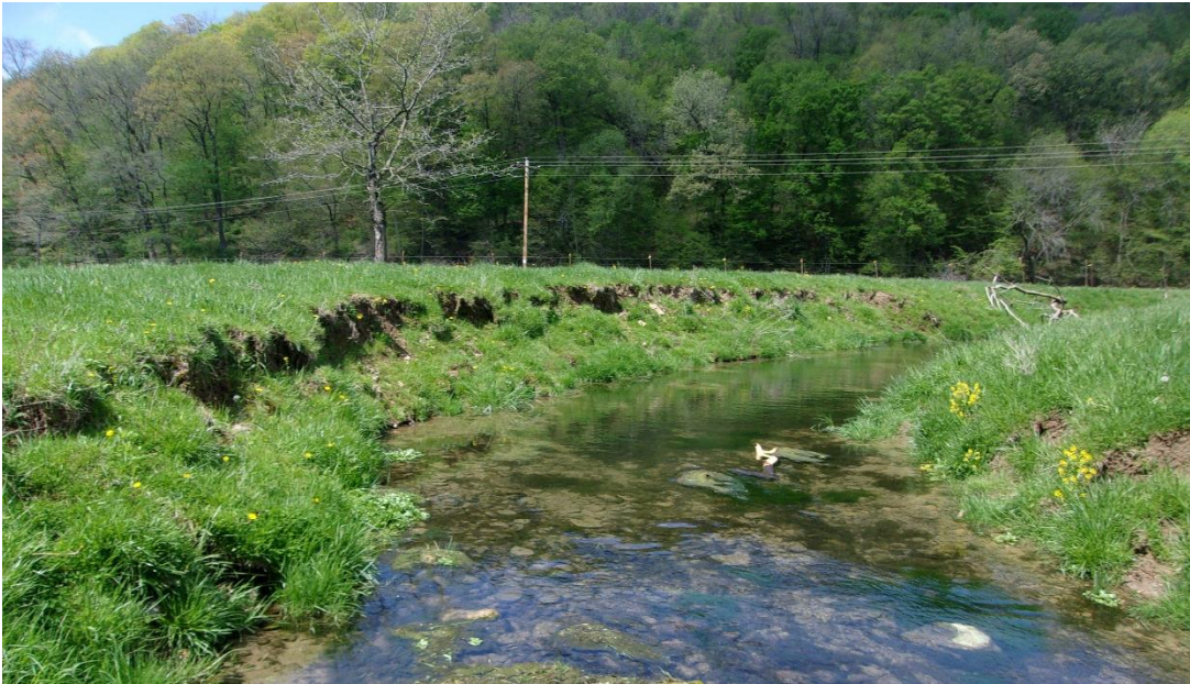
Image 20 – Severe undercut with slump and vegetative overhang
