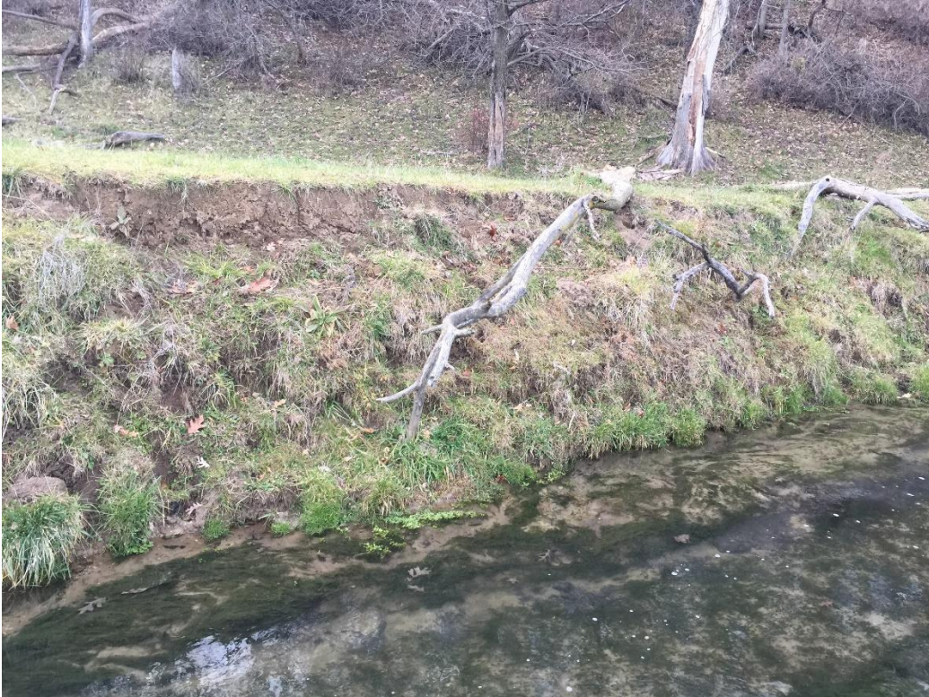
Image 10B – Severe undercut with slump and vegetative overhang
