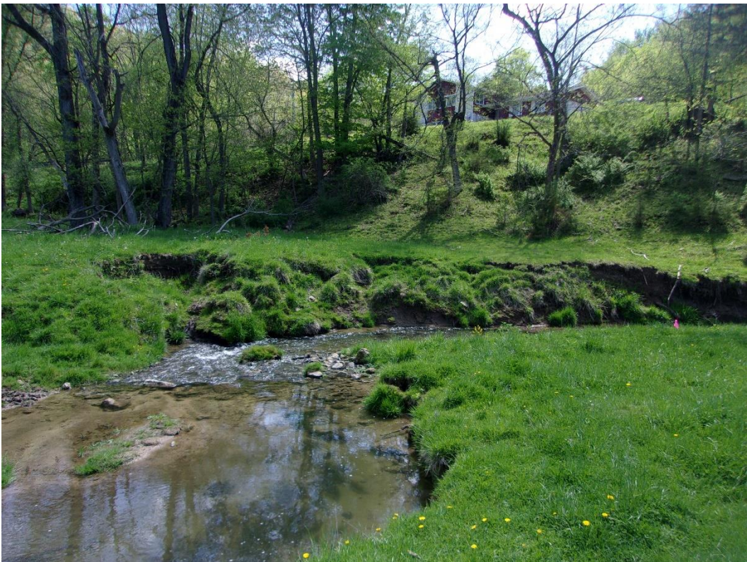
Image 6 – Severe undercut with extreme active slump!
