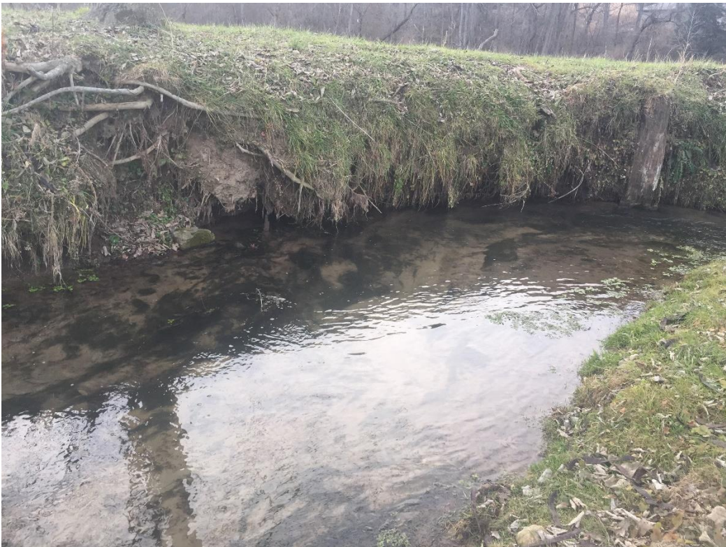
Image 14B – Severe undercut with exposed roots. Stream visibly flows approximately 1.5' under the hollowed out bank with grass and roots draping into the water.
