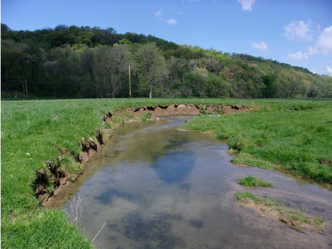
Image 5 – Severe undercut with slump and vegetative overhang
