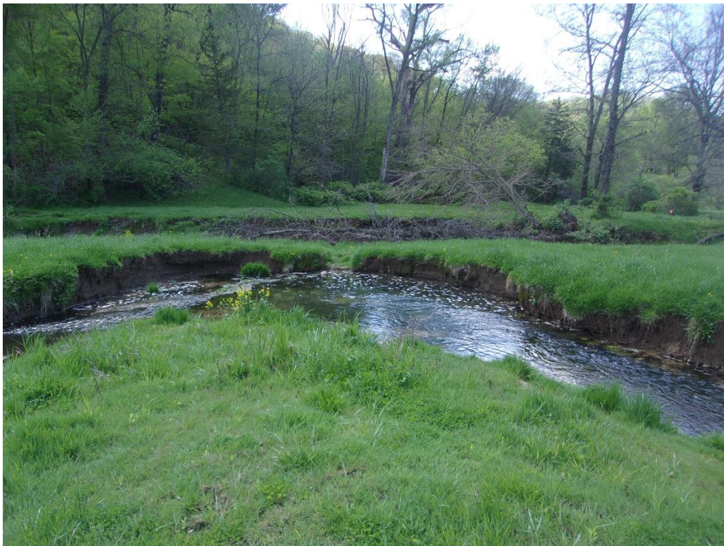
Image 16 – Severe undercut with vegetative overhang
