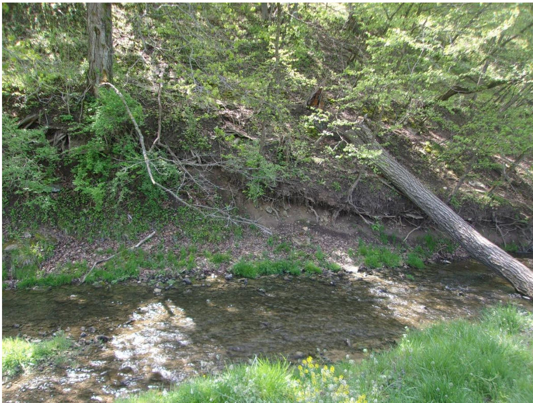
Image 8 – Severe undercut with slump, vegetative overhang, and exposed tree roots
