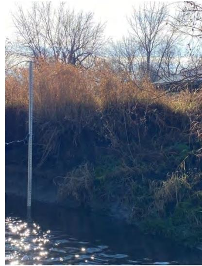
Figure 20.0: Sta. 32+25-34+22 Severe. Bare banks, vegetative overhang, slumps, and channel cross-section is U-shaped.
