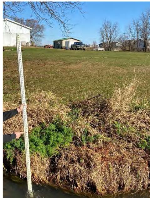
Figure 27.0: Sta. 36+50-37+50 Slight/Moderate. Some bare banks, vegetative overhang, and slumps.
