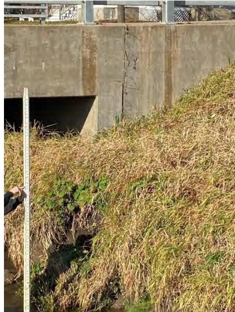
Figure 31.0: Sta. 40+00-40+25 Moderate. Slumps, vegetative overhang, and channel cross-sections U-Shaped.
