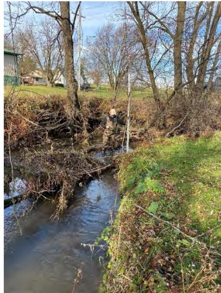
*Figure 44.0: Sta. 56+90-57+35 Moderate/Severe. Bare banks, exposed tree roots, slumps and trees falling into stream.*
