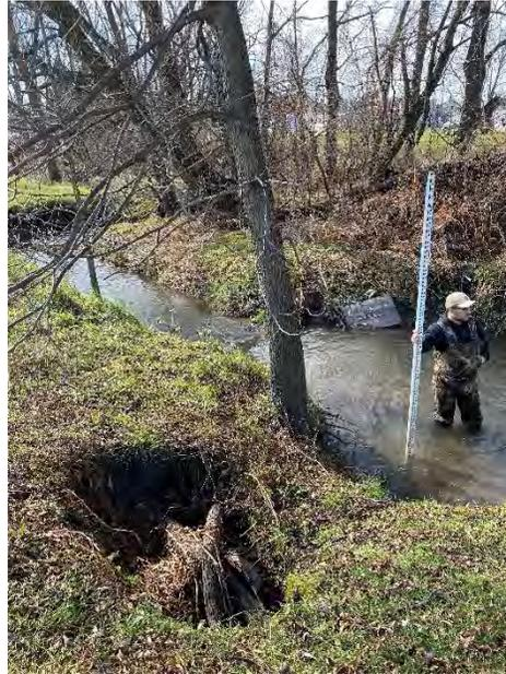
*Figure 42.0: Sta. 56+50-56+90 Moderate. Bare banks, vegetative overhang, slumps, exposed outfall, and channel cross-section is U-Shaped.*
