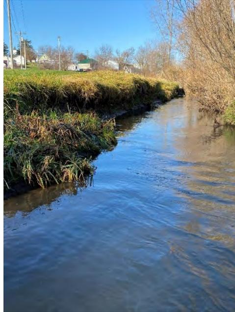
*Figure 16.0: Sta. 22+00-23+50 Moderate/Severe. Bare banks, vegetative overhang, and slumps.*
