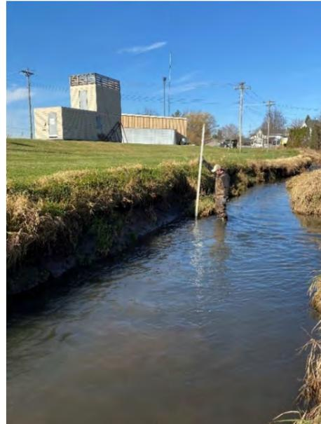
Figure 24.0: Sta. 35+00-35+50 Severe. Bare banks, vegetative overhang, slumps, and channel cross-section U-shaped
