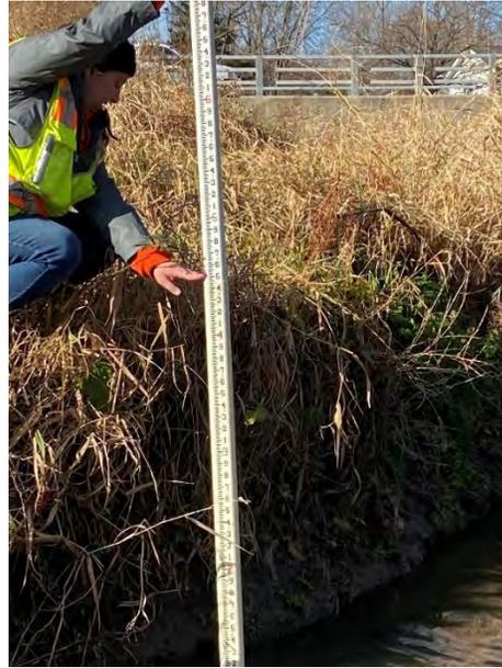
Figure 30.0: Sta. 38+75-40+00 Moderate. Bare banks, slumps, vegetative overhang, and exposed roots.
