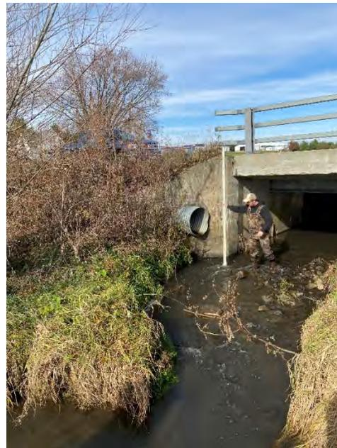
Figure 47.0 Sta. 57+75-58+00 Slight. Vegetative overhang. Culvert within bridge.
