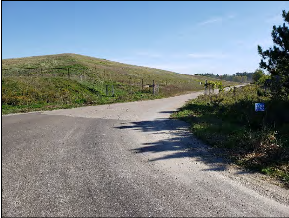
Photo 1: Gate and access road into the facility. Looking east; southwest corner of Landfill No. 3171 on left side of photograph.
