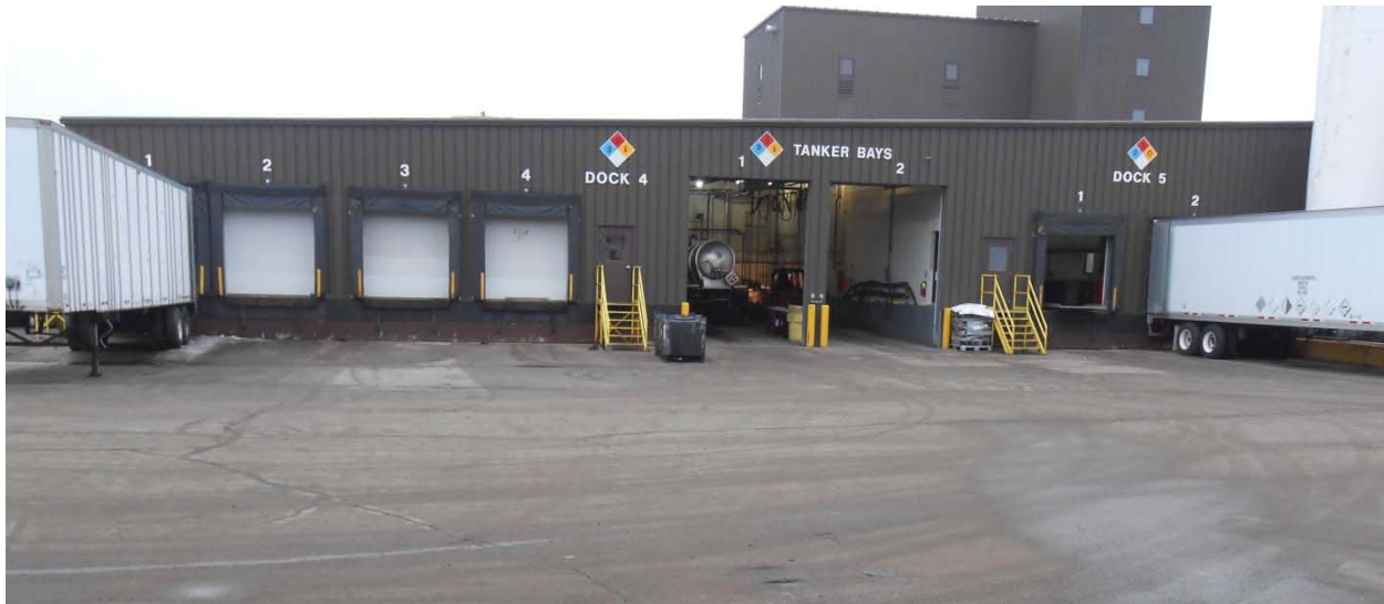
Photo taken April 9, 2013 Looking west at east side of the E-II Warehouse Building
