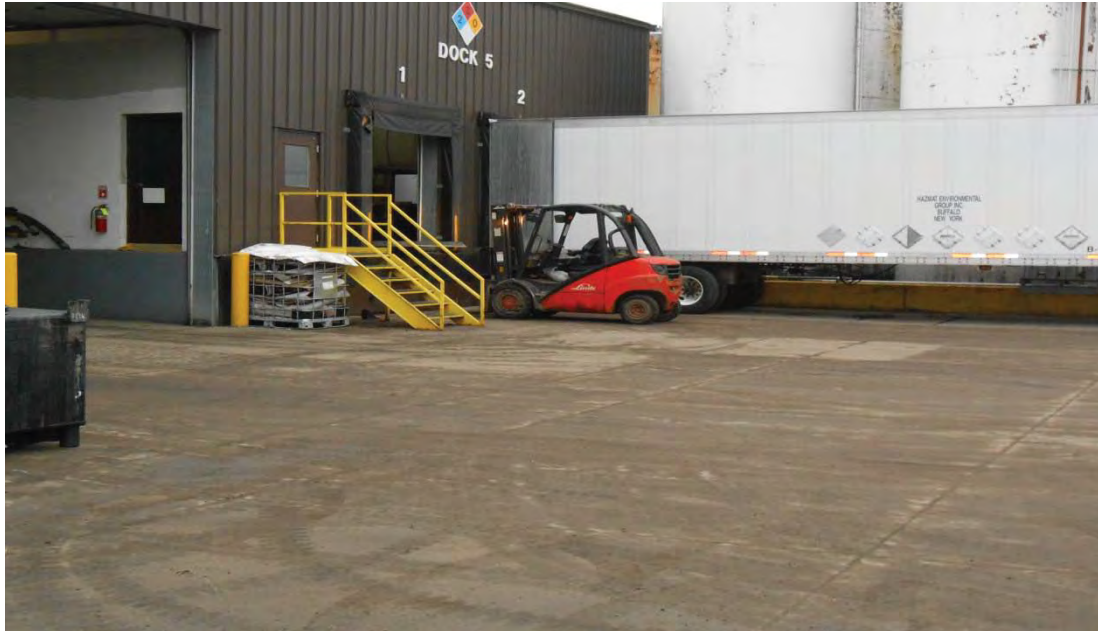
Exterior view of Dock 5 of E-II Warehouse Building looking northwest.
