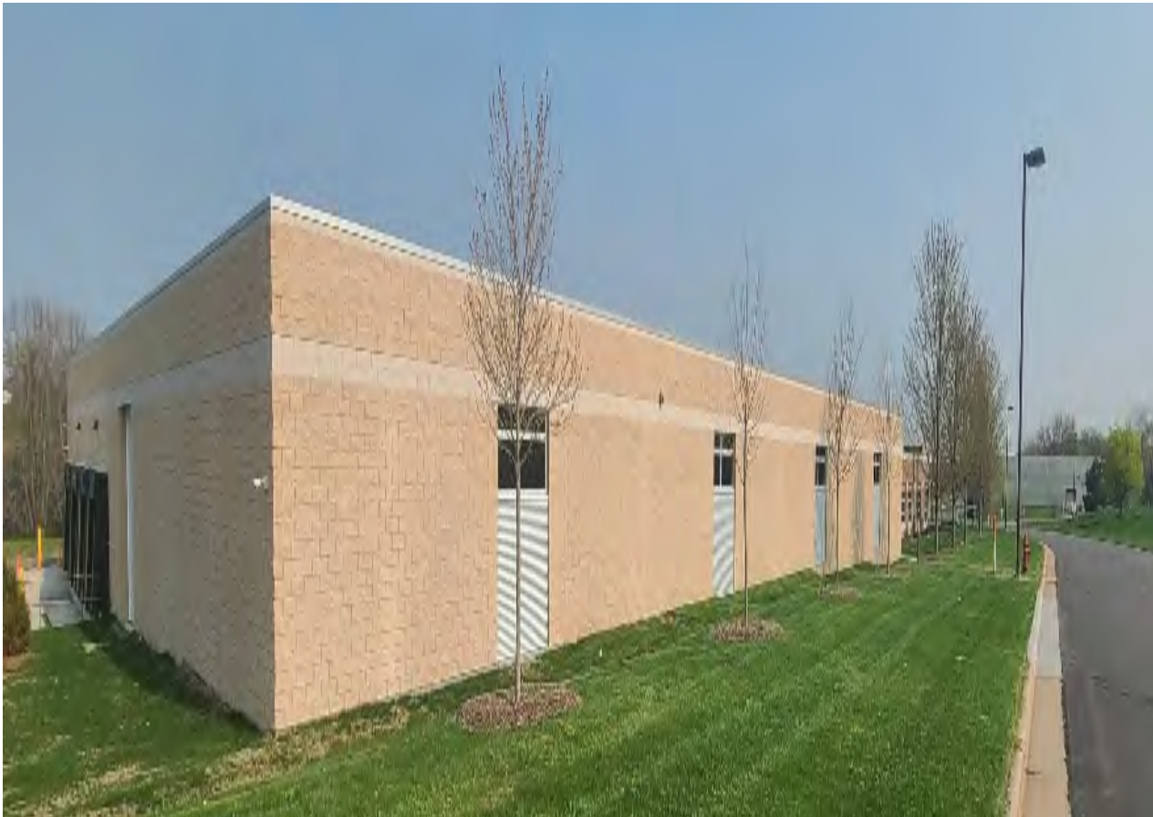
Photo #11 - Westside Building (Outside - West)
