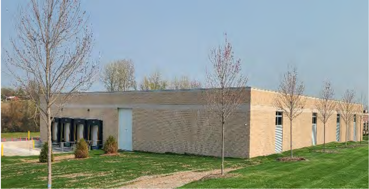
Photo #10 - Northside Building (Outside - North)
