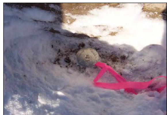
4 SOIL MARKER INSTALLATION CONTINUES.
