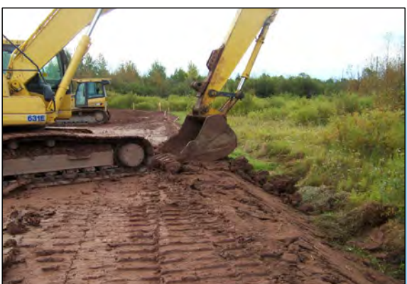
6 SLOPE IS INSTALLED ON EAST SIDE OF AREA H.
