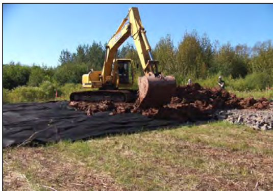
5 EXCAVATOR IS USED TO BEGIN PLACEMENT OF CLAY BACKFILL IN AREA H.
