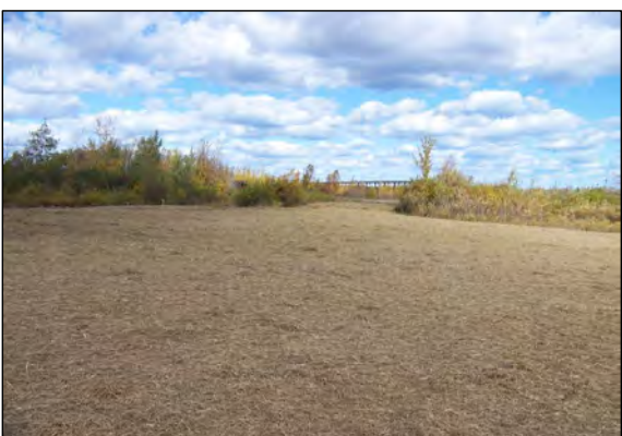
5 AREA G SEEDING COMPLETED.
