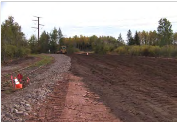
6 TOPSOIL PLACEMENT IN AREA G IS COMPLETED.
