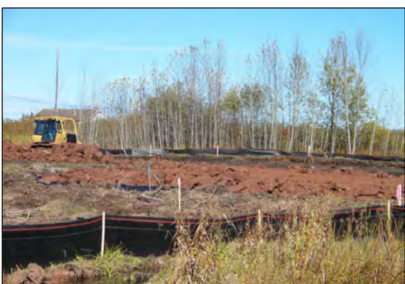
6 PLACING CLAY BACKFILL IN AREA B.
