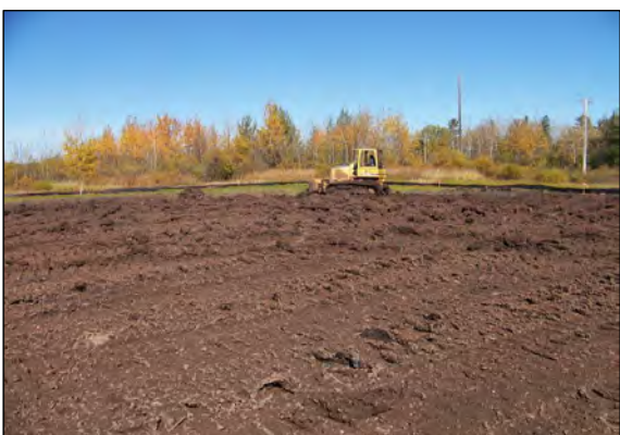
3 MATERIAL CUT FROM AREA B BEING PLACED AND GRADED IN AREA A.
