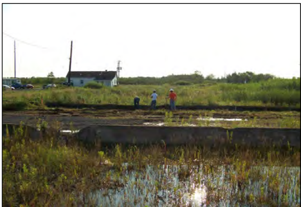
5 INSTALLATION OF EROSION CONTROLS CONTINUES THIS WEEK.
