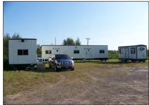
1 OFFICE AREA MOBILIZATION BEGINS.
