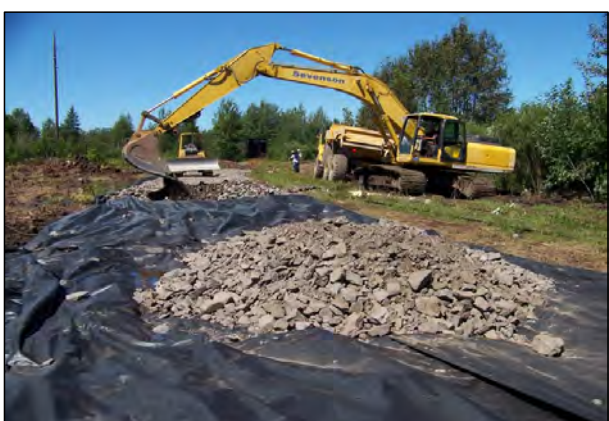
2 INSTALLATION OF FABRIC AND STONE IN AREA G TO BRIDGE OVER EXTREMELY WET CONDITIONS.
