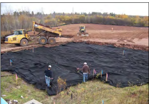
2 CREW DEPLOYS GEOTEXTILE PRIOR TO CLAY GENERAL FILL PLACEMENT IN AREA B.
