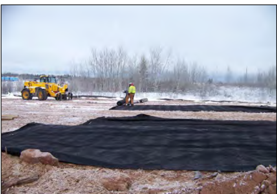
5 CREW DEPLOYS GEOTEXTILE PRIOR TO FILL PLACEMENT.
