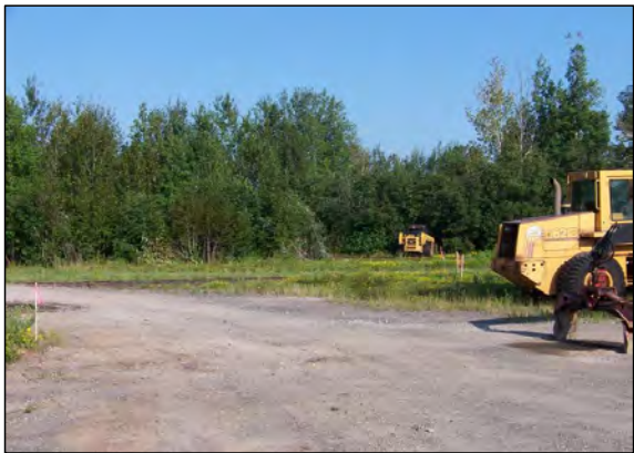
3 CLEARING CONTRACTOR ONSITE.
