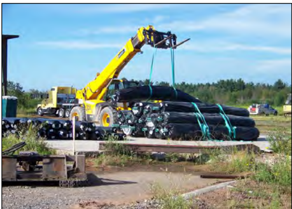
6 REACTIVE CORE MAT IS DELIVERED TO JOBSITE.
