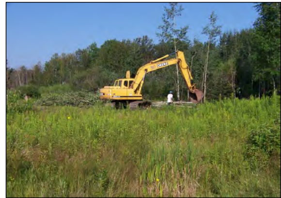
4 CLEARING CONTRACTOR ONSITE.
