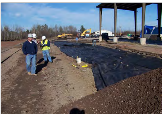
3 INSTALLATION OF ROAD BASE SURFACE COVER IN AREA B.
