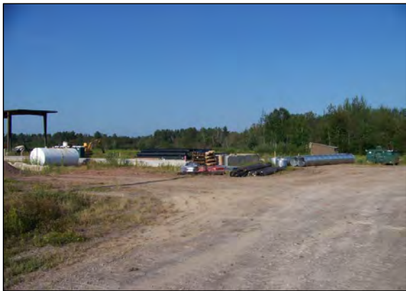
2 MATERIAL FOR PROJECT BEING DELIVERED TO SITE.
