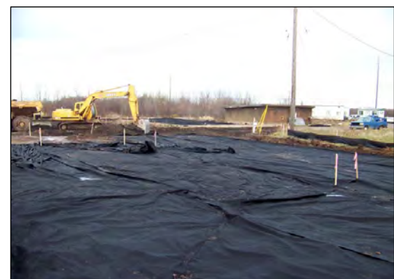
4 SUBGRADE OPERATIONS IN AREA B CONTINUE. GEOTEXTILE IS DEPLOYED PRIOR TO SOIL COVER INSTALLATION.
