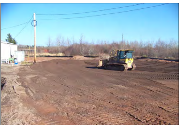
2 SUBGRADING OPERATIONS CONTINUE IN AREA B.
