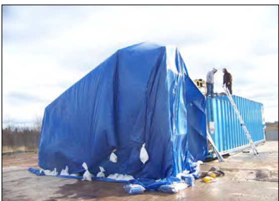
3 CREW CONSTRUCTS SHELTER AROUND WATER TREATMENT SYSTEM.
