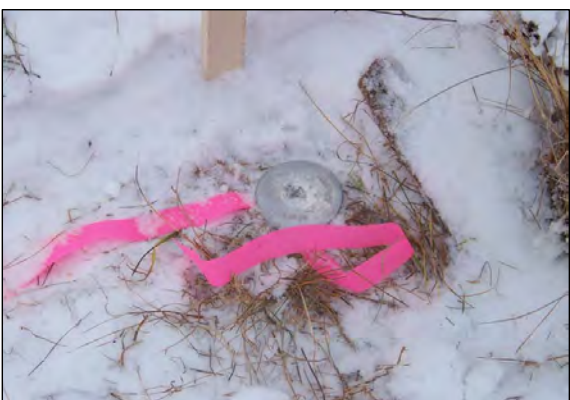
2 SURVEYORS ONSITE TO INSTALL SOIL MARKERS AT CORNERS OF SURFACE COVER AREAS.
