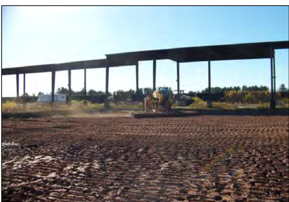
6 MATS ARE MOVED TO SOUTHERN END OF AREA B IN PREPARATION FOR TOPSOIL PLACEMENT.
