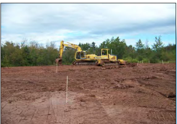
2 CLAY BACKFILL IS ADDED IN AREA H TO CREATE A PITCH FOR DRAINAGE AWAY FROM TRACKS. EXCAVATOR WORKS SLOPE ALONG TRACKS IN PREPARATION FOR TAPER STONE.
