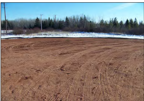
3 AREA A COVER IS COMPLETED.
