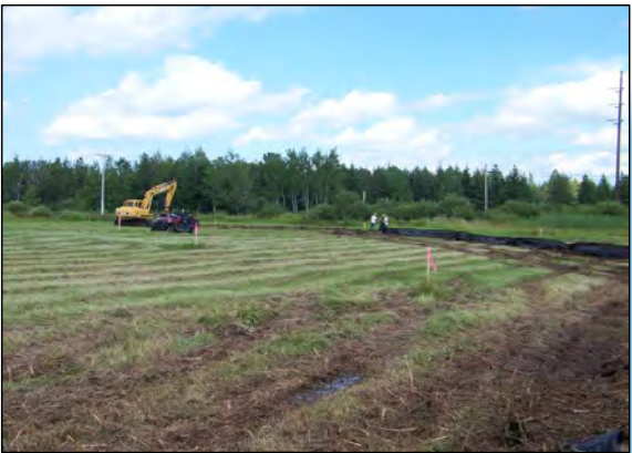
5 CREW INSTALLS SILT FENCE IN WORK AREAS.
