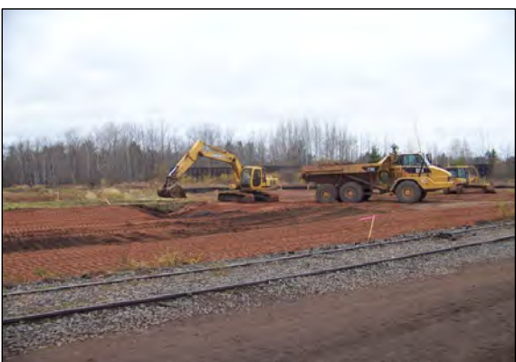
5 BACKFILL IS PLACED IN AREA B.
