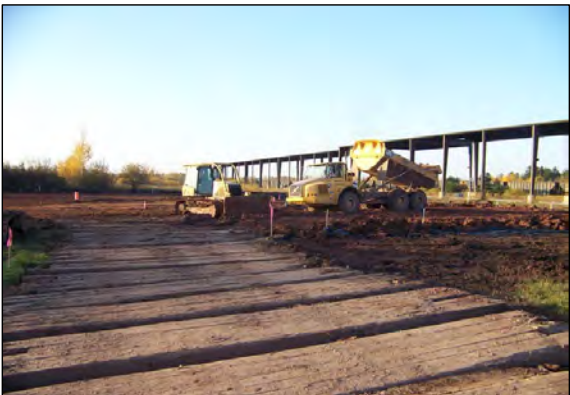
5 SURFACE COVER INSTALLATION IN AREA B.
