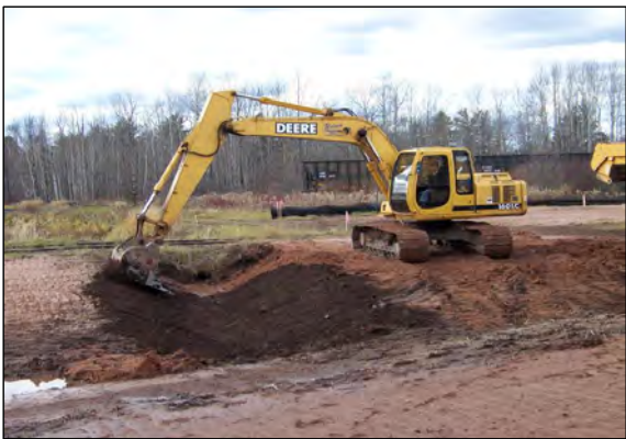
6 INSTALLATION OF CLAY VEGETATED SURFACE COVER IN AREA B.
