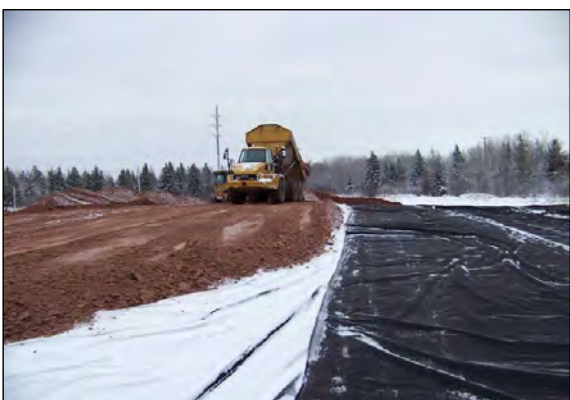
3 GENERAL FILL IS PLACED IN AREA A.
