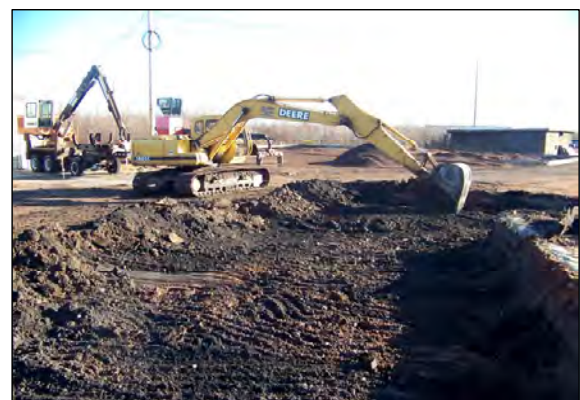
1 SUBGRADING OPERATIONS CONTINUE IN AREA B.
