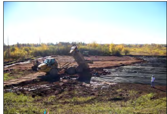
4 SURFACE COVER INSTALLATION IN AREA B.
