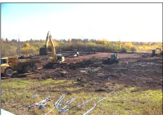
2 SUBGRADE LEVELING IN AREA B.
