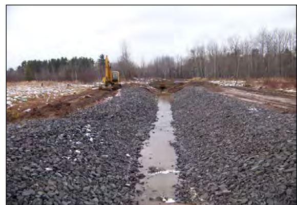
1 A VIEW OF THE OUTFALL DITCH.
