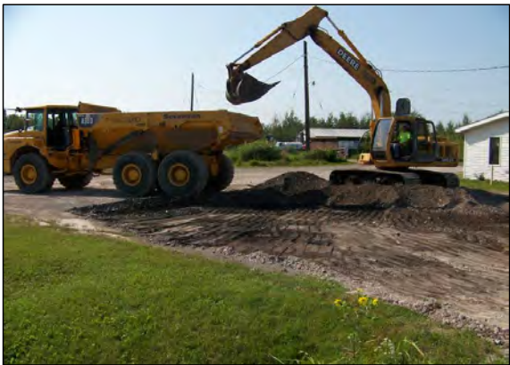
3 CONSTRUCTION ENTRANCES ARE INSTALLED.
