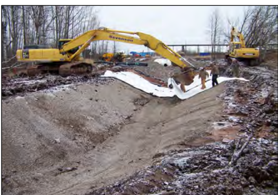
6 CREW DEPLOYS RCM IN OUTFALL DITCH.
