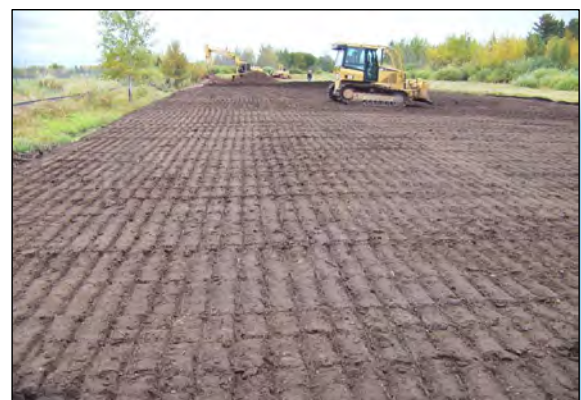
1 TOPSOIL PLACEMENT IN AREAS S1 & S2.
