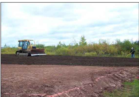
3 TOPSOIL PLACEMENT IN AREA H IS COMPLETED.
