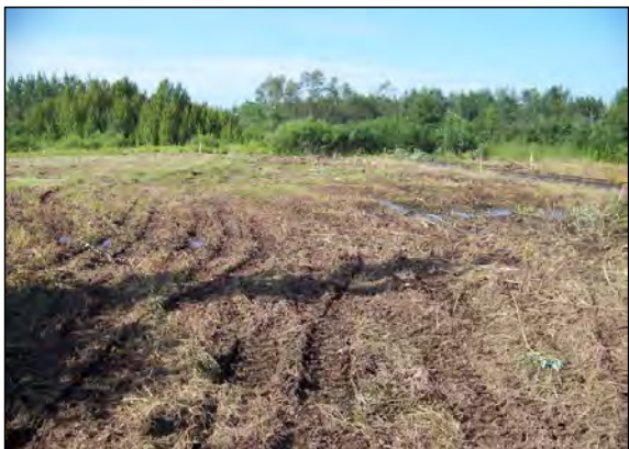
6 AREA H AFTER CLEARING.
