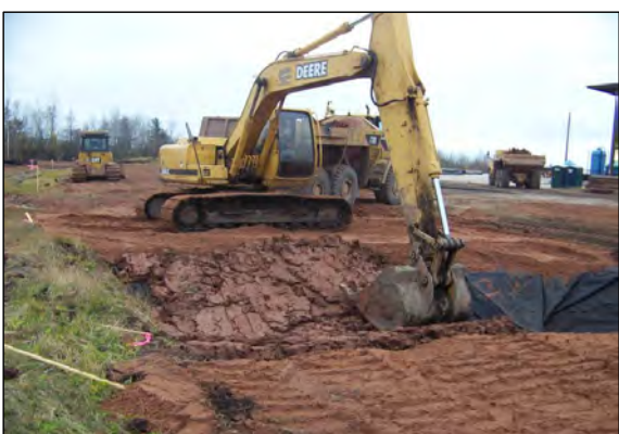
6 BACKFILL IS PLACED IN AREA B.
