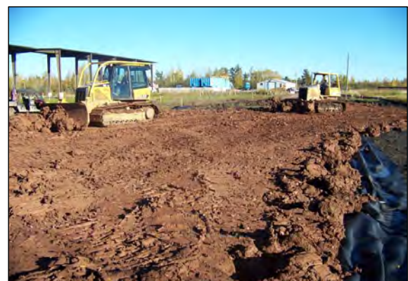
1 SURFACE COVER INSTALLATION IN AREA B.
