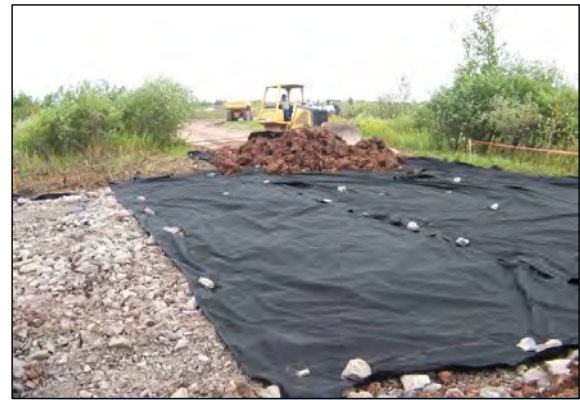
4 CLAY BACKFILL IS PLACED IN AREA H.
