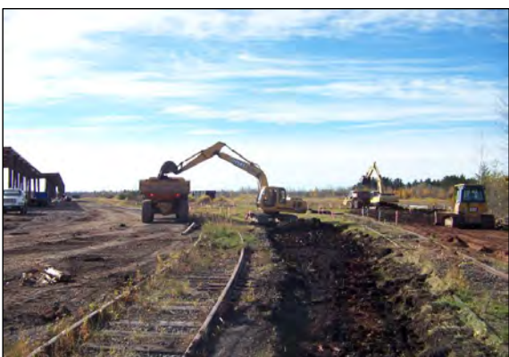
3 CUT / FILL OPERATIONS IN AREA B CONTINUE.
