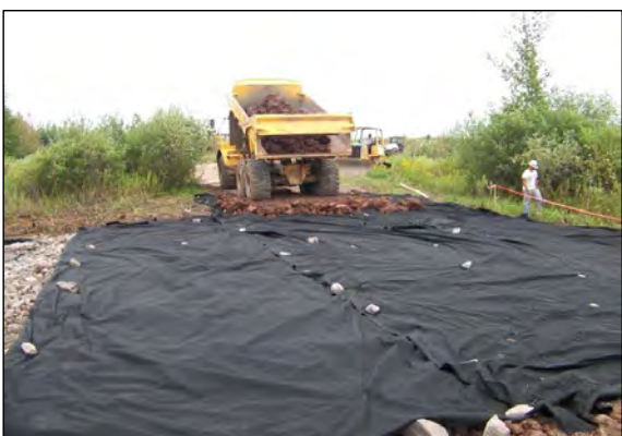
3 CLAY BACKFILL IS PLACED IN AREA H.
