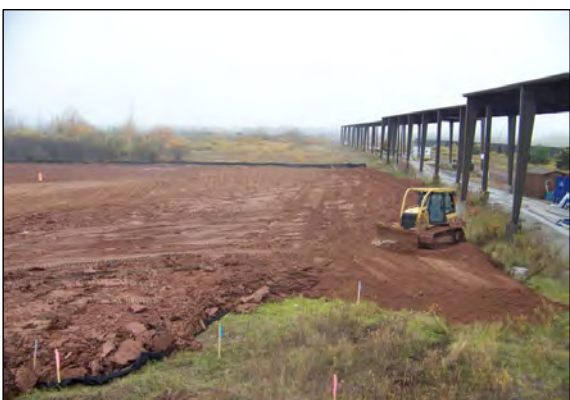
3 GENERAL FILL IS PLACED ALONG DRIP TRACK IN AREA B.
