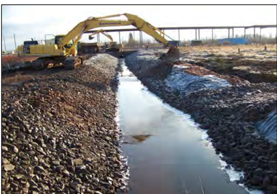
3 RIP RAP PLACEMENT CONTINUES IN OUTFALL DITCH.
