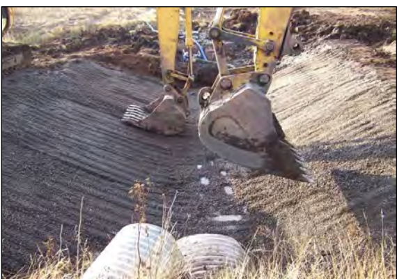
2 SECTION OF OUTFALL DITCH IS EXCAVATED; GRAVEL IS ADDED TO DITCH PRIOR TO RCM.
