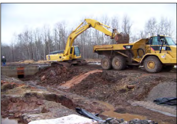
2 OUTFALL DITCH EXCAVATION CONTINUES.
