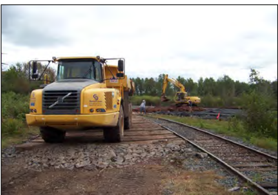
2 CLAY BACKFILL IS PLACED IN AREA G; EXCAVATOR IS USED TO BEGIN INSTALLATION TO PREVENT TEARING GEOTEXTILE.
