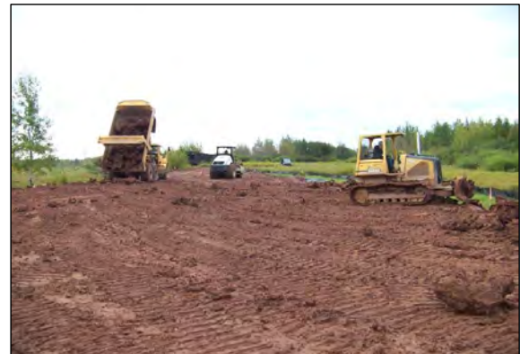
4 CLAY BACKFILL CONTINUES TO BE PLACED IN AREA S2.
