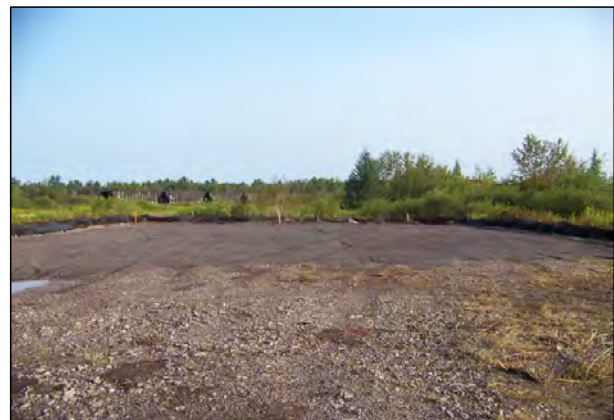
4 AREA F2 AFTER 2.5 INCHES OF RAIN; NO SETTLEMENT IN AREA.
