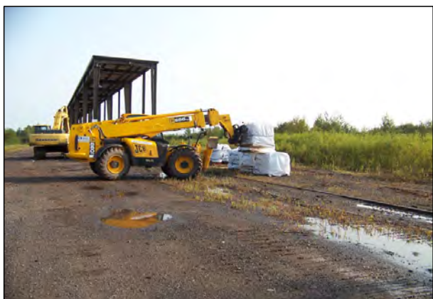
6 CONSTRUCTION MATERIALS CONTINUE TO ARRIVE ON SITE.
