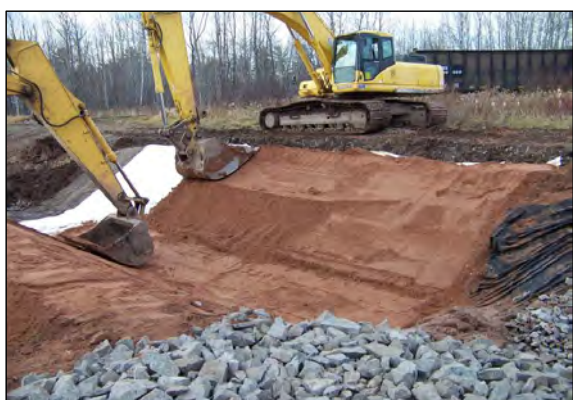
6 GENERAL FILL PLACEMENT.
