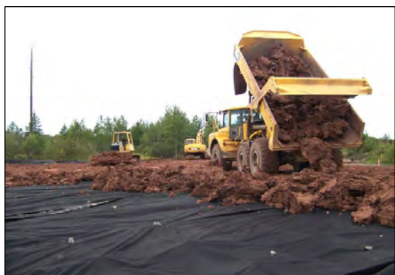
3 CLAY BACKFILL PLACEMENT CONTINUES IN AREA G.
