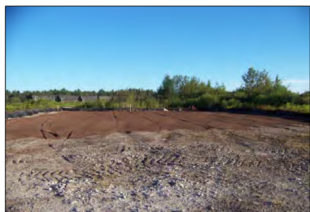
1 AREA F2 CAPPING IS COMPLETED MONDAY 8-16-2010.
