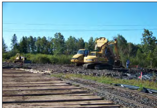
4 PLACEMENT OF GEOTEXTILE AND STONE FOR BRIDGING IN AREA G IS COMPLETED TODAY.
