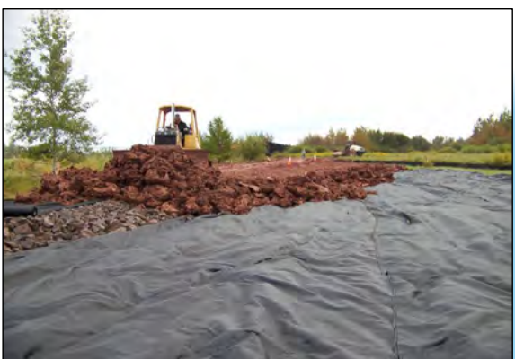
3 CONTINUING TO PLACE CLAY BACKFILL IN AREA S2.
