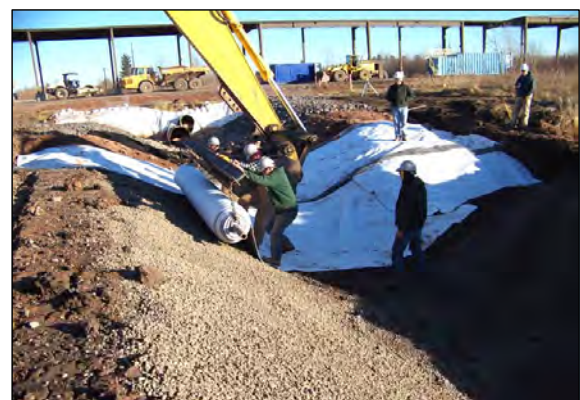
4 RCM IS INSTALLED IN DITCH.
