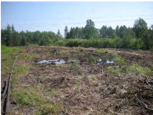
Photograph 1 – Looking southeast at Area G
