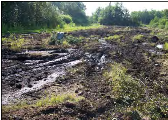
5 AREA G AFTER CLEARING.
