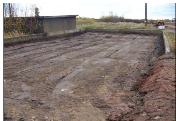
4 IN PREPARATION FOR SUBGRADE FILL PLACEMENT, EXISTING MATERIAL IN CONCRETE BASIN IS STABILIZED.
