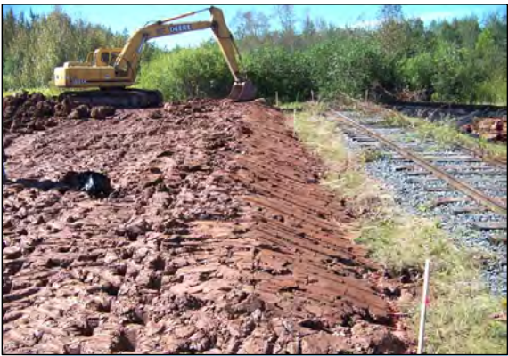
5 INSTALLING SLOPE ALONG TRACKS IN AREA H.
