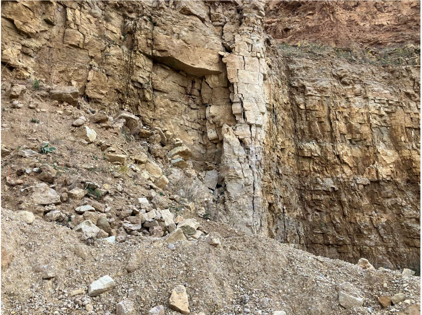
Photo 17 (SEH, October 2025) Gudgeon Pit Quarry – Similar to observations made at Seas Branch Quarry, some larger voids/cavities were observed but are not entirely naturally occurring features. The example above shows evidence of both previous mining impacts to the bedrock surface along with natural weathering and separation of rock from the rock face. Rockfall and weathered material are still present below the cavities, deposited as recent colluvium along the base of the quarry wall. While and fractures, no evidence of sinkholes or caverns was observed at the site. As commonly found in carbonate bedrock conditions, the frequency and size of voids decrease with depth on the quarry wall as dissolved carbon dioxide concentrations generally decrease with depth. The concentration of dissolved carbon dioxide nearer the surface generally contributes to the dissolution of minerals. The carbonate rocks above the shaly layer have more frequent fracturing than the carbonate rocks below the shaly layer, with bedrock fractures evenly distributed throughout each unit. See Photo 14 for more descriptive details.
