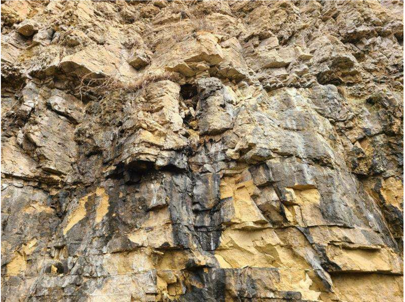
Photo 5 (SEH, April 2026) Seas Branch Quarry – Closer view of mineral precipitates (and epilithic algae) on rock surface along quarry walls. Fresher rock face (yellow) where surficial staining had not occurred or stained surface has broken off exposing fresh rock. Bedrock fractures are evenly distributed throughout the layer not every fracture becomes a pathway for percolating water. Depth to the uppermost water table is estimated to be approximately 90 feet below the quarry floor. See Photo 1 for more descriptive details.
