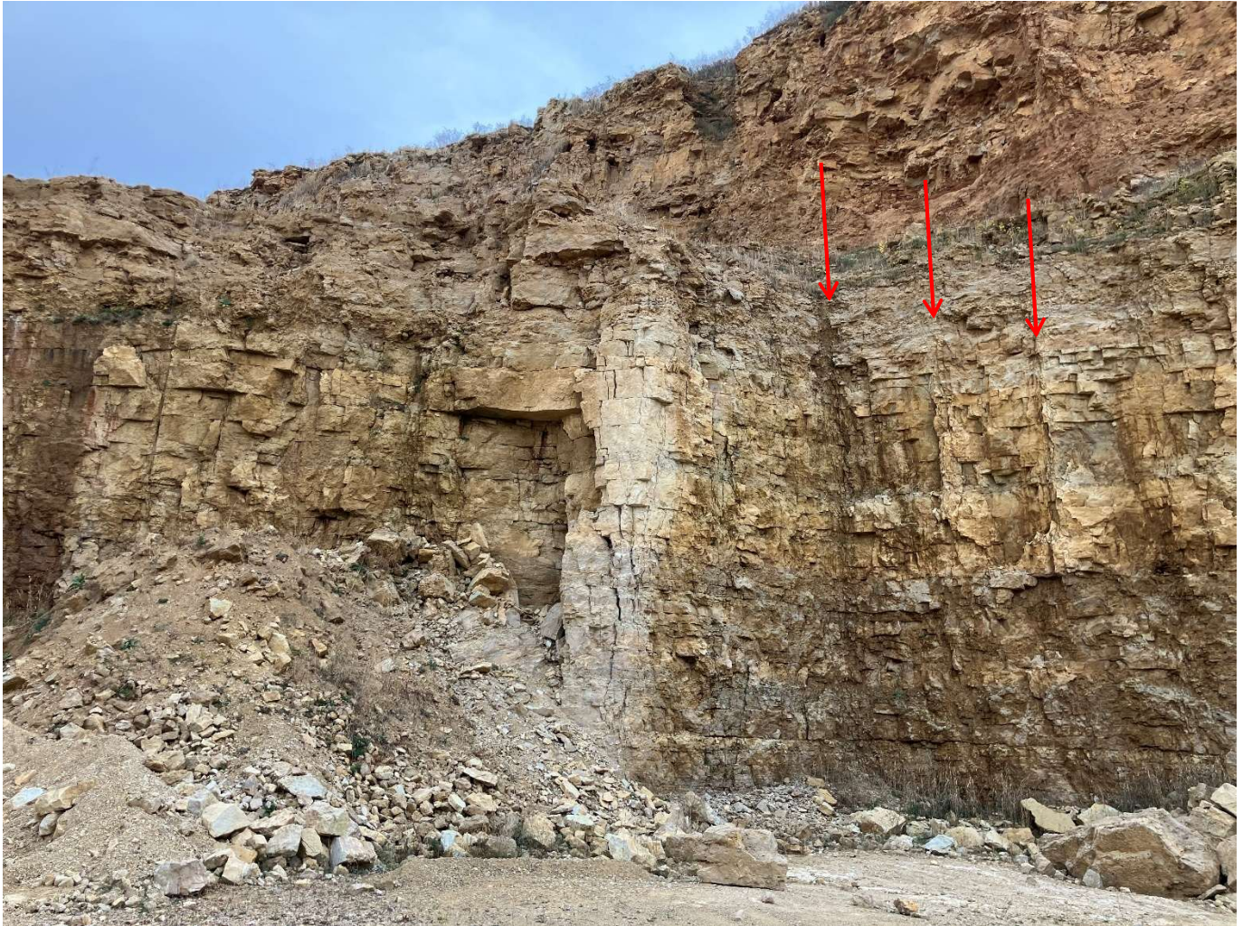
Photo 15 (SEH, October 2025) Gudgeon Pit Quarry – Similar to Seas Branch Quarry, the bedrock outcrop shows evidence of natural fractures, with greater heterogeneity, thinner bedding, and increased fracturing observed in the upper bedrock layer of the Oneota Dolomite and transitioning to a more homogeneous and thicker bedded unit in the lower bedrock layer of the Oneota Dolomite below. The shaly layer between the upper and lower bedrock layers within the Hager City Member of the Oneota Dolomite shows evidence of being a pathway for surface water percolating downward through the unsaturated bedrock; these pathways in the unsaturated bedrock layer may locally intersect the quarry wall and seasonally form seeps as noted by darker mineral precipitates on rock surface at/below contact (note darker mineral precipitation on rock surface at/below contact). The carbonate rocks above the shaly layer have more frequent fracturing than the carbonate rocks below the shaly layer, with bedrock fractures evenly distributed throughout each unit. Arrows pointing to evidence of evenly spaced blasting and mining activities of the quarry. See Photo 14 for more descriptive details.
