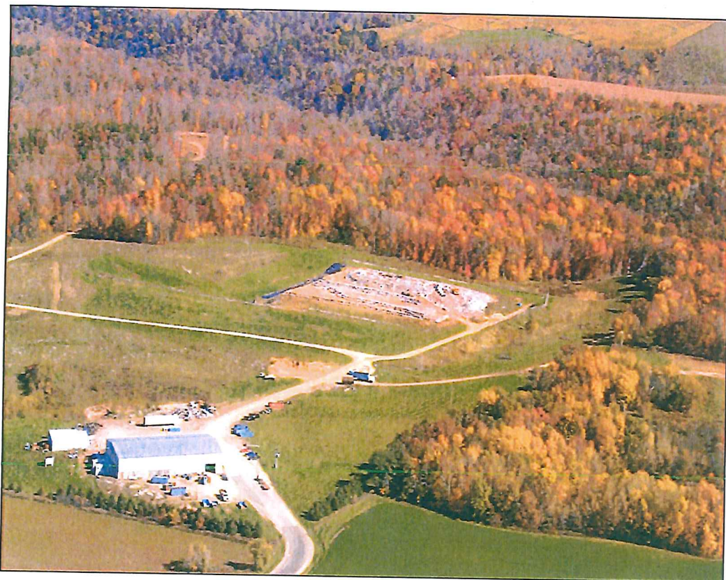
(3) View toward northeast showing access roads (to be used for clay haul)
