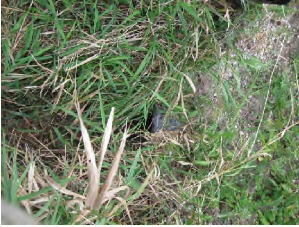
W-2 culvert near W2-6w
