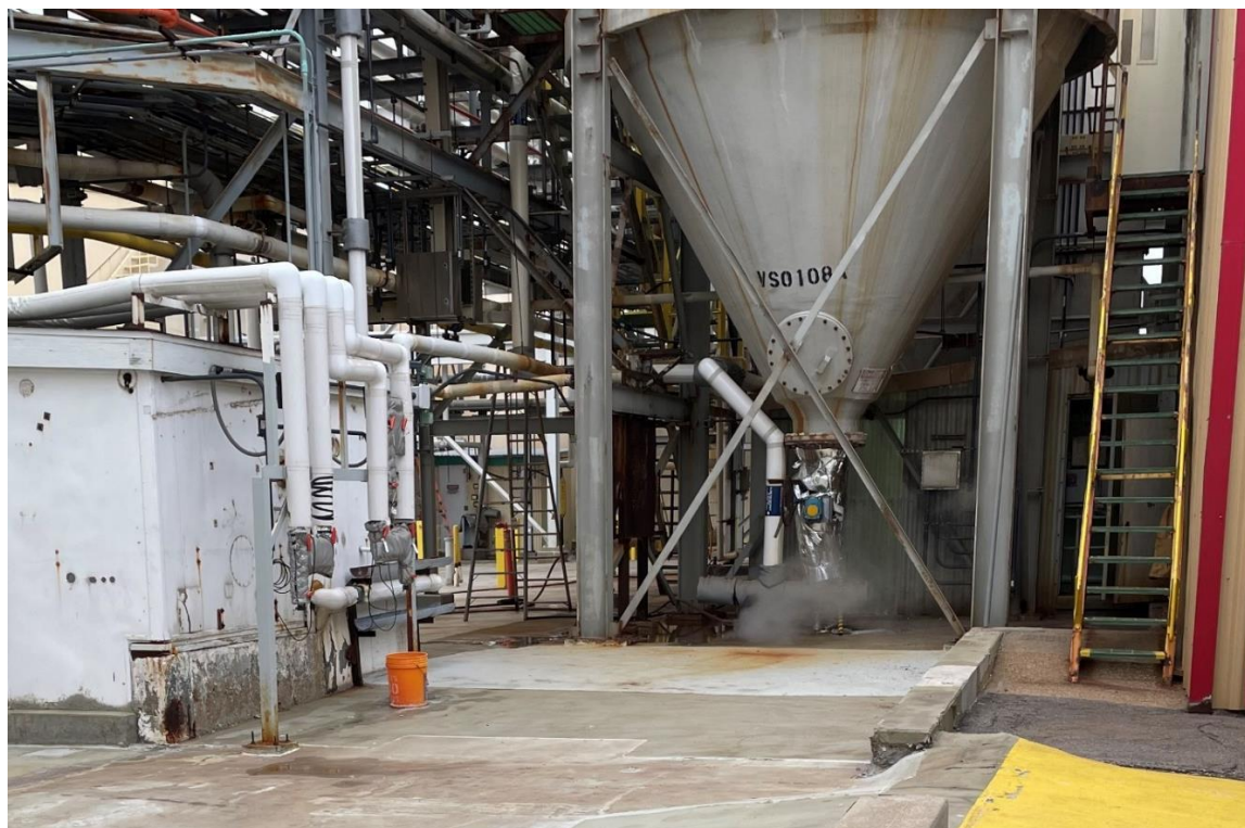
Figure 3 - Clarifier Purge Pit
