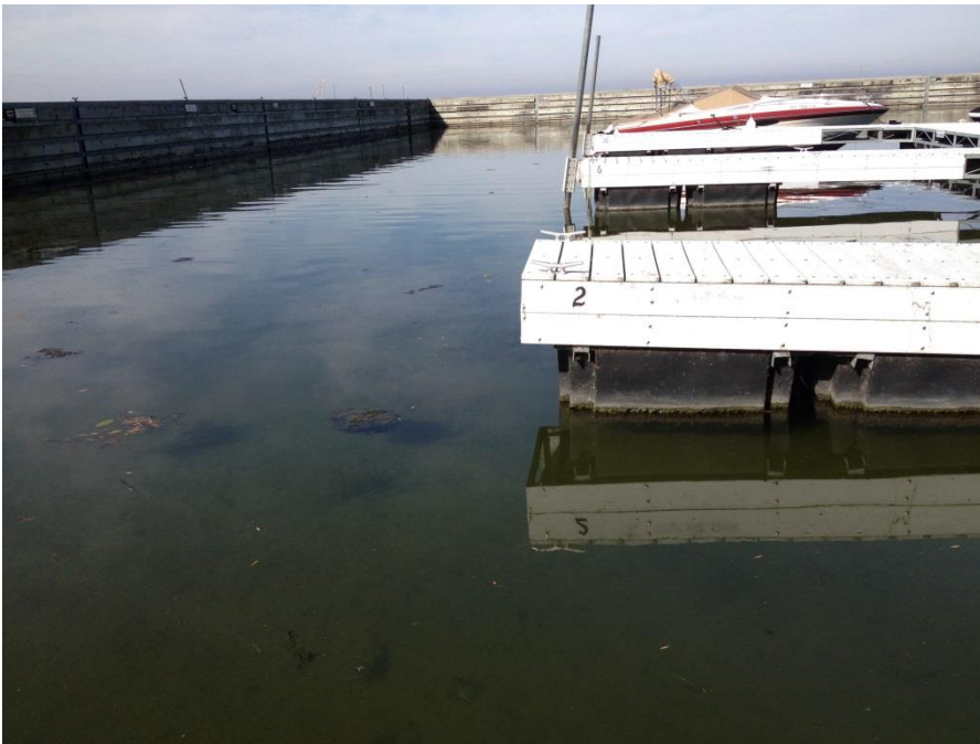
Photo 4. Shallow depths along south edge of floating finger piers
