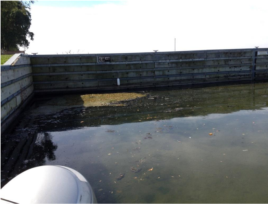
Photo 3. Sediment accumulation in Southeast Corner of harbor
