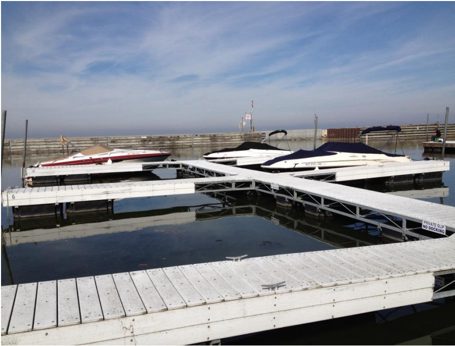
Photo 5. Floating Finger Pier System
