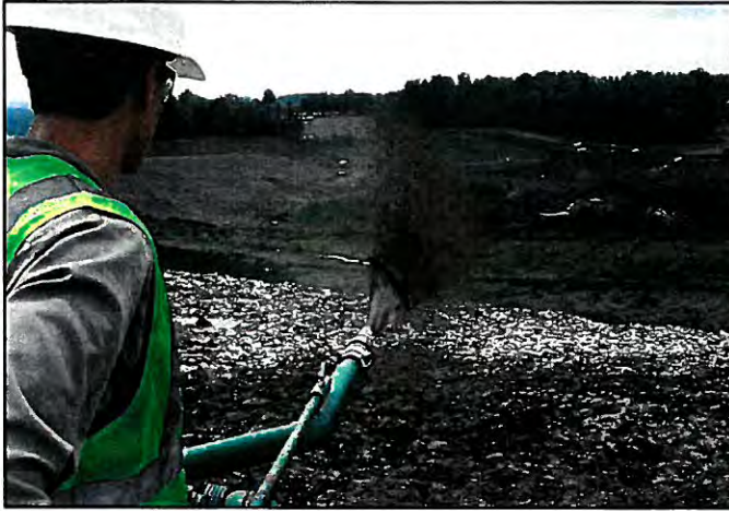
Application of Posi-Shell® via Deck-Mounted Discharge Wand
