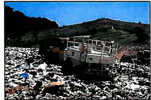
Proper orientation of equipment on slope
