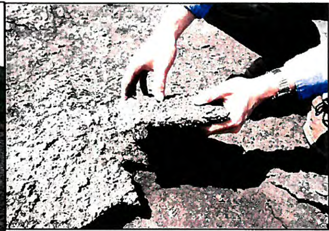
Cured Long-Term Posi-Shell® Coating
