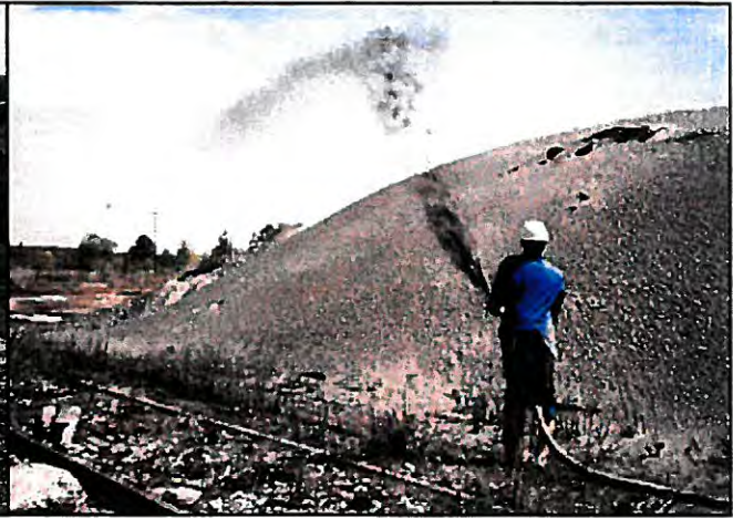
Application of Posi-Shell® via Extension Hose
