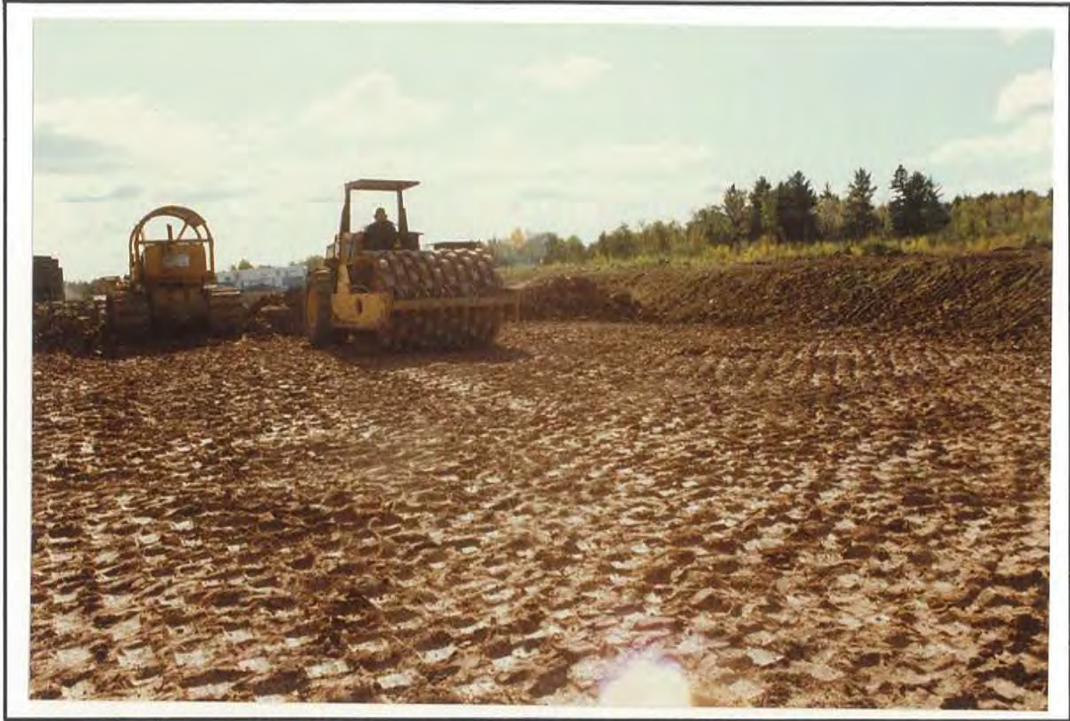
PHOTO 7 CLAY BARRIER SOIL CONSTRUCTION
