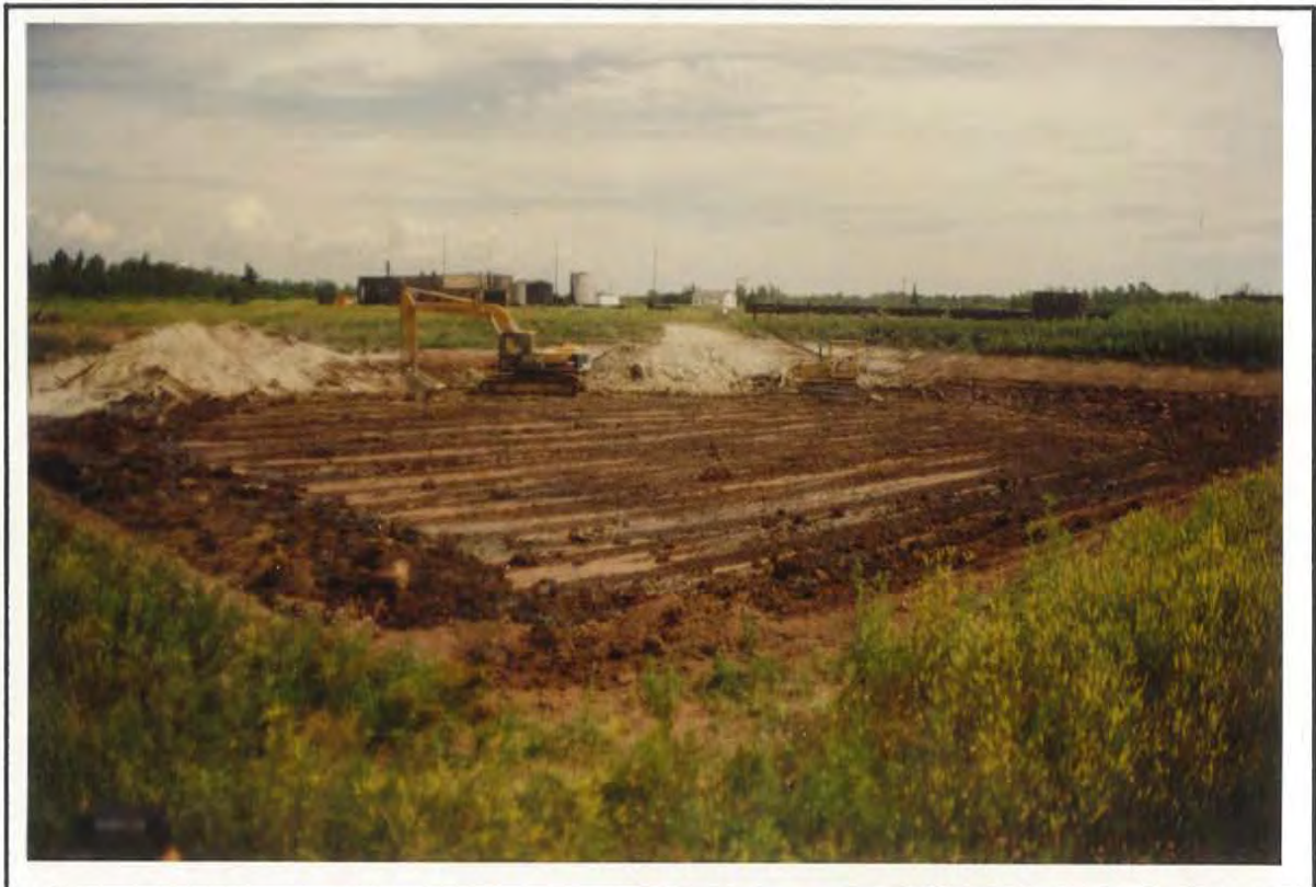
PHOTO 6 PUSHING SLUDGE TO ADMIXTURE PILES
