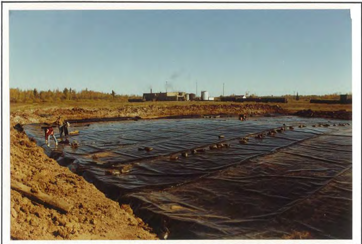
PHOTO 14 LAST LINER PANELS PLACED ON NORTHERN END OF CAP
