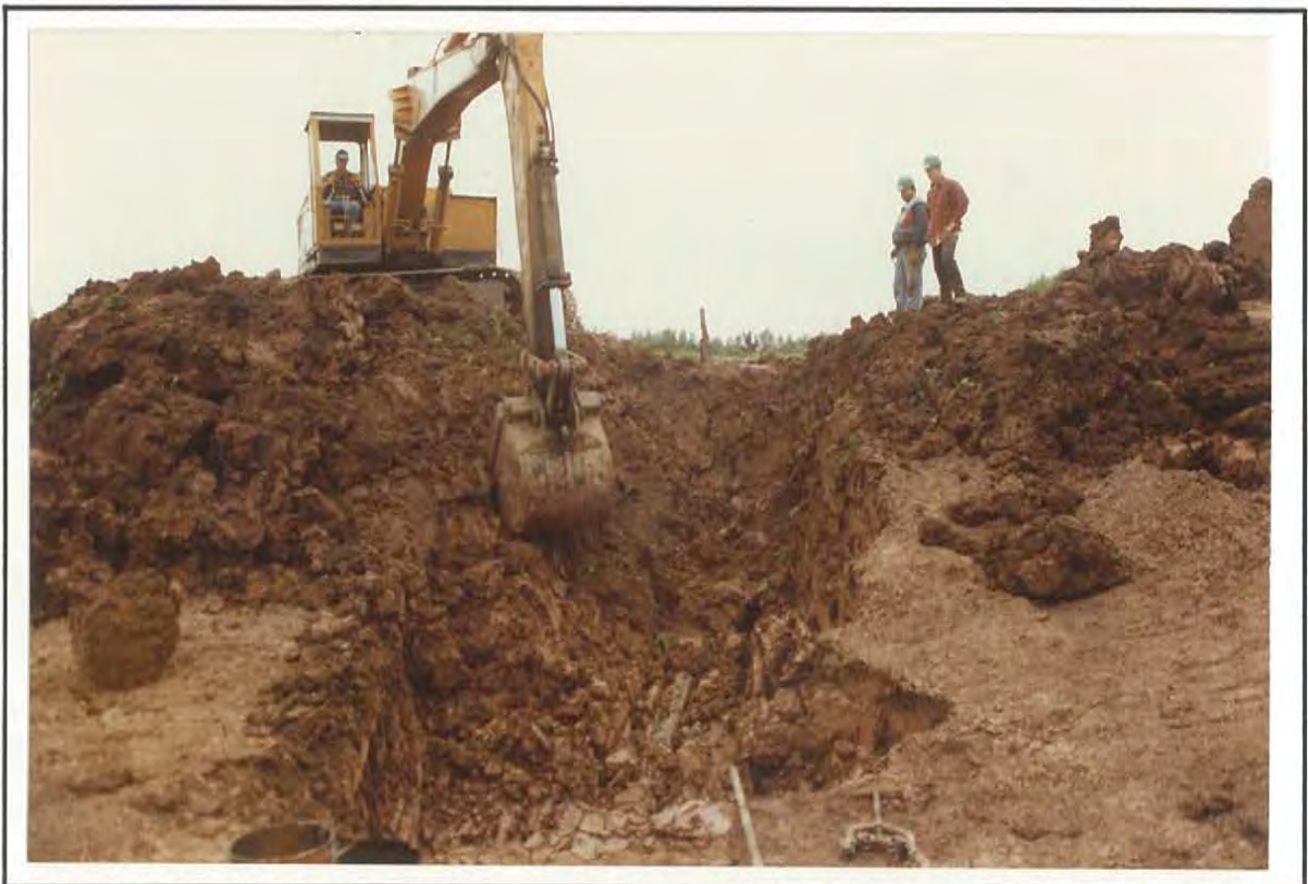
PHOTO 2 REMOVING BURIED PIPES
