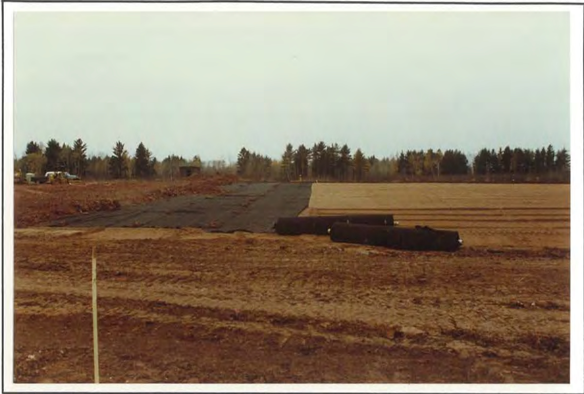
PHOTO 21 DRAINAGE LAYER MATERIAL WITH GEOTEXTILE
