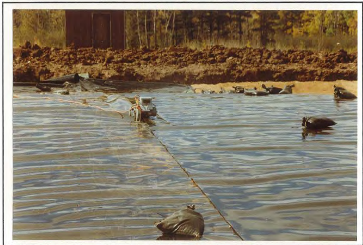
PHOTO 16 FUSION WELDING OF THE LINER
