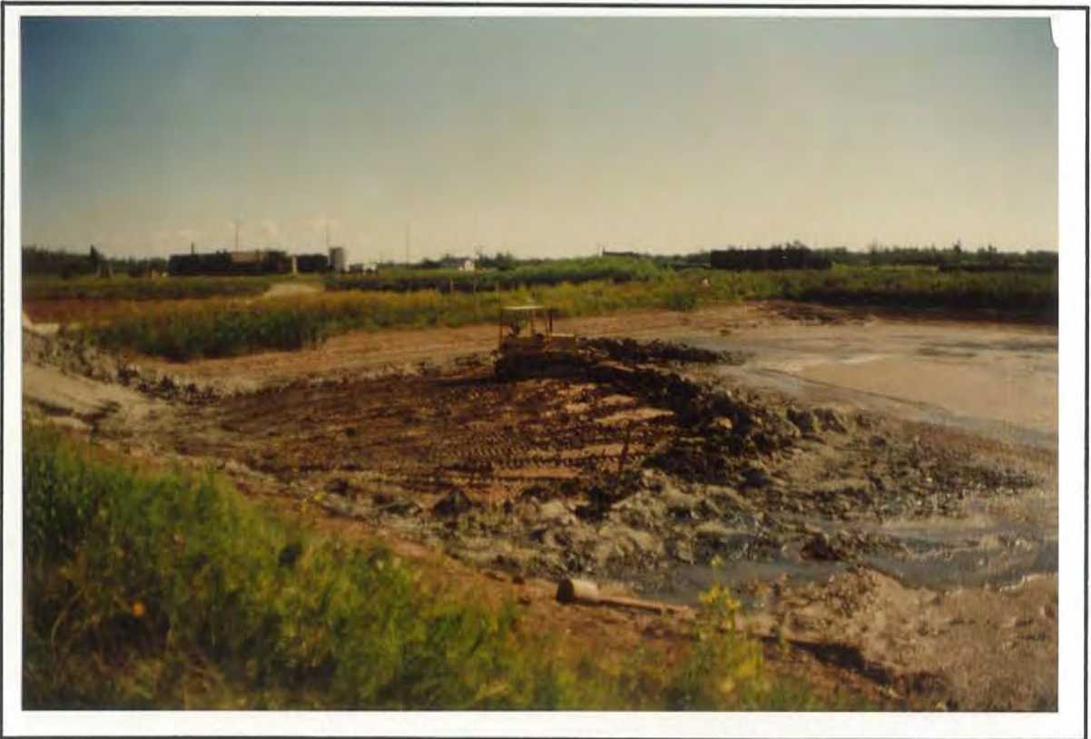
PHOTO 12 PUSHING SLUDGE SOUTH AND EAST
