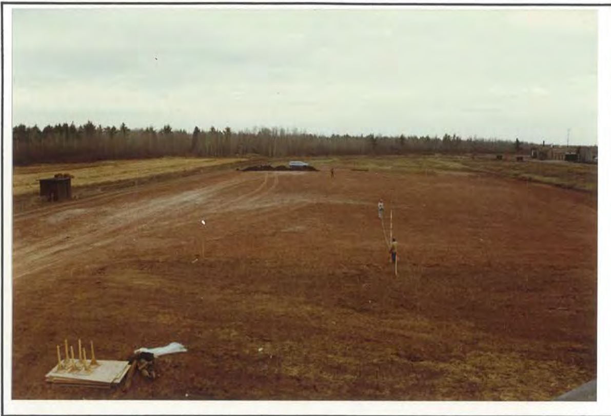
PHOTO 23 CHECKING ELEVATIONS OF UNCLASSIFIED SOIL FILL
