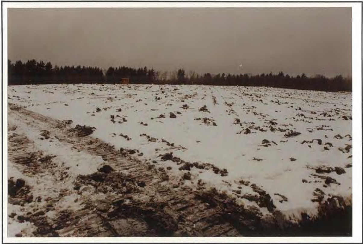
PHOTO 25 SNOW COVERED TOPSOIL END OF CONSTRUCTION FOR 1988
