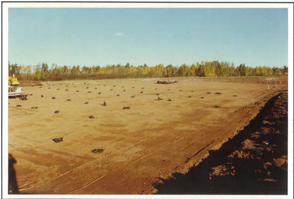
PHOTO 10 SAND CUSHION AND ANCHOR TRENCH ALONG EAST EDGE OF CAP
