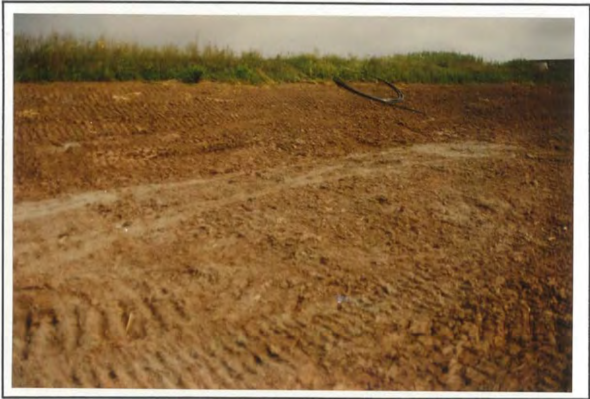
PHOTO 17 LAGOON BOTTOM AFTER CLEANUP
