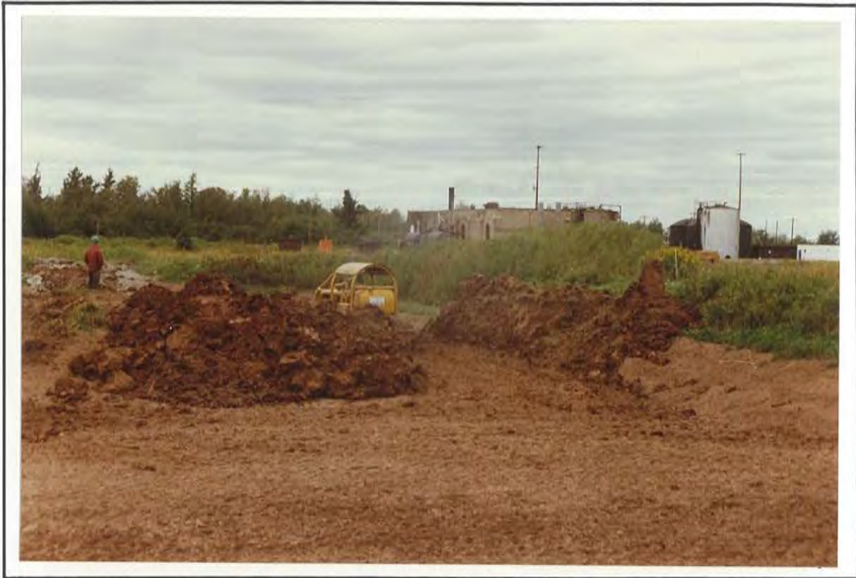
PHOTO 3 EXCAVATING CENTER DIKE
