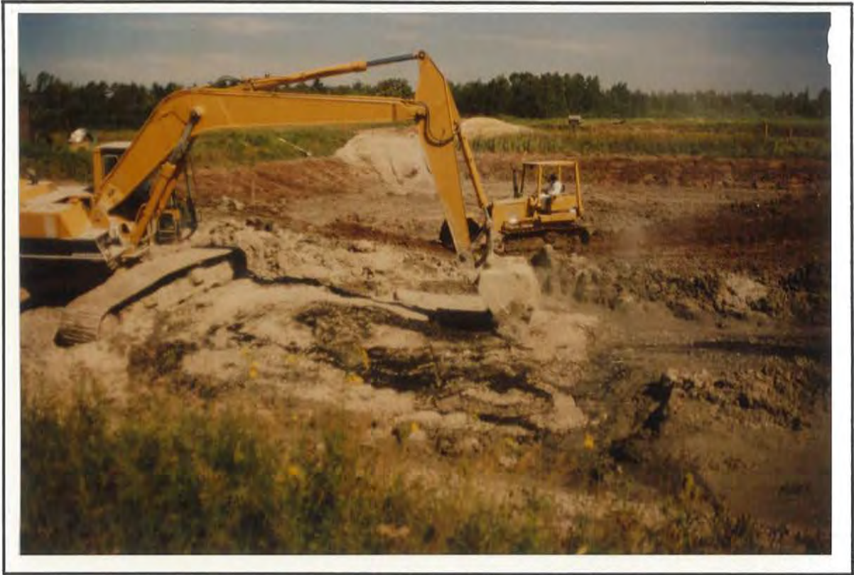
PHOTO 7 MIXING SLUDGE WITH ADMIXTURE
