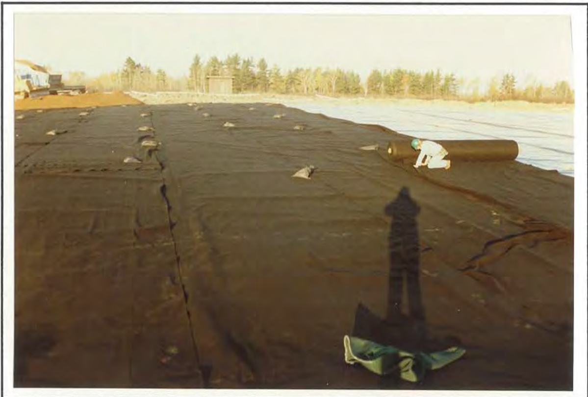
PHOTO 18 GEOTEXTILE (FILTER FABRIC) PLACEMENT
