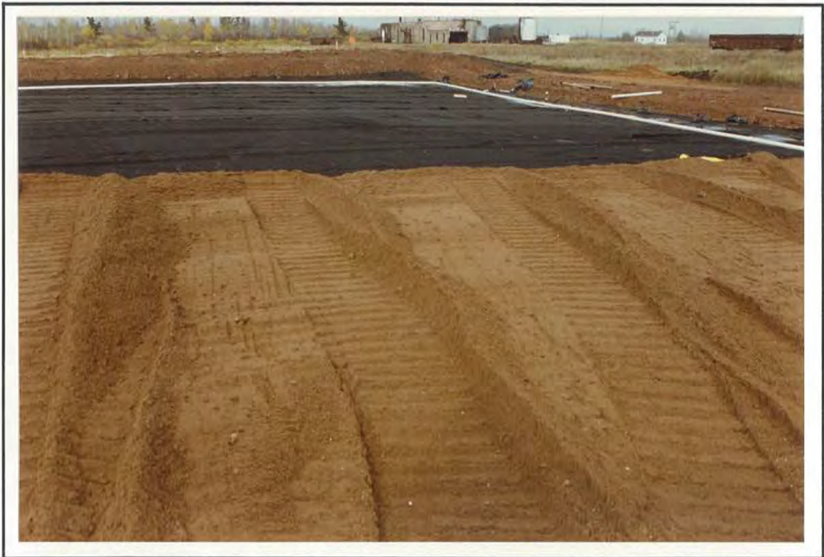
PHOTO 20 DRAINAGE LAYER MATERIAL PLACED ON GEOTEXTILE
