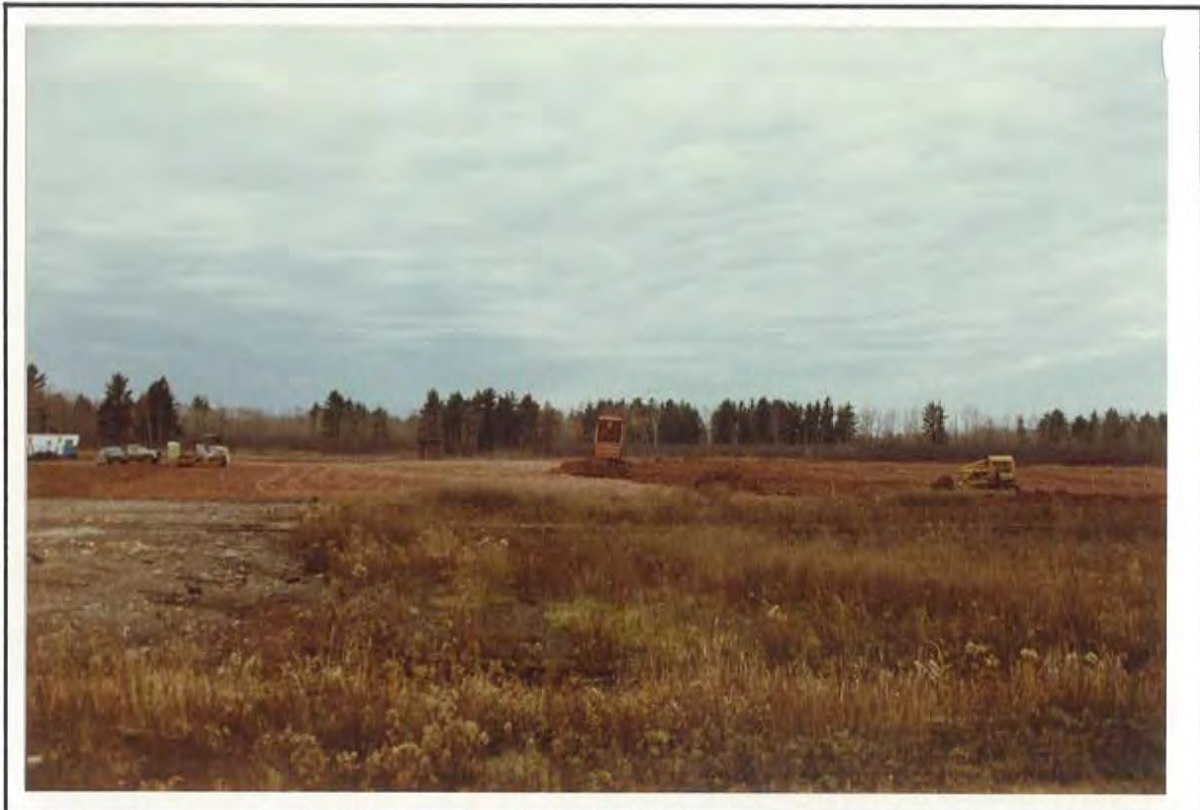
PHOTO 22 PLACING, SPREADING AND COMPACTING THE UNCLASSIFIED FILL
