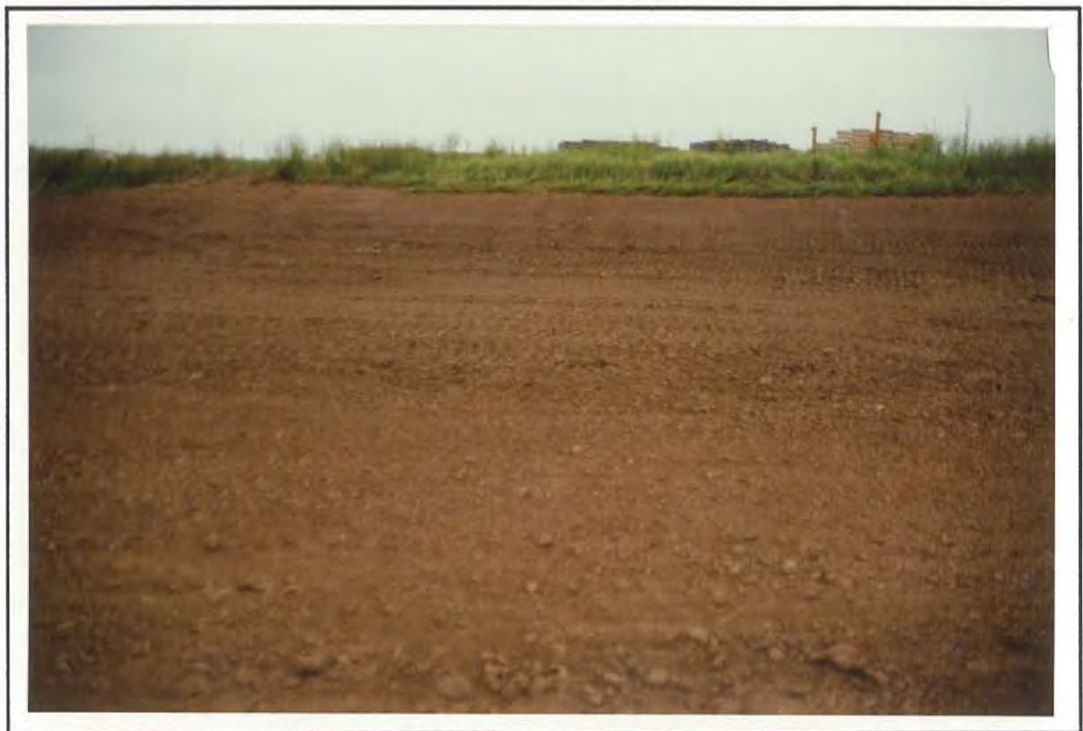
PHOTO 10 FINAL GRADE - ALL SLUDGE REMOVED
