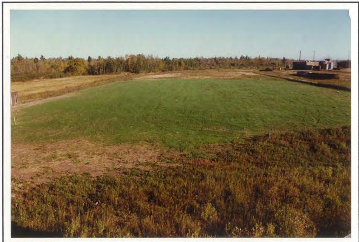
PHOTO 26 OVERVIEW OF COMPLETED CAP (LOOKING NORTH)
