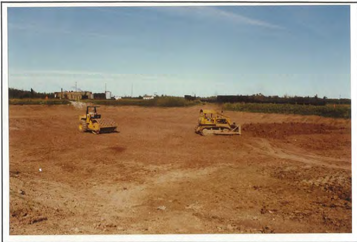
PHOTO 5 SPREADING AND COMPACTING UNCLASSIFIED SOIL FILL
