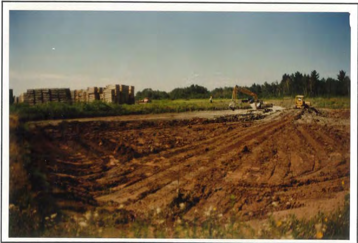
PHOTO 16 PUSHING SLUDGE TO BACKHOE
