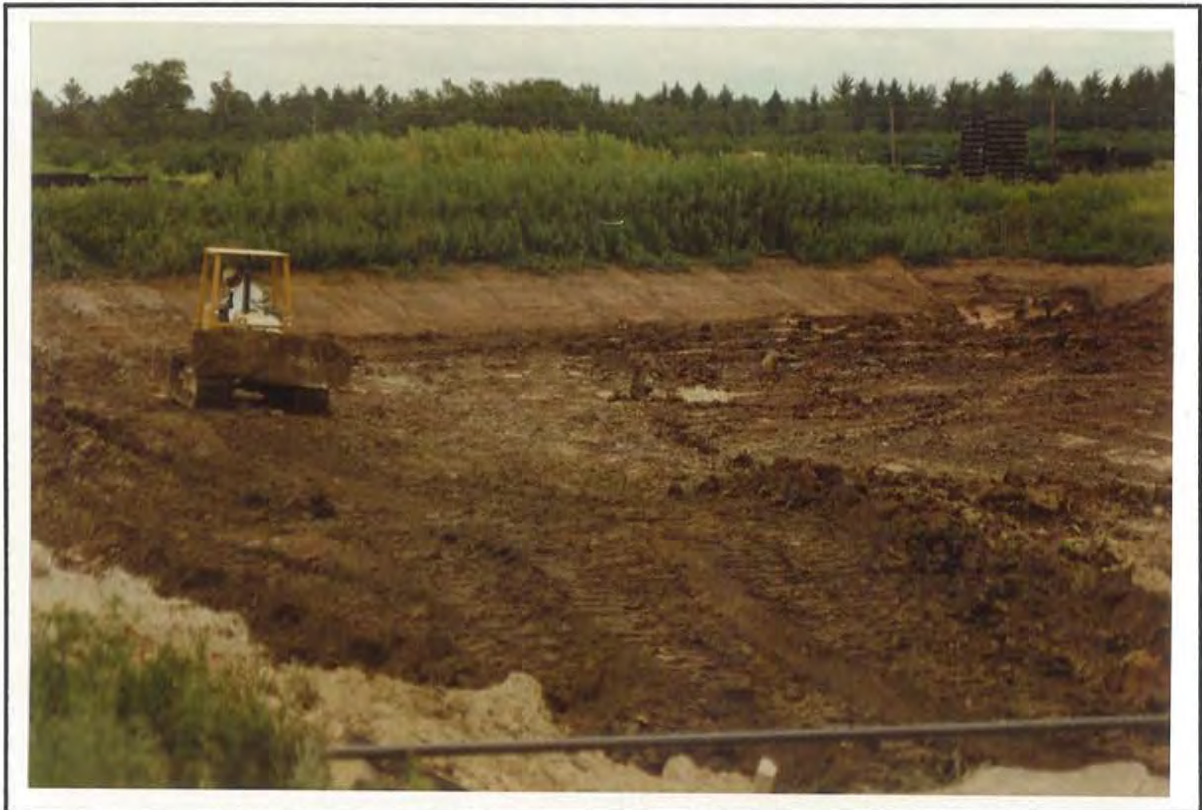
PHOTO 8 CLEANING BOTTOM TO FINAL GRADE
