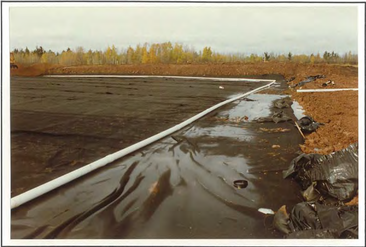
PHOTO 19 DRAINAGE PIPE PLACEMENT
