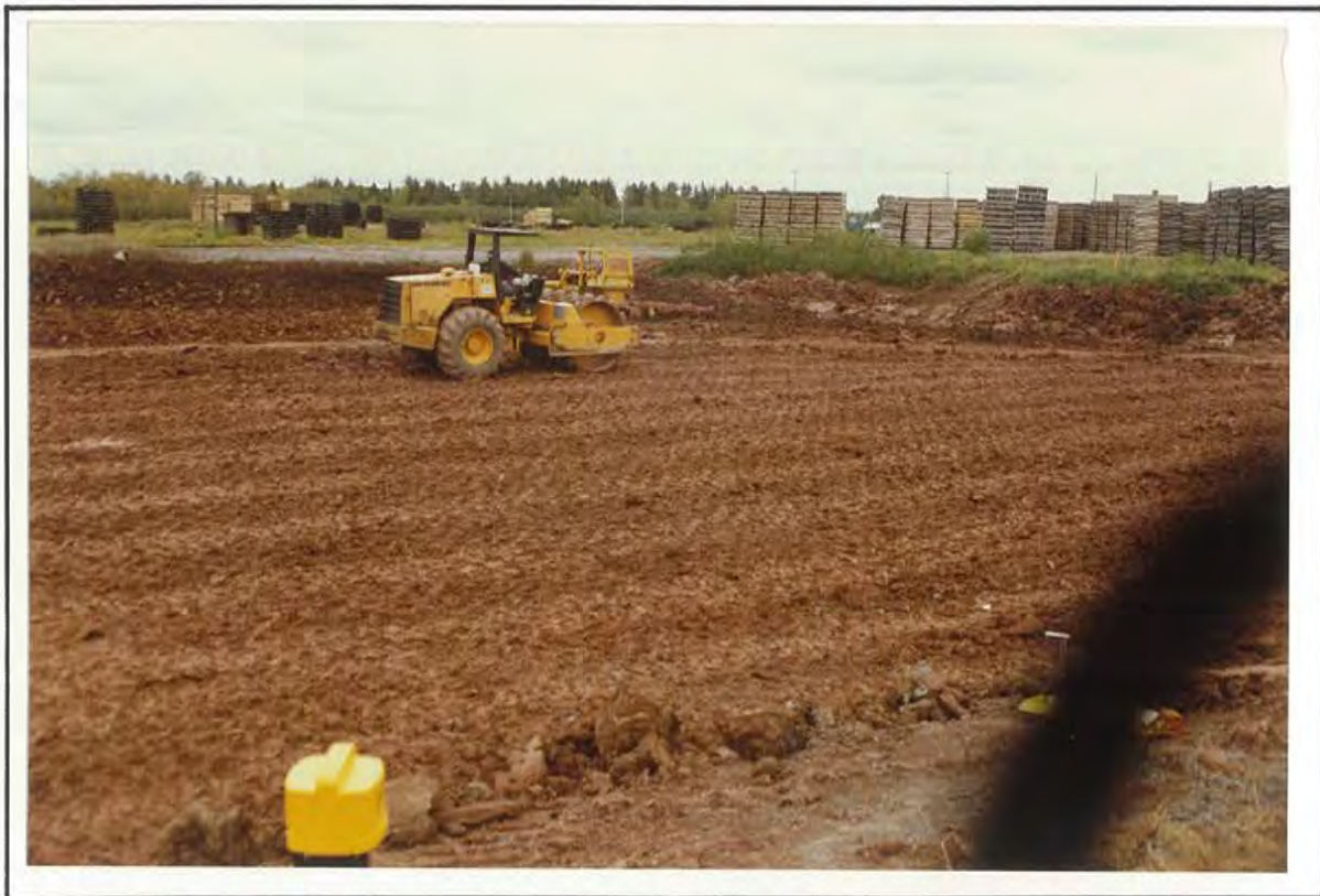
PHOTO 4 FIRST LAYER OF UNCLASSIFIED SOIL FILL
