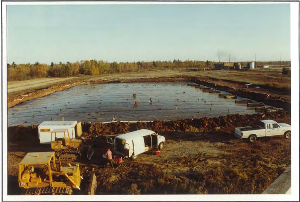
PHOTO 15 COMPLETED LINER INSTALLATION
