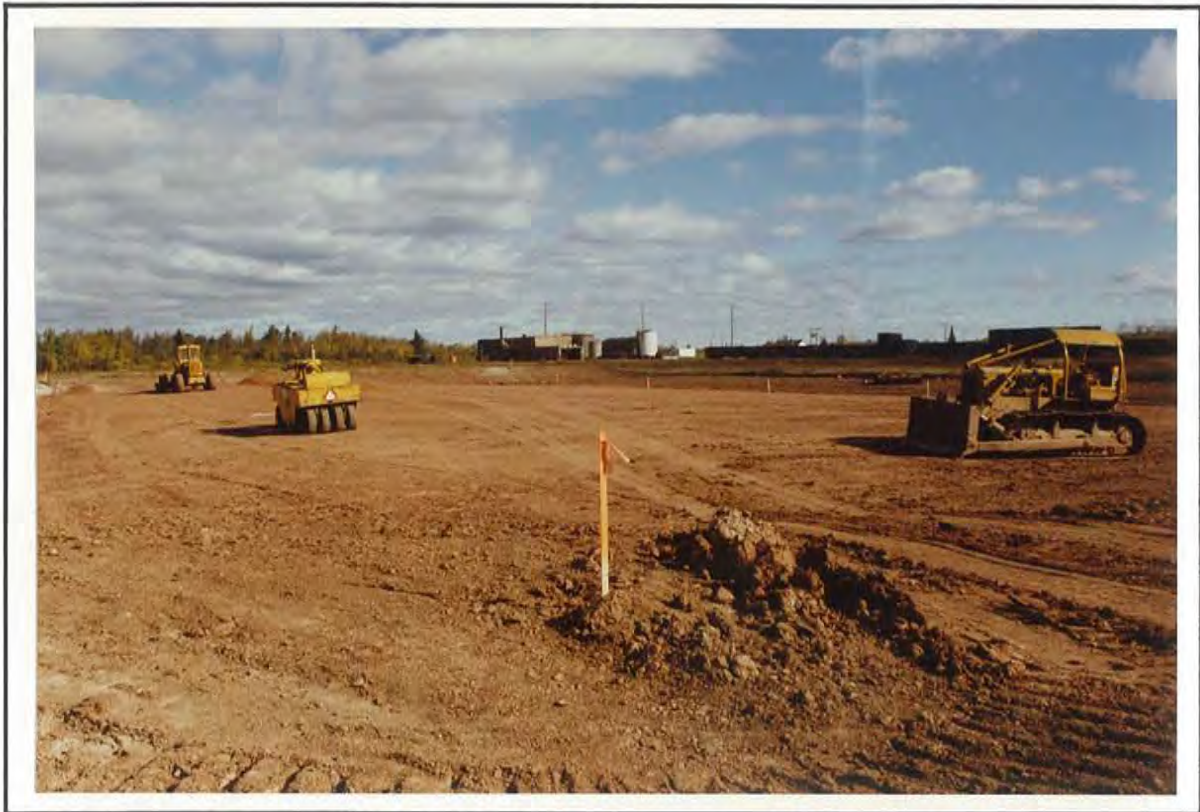
PHOTO 8 FINAL GRADING AND COMPACTING CLAY BARRIER SOIL
