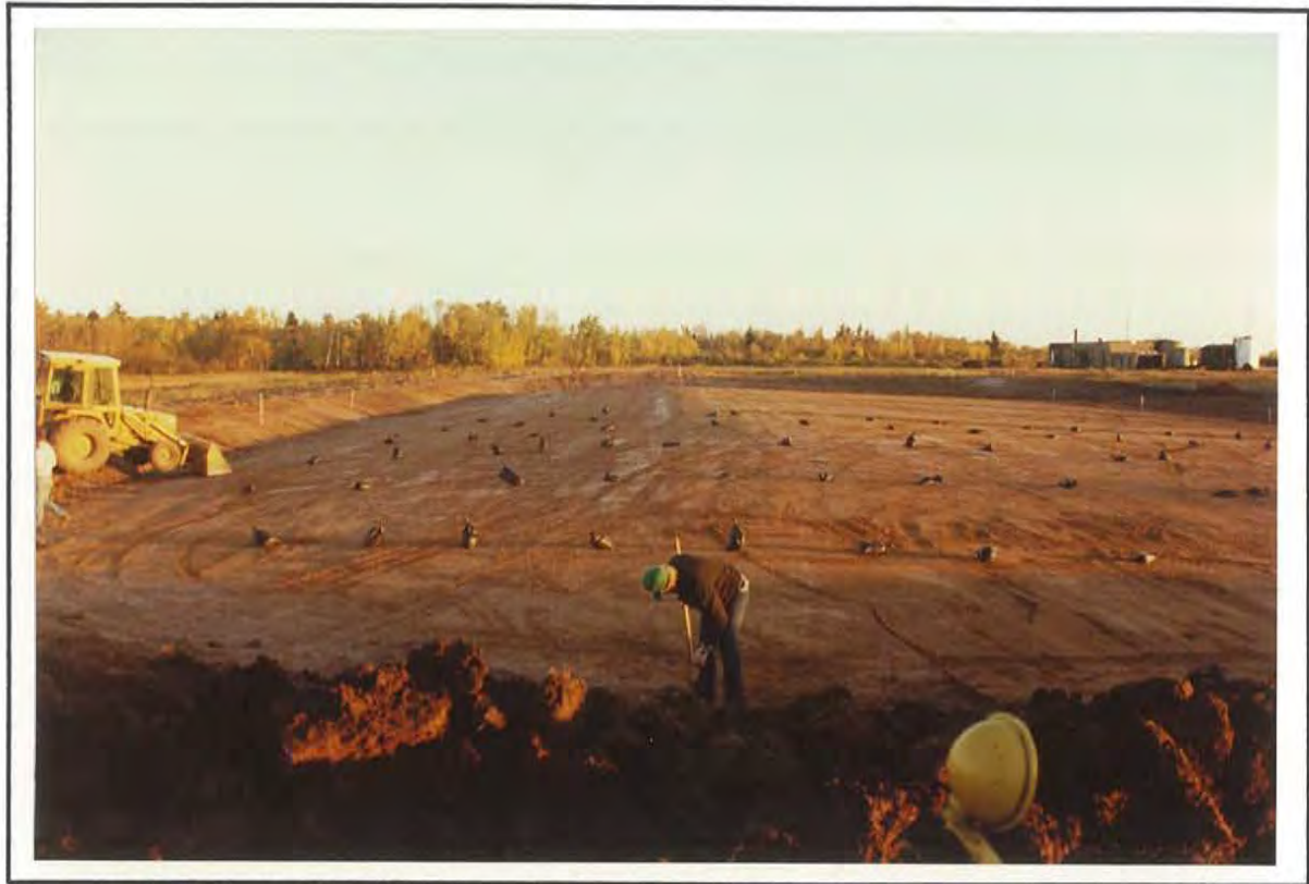
PHOTO 9 SAND CUSHION AND ANCHOR TRENCH ALONG WEST EDGE OF CAP
