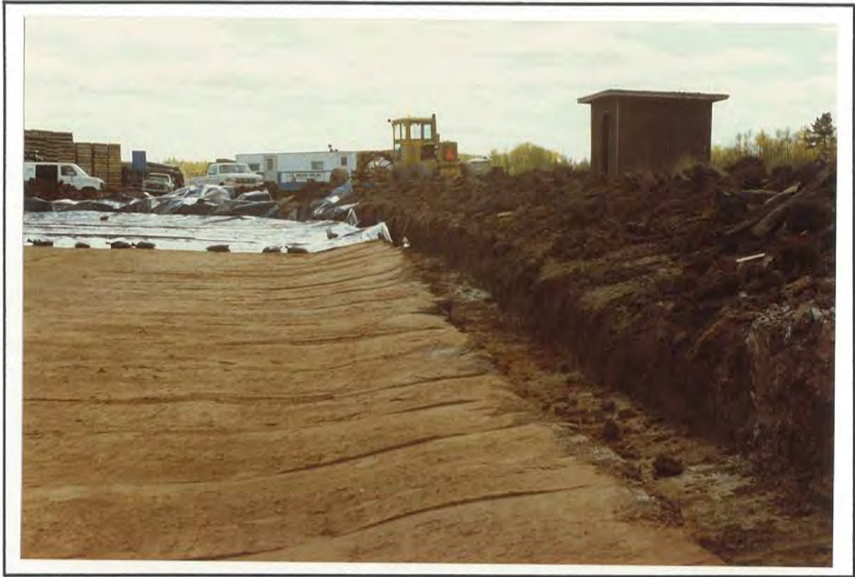
PHOTO 13 LINER PLACED ON SAND CUSHION AND IN ANCHOR TRENCH
