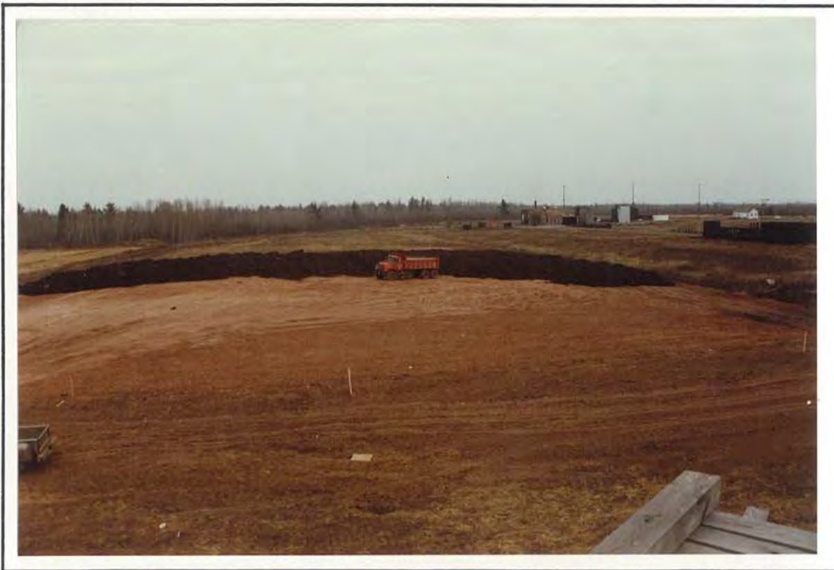
PHOTO 24 PLACING TOPSOIL LAYER
