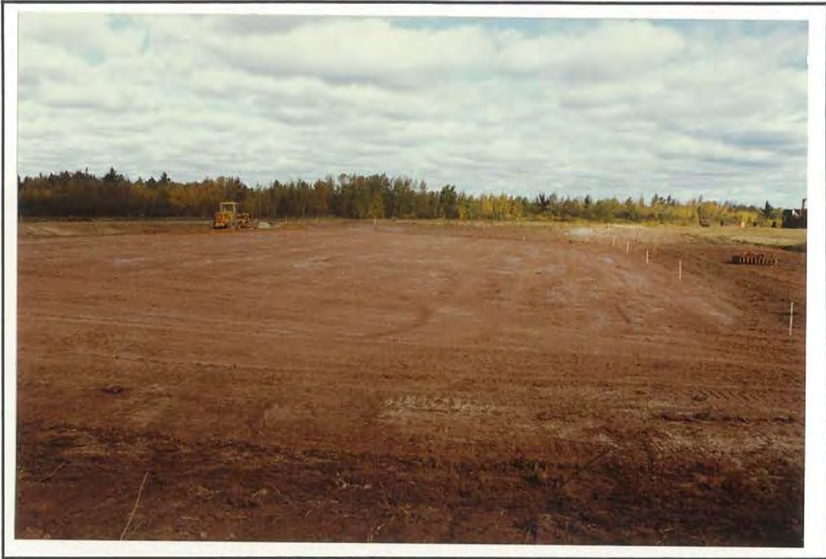
PHOTO 11 SPREADING SAND CUSHION SOIL
