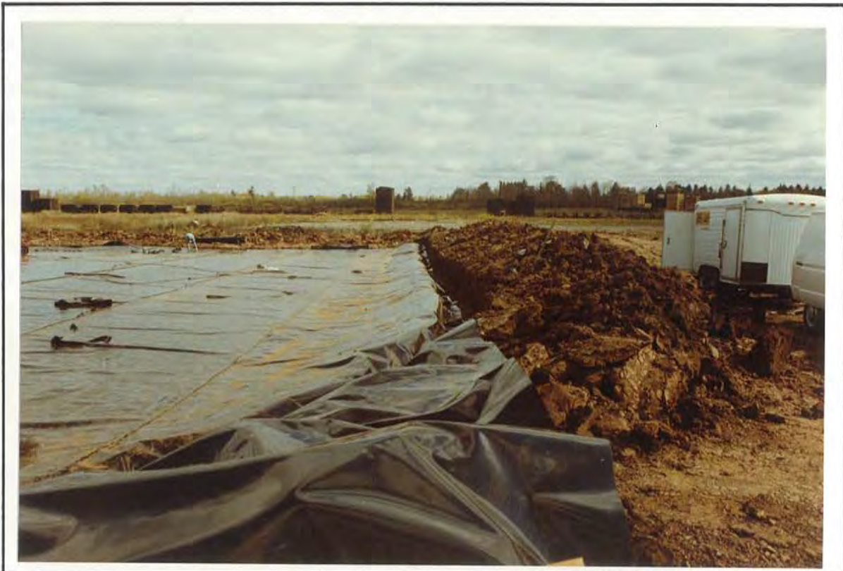
PHOTO 12 HDPE LINER IN PLACE ALONG SOUTH EDGE OF CAP
