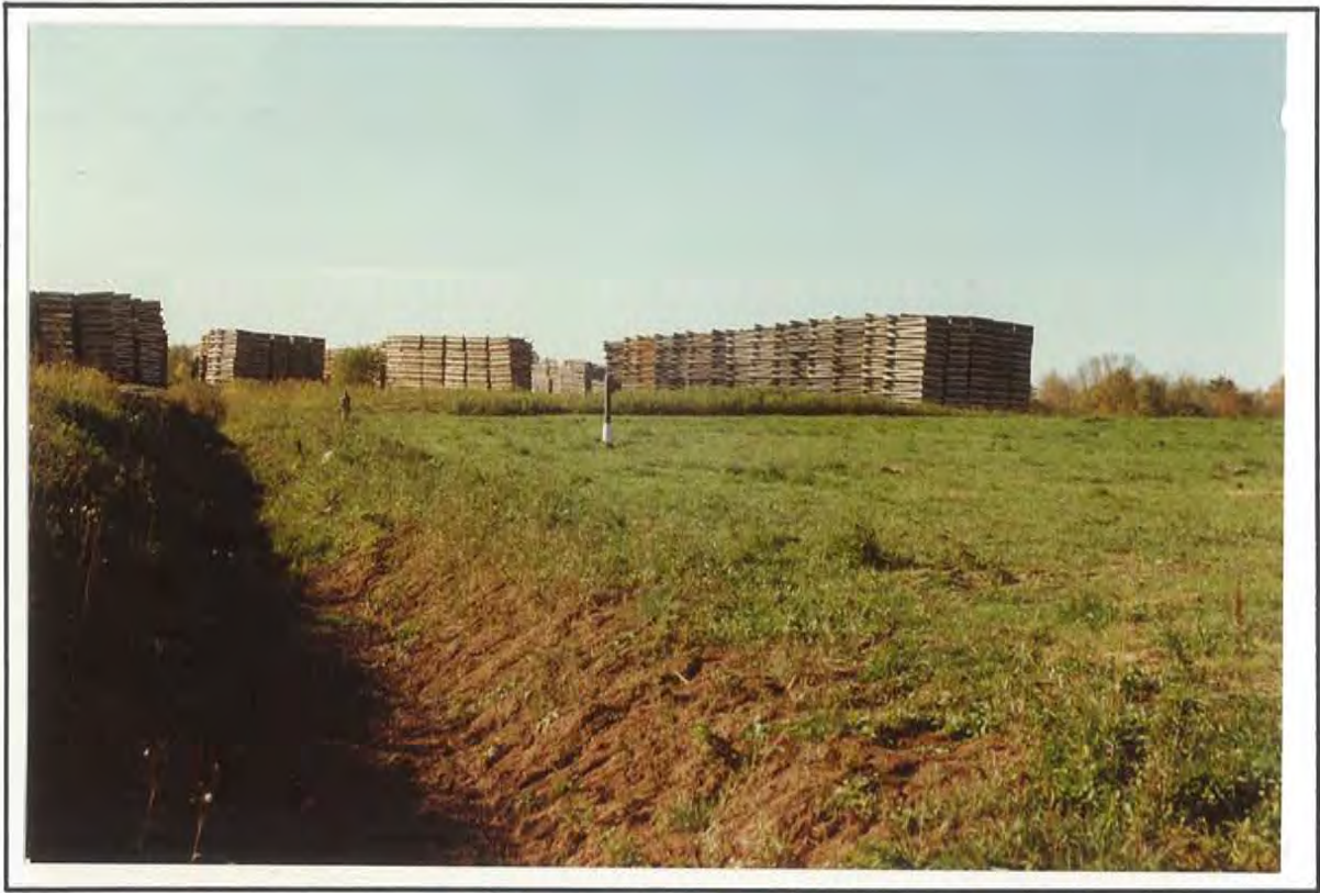
PHOTO 29 DRAINAGE CHANNEL AT WEST CAP EDGE (LOOKING SOUTH)
