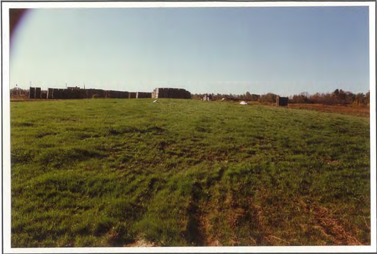
PHOTO 27 COMPLETED CAP (LOOKING SOUTH)
