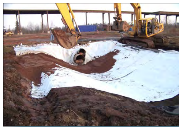
3 GENERAL FILL IS PLACED OVER RCM PRIOR TO GEOTEXTILE & RIP RAP.
