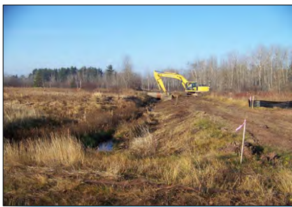
1 SLOPES IN OUTFALL DITCH ARE PREPARED FOR CONSTRUCTION.
