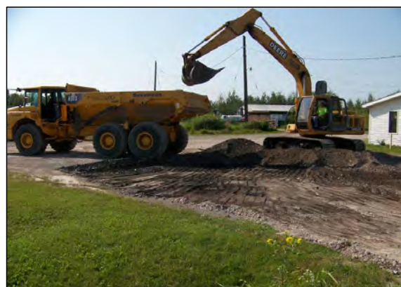
3 CONSTRUCTION ENTRANCES ARE INSTALLED.
