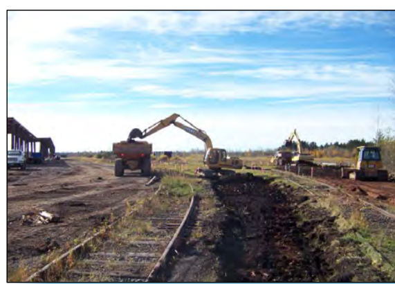
3 CUT / FILL OPERATIONS IN AREA B CONTINUE.
