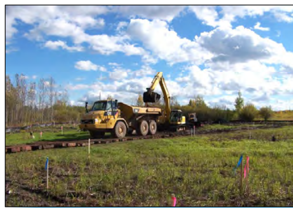
3 SOIL REMOVAL ACTIVITIES IN AREA B.
