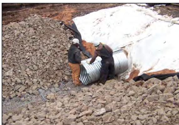
4 CREW EXTENDS CULVERT ON WEST SIDE OF RR CROSSING.
