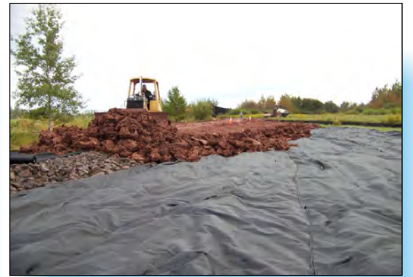
3 CONTINUING TO PLACE CLAY BACKFILL IN AREA S2.
