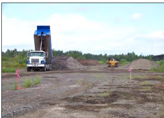
4 MATERIALS FOR PROJECT ARE DELIVERED TO SITE AND STOCKPILED.
