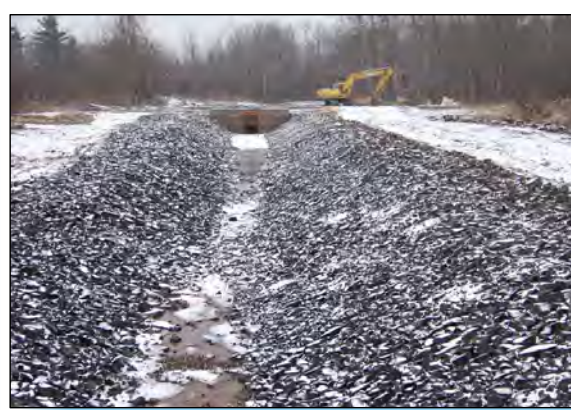
3 A VIEW COMPLETED OF OUTFALL DITCH LOOKING WEST "UPSTREAM SECTION".
