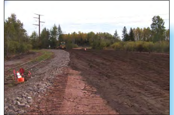
6 TOPSOIL PLACEMENT IN AREA G IS COMPLETED.
