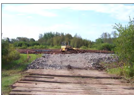
1 CLAY BACKFILL CONTINUES TO BE PLACED IN AREA H.
