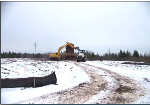
1 COMPACTING SUBGRADE IN AREA A; IN PREPARATION FOR AREA A COVER.
