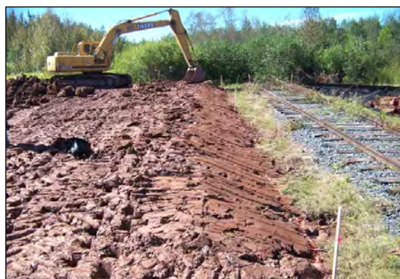
5 INSTALLING SLOPE ALONG TRACKS IN AREA H.
