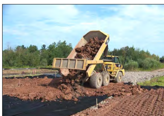
2 CLAY BACKFILL CONTINUES TO BE PLACED IN AREA H.
