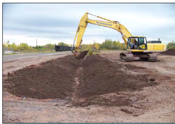
2 TOPSOIL IS PLACED IN F1 DITCH IN PREPARATION FOR SEEDING.
