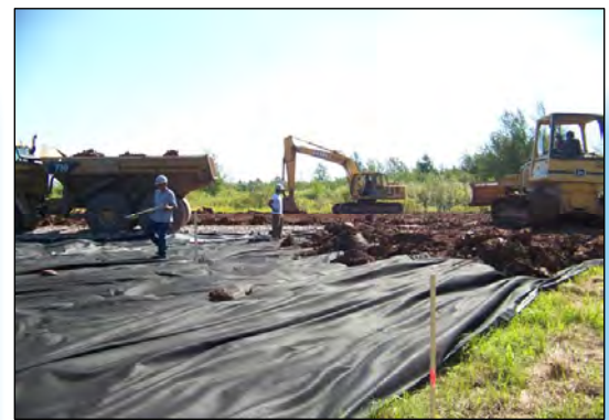
6 CONTINUING TO PLACE CLAY BACKFILL IN AREA H.
