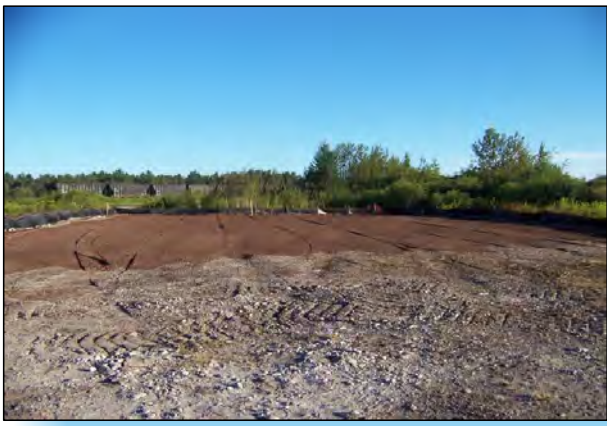
1 AREA F2 CAPPING IS COMPLETED MONDAY 8-16-2010.
