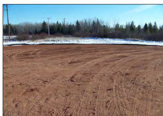
3 AREA A COVER IS COMPLETED.
