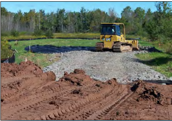
1 STONE IS PLACED FOR ACCESS BETWEEN AREAS S1 & S2.
