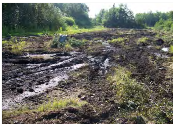
5 AREA G AFTER CLEARING.
