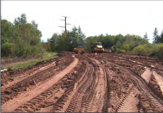
4 PLACEMENT OF CLAY BACKFILL CONTINUES IN AREA G.
