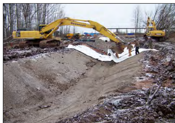
6 CREW DEPLOYS RCM IN OUTFALL DITCH.
