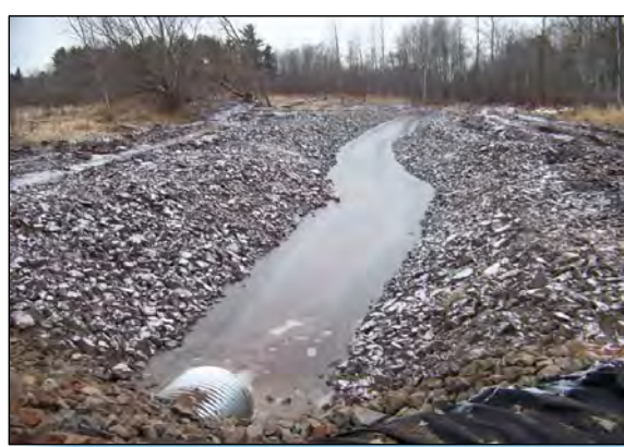
2 A VIEW OF COMPLETED OUTFALL LOOKING WEST "DOWNSTREAM SECTION".
