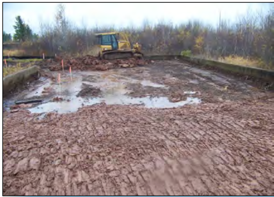
1 CLAY BACKFILL IS PLACED INSIDE CONCRETE BASIN IN AREA B.
