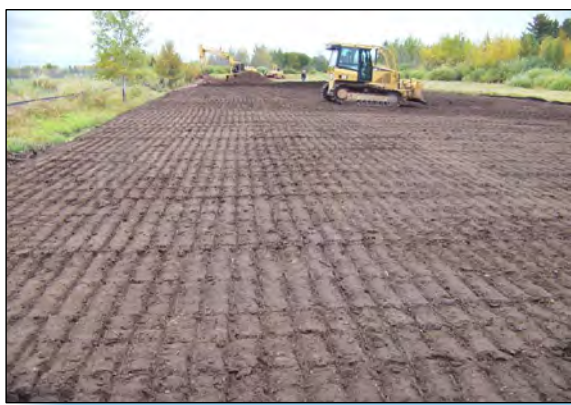
1 TOPSOIL PLACEMENT IN AREAS S1 & S2.
