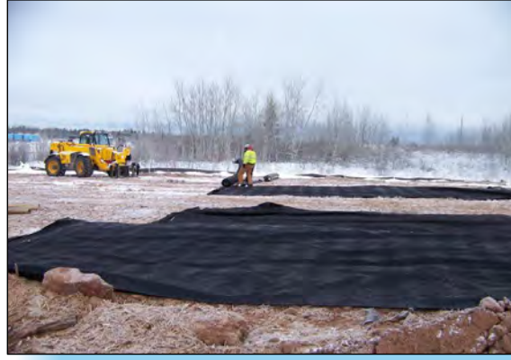
5 CREW DEPLOYS GEOTEXTILE PRIOR TO FILL PLACEMENT.
