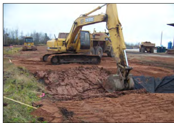
6 BACKFILL IS PLACED IN AREA B.
