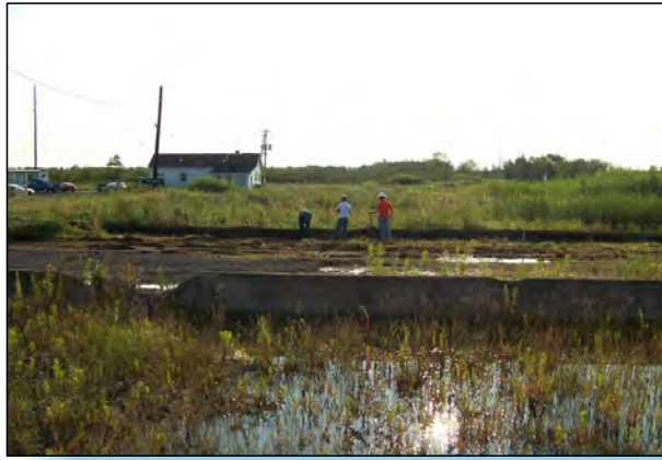
5 INSTALLATION OF EROSION CONTROLS CONTINUES THIS WEEK.
