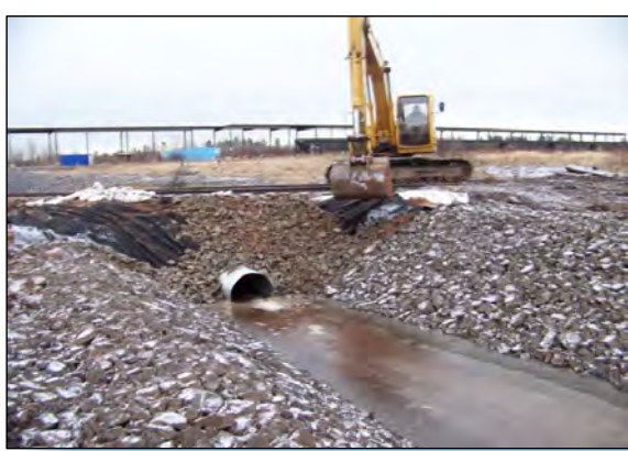
1 RIP RAP IS PLACED AT HEADWALL IN OUTFALL DITCH.
