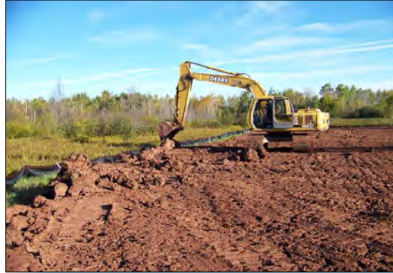
5 EXCAVATOR IS USED TO INSTALL SLOPE IN AREA S2.
