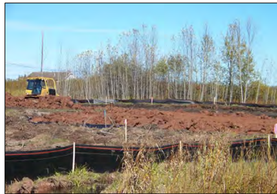
6 PLACING CLAY BACKFILL IN AREA B.
