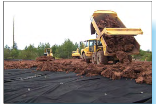
3 CLAY BACKFILL PLACEMENT CONTINUES IN AREA G.
