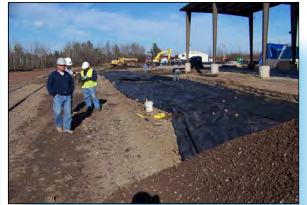
3 INSTALLATION OF ROAD BASE SURFACE COVER IN AREA B.
