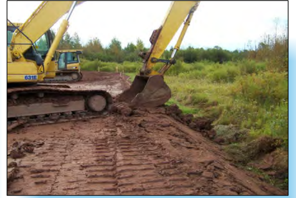
6 SLOPE IS INSTALLED ON EAST SIDE OF AREA H.
