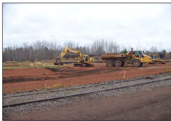
5 BACKFILL IS PLACED IN AREA B.
