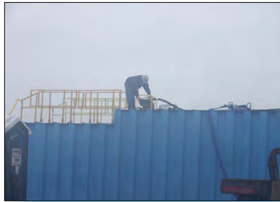
2 CREW CONTINUES TO TREAT WATER.
