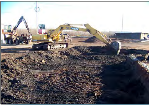
1 SUBGRADING OPERATIONS CONTINUE IN AREA B.
