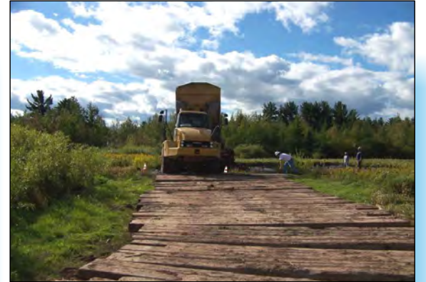
6 CLAY BACKFILL IS PLACED IN AREA S1.
