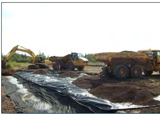
1 BACKFILLING ROAD BASE AND CLAY BACKFILL IN AREA F1.
