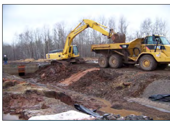
2 OUTFALL DITCH EXCAVATION CONTINUES.
