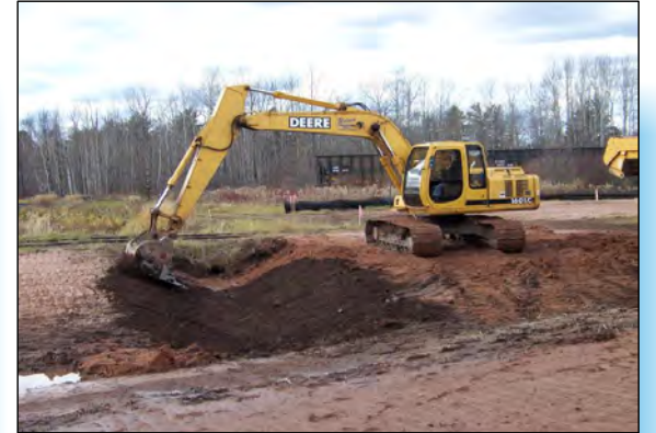
6 INSTALLATION OF CLAY VEGETATED SURFACE COVER IN AREA B.
