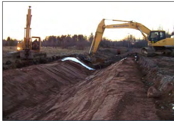
5 GENERAL FILL IS PLACED OVER RCM PRIOR TO GEOTEXTILE & RIP RAP.
