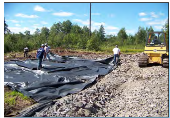
3 WOVEN GEOTEXTILE IS PLACED IN AREA G PRIOR TO STONE.
