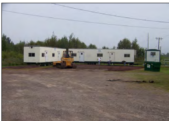
1 PARKING AREA IS INSTALLED.
