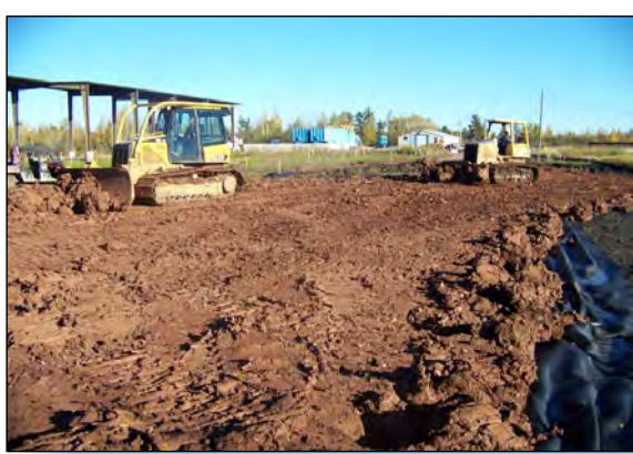
1 SURFACE COVER INSTALLATION IN AREA B.
