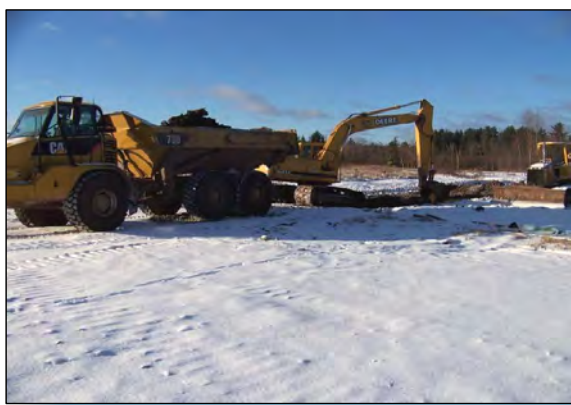
4 EXCAVATION IN AREA B ADJACENT TO OUTFALL DITCH.
