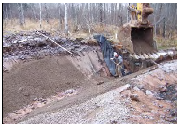
5 OUTFALL DITCH EXCAVATION IS COMPLETED; GRAVEL IS ADDED.
