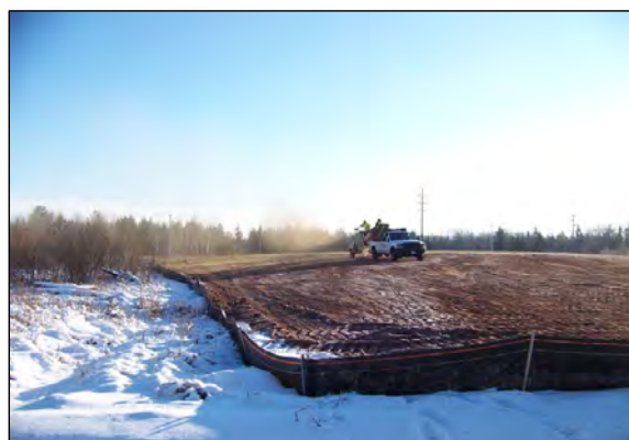
5 STRAW IS PLACED IN AREA A.
