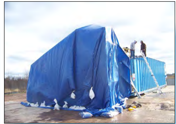
3 CREW CONSTRUCTS SHELTER AROUND WATER TREATMENT SYSTEM.
