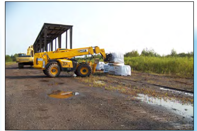
6 CONSTRUCTION MATERIALS CONTINUE TO ARRIVE ON SITE.
