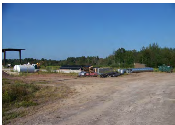
2 MATERIAL FOR PROJECT BEING DELIVERED TO SITE.
