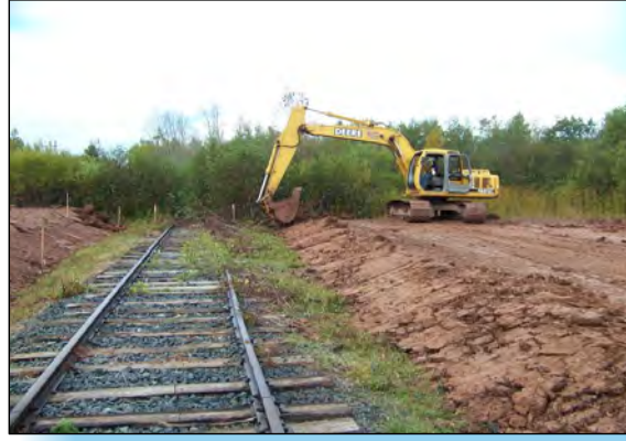
5 SLOPE IS INSTALLED ON WEST SIDE OF AREA H.
