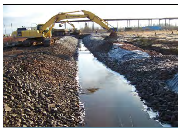
3 RIP RAP PLACEMENT CONTINUES IN OUTFALL DITCH.
