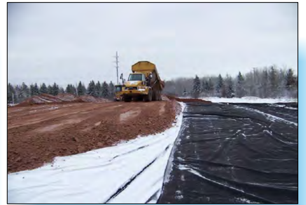
3 GENERAL FILL IS PLACED IN AREA A.
