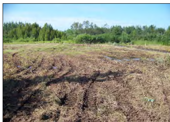
6 AREA H AFTER CLEARING.
