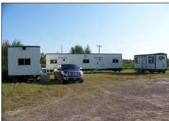
1 OFFICE AREA MOBILIZATION BEGINS.
