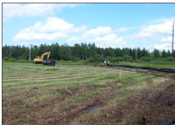
5 CREW INSTALLS SILT FENCE IN WORK AREAS.
