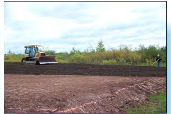
3 TOPSOIL PLACEMENT IN AREA H IS COMPLETED.
