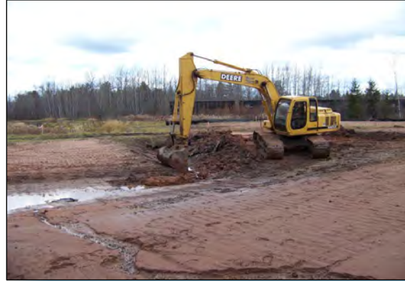
5 INSTALLATION OF CLAY VEGETATED SURFACE COVER IN AREA B.
