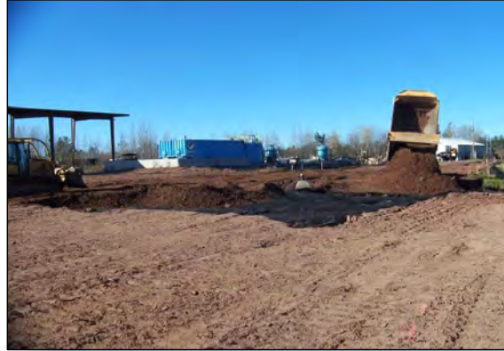
5 CONTINUING TO PLACE GENERAL FILL / CLAY GENERAL FILL IN AREA B.
