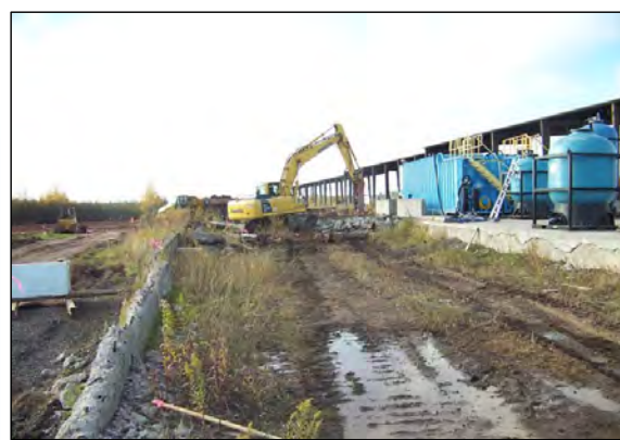
6 DEMOLISHING CONCRETE PIERS AND WALL IN PENTA TANK FARM AREA.
