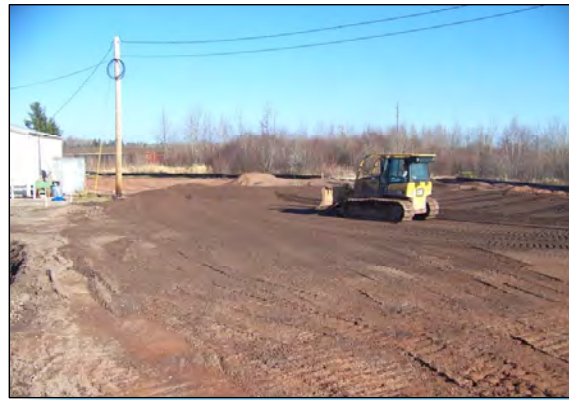
2 SUBGRADING OPERATIONS CONTINUE IN AREA B.
