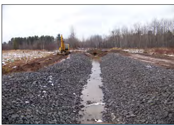
1 A VIEW OF THE OUTFALL DITCH.
