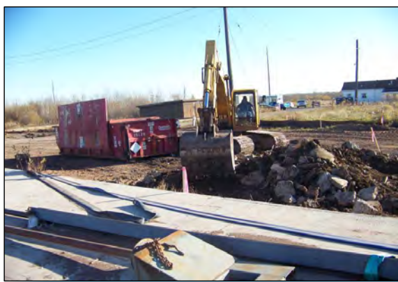
4 PENTA TANK FARM DEBRIS IS LOADED OUT FOR DISPOSAL.
