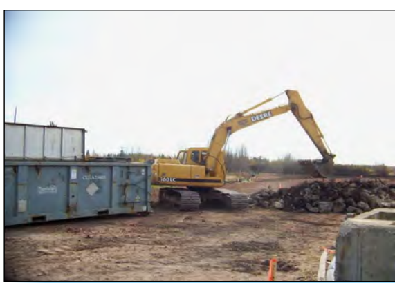
1 DEBRIS FROM PENTA TANK FARM IS LOADED FOR DISPOSAL.
