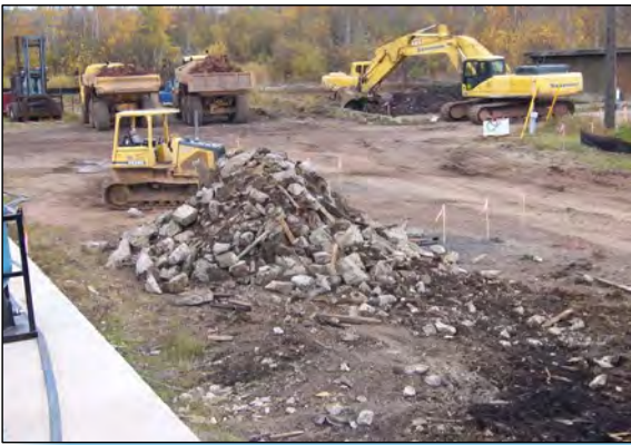
1 CONCRETE FROM PENTA TANK FARM IS DEMOLISHED AND STOCKPILED.
