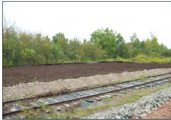
2 TOPSOIL PLACEMENT IS COMPLETED ON THE WESTERN SIDE OF AREA H.
