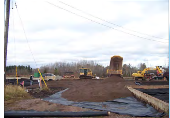
6 INSTALLATION OF ROAD BASE SURFACE COVER IN AREA B.
