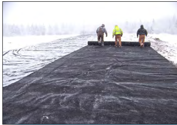
2 GEOTEXTILE IS DEPLOYED PRIOR TO BACKFILL IN AREA A.
