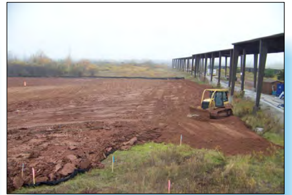
3 GENERAL FILL IS PLACED ALONG DRIP TRACK IN AREA B.
