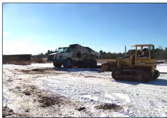
5 BACKFILLING OF EXCAVATION AREA ADJACENT TO OUTFALL DITCH.
