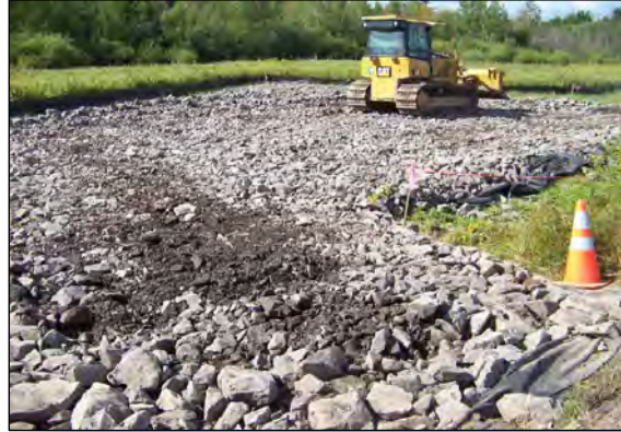
5 STONE BRIDGING IN AREA S1 IS COMPLETED TODAY.
