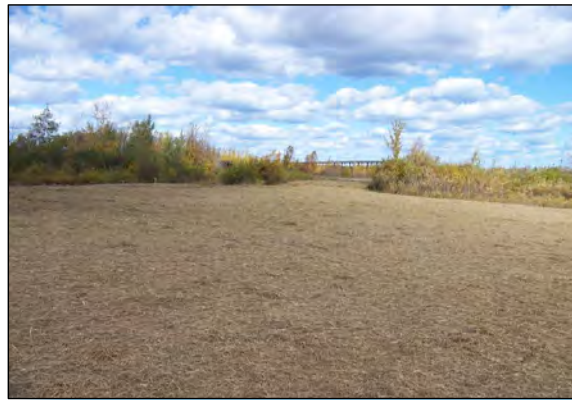
5 AREA G SEEDING COMPLETED.
