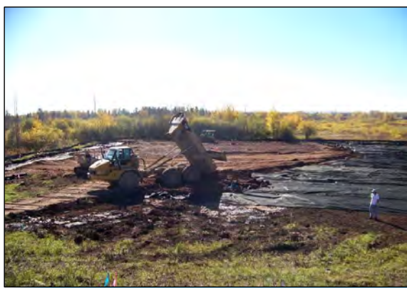
4 SURFACE COVER INSTALLATION IN AREA B.
