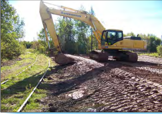
4 SLOPE IS INSTALLED IN AREA G IN PREPARATION FOR TAPER STONE.
