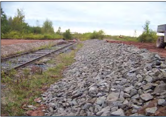
1 A VIEW OF THE STONE PLACED ON THE SLOPE ALONG TRACKS IN AREA H.
