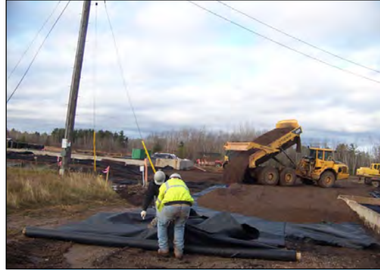
5 INSTALLING OF ROAD BASE SURFACE COVER IN AREA B.
