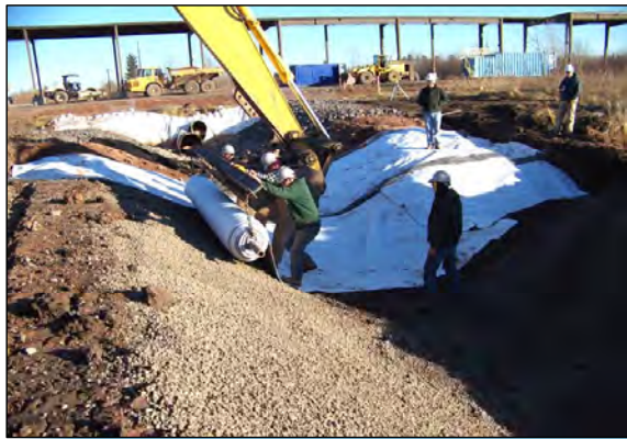
4 RCM IS INSTALLED IN DITCH.
