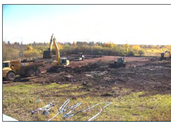
2 SUBGRADE LEVELING IN AREA B.
