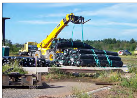
6 REACTIVE CORE MAT IS DELIVERED TO JOBSITE.
