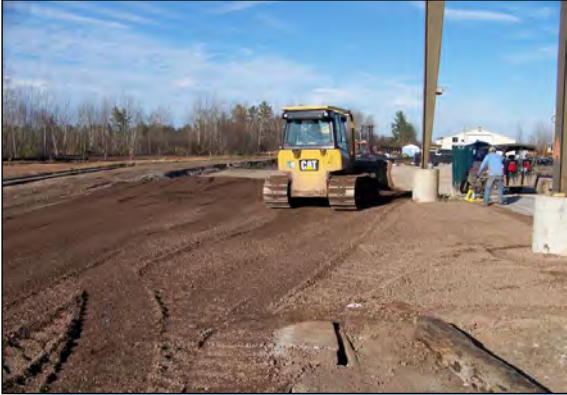
4 INSTALLATION OF ROAD BASE SURFACE COVER IN AREA B.
