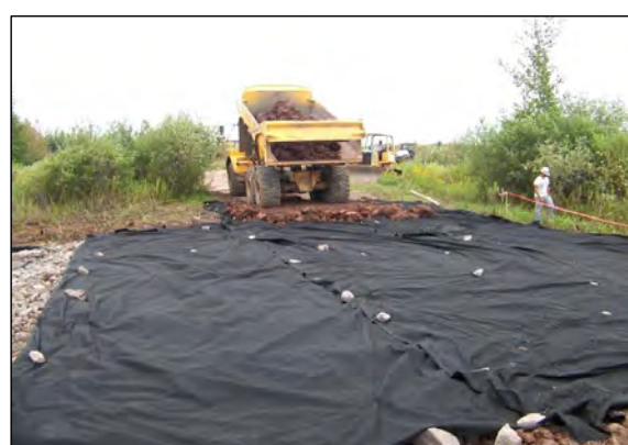
3 CLAY BACKFILL IS PLACED IN AREA H.
