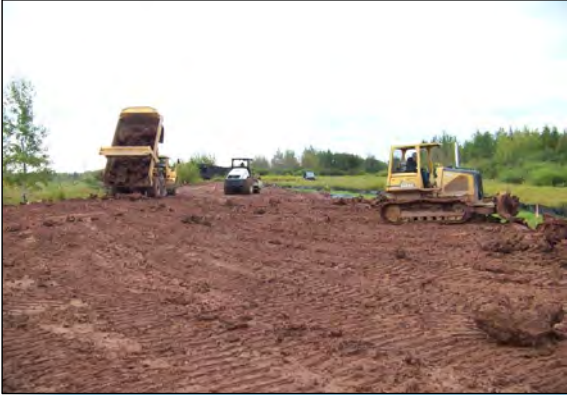
4 CLAY BACKFILL CONTINUES TO BE PLACED IN AREA S2.
