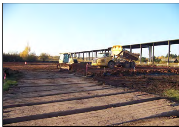
5 SURFACE COVER INSTALLATION IN AREA B.
