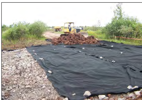
4 CLAY BACKFILL IS PLACED IN AREA H.
