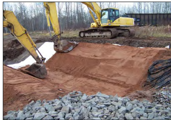
6 GENERAL FILL PLACEMENT.
