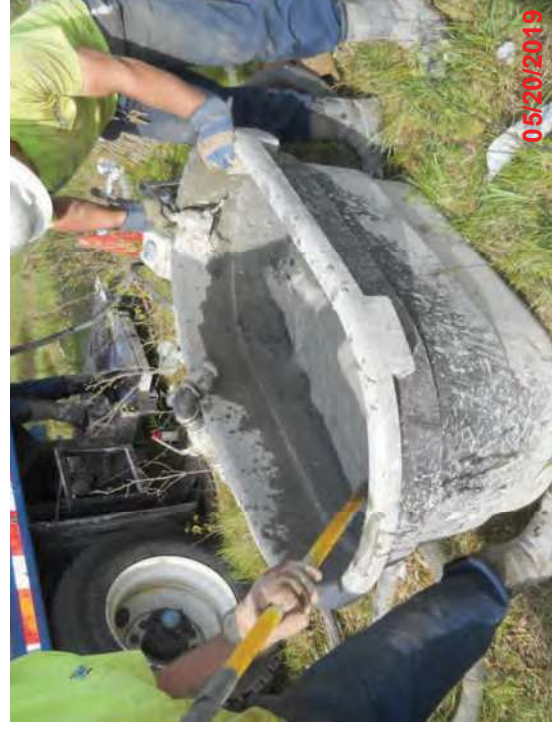
Mixing the bentonite-sand slurry to fill the boreholes
