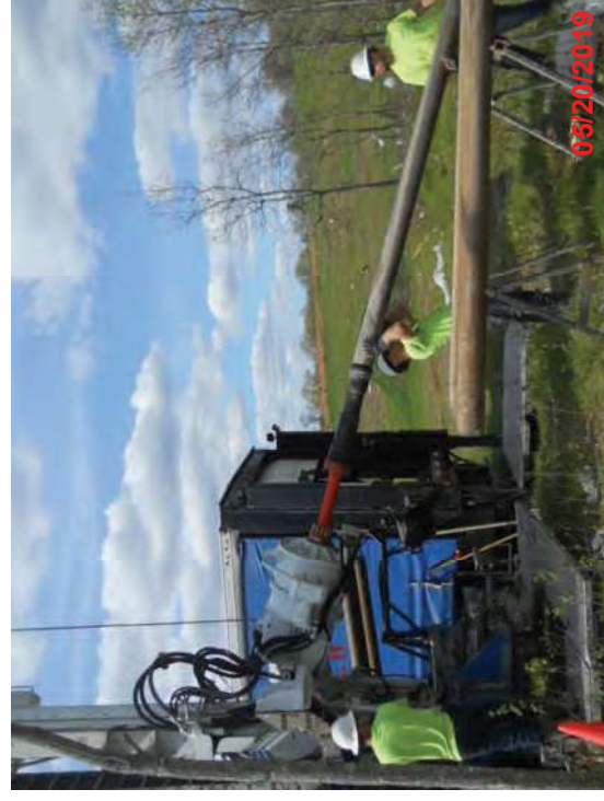
Trut Companies performing Rotary Sonic drilling
