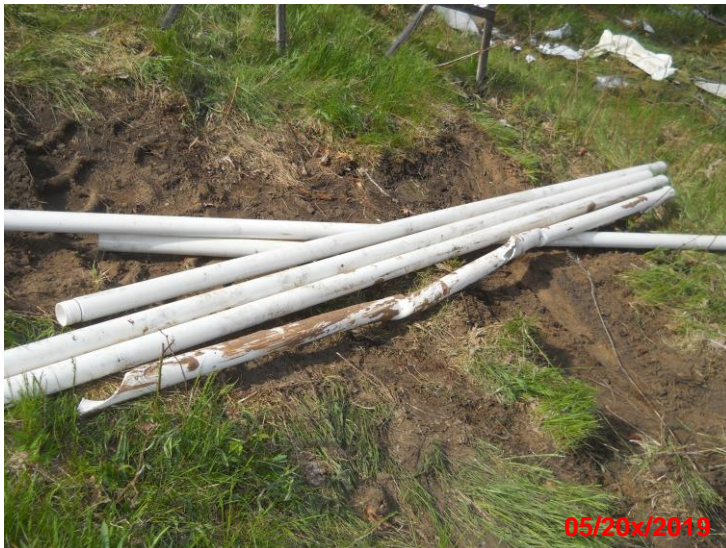
Casings removed from wells
