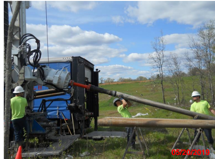
Traut Companies performing Rotary Sonic drilling
