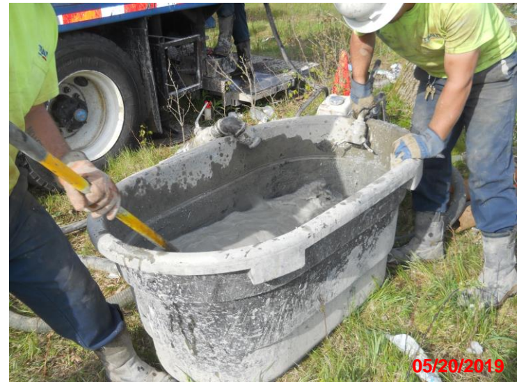
Mixing the bentonite-sand slurry to fill the boreholes
