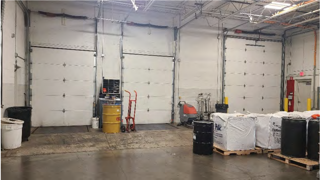
Photo #13 - Warehouse RM 124 - Loading Docks #2, #3 and #4 (Inside)
