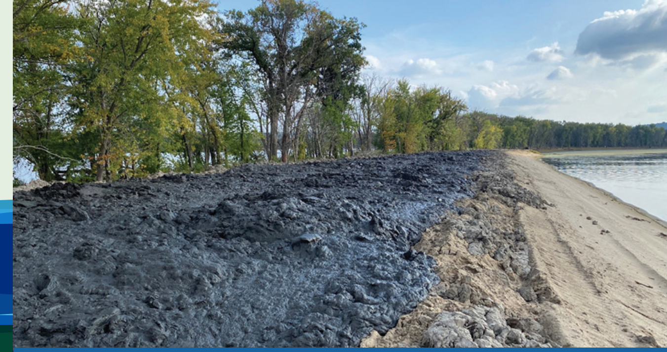
F14 – After Wet Topsoil Placed
