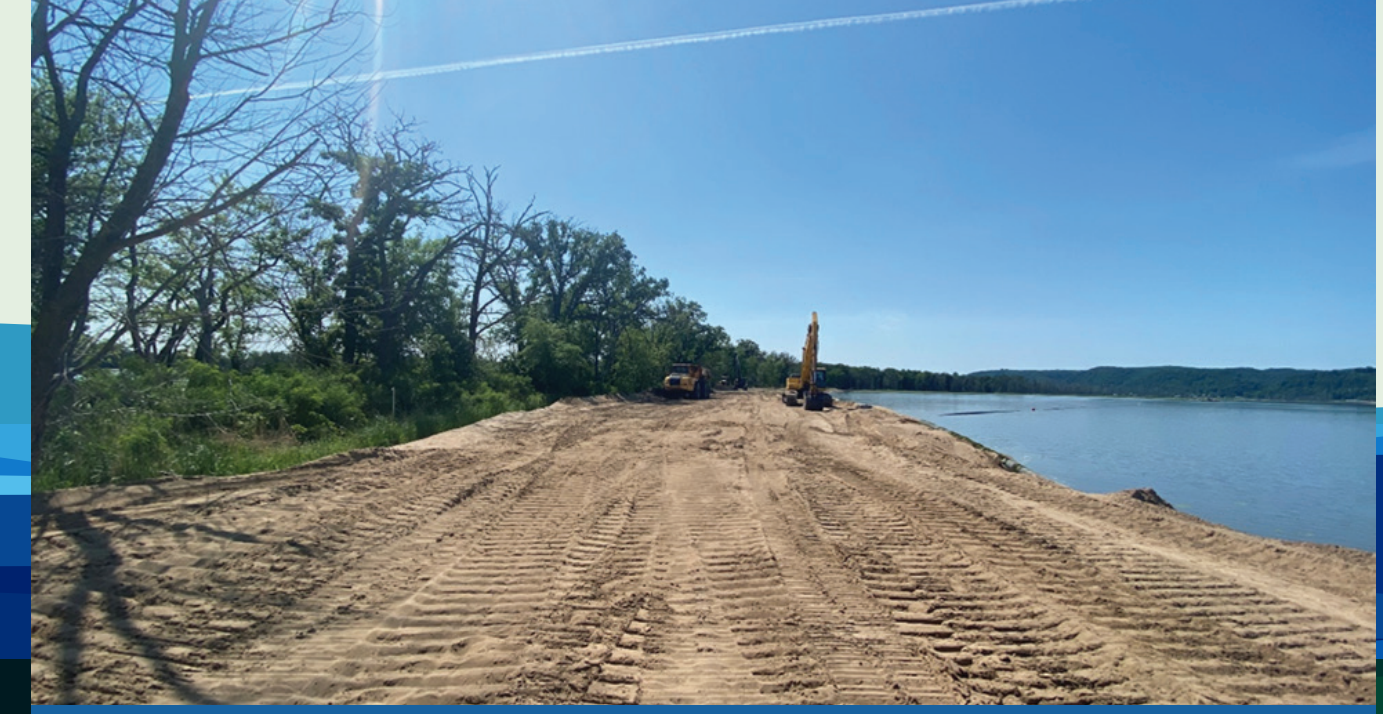
F14 – After Granular Fill Placed
