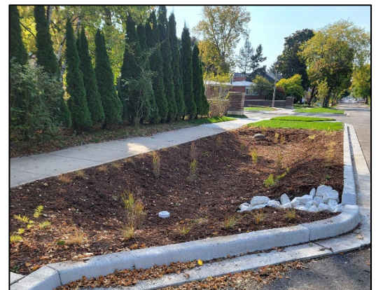
Bioswale along Downer Avenue. / Photo Credit: Village of Shorewood
