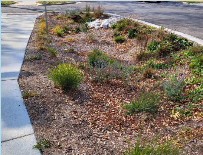
Bioswale along Menlo Boulevard. / Photo Credit: Village of Shorewood
