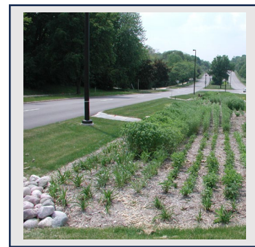
Photo credit: Wisconsin DNR. A biofilter built on the side of the road.
