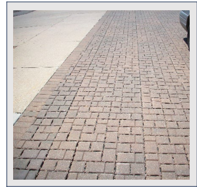
Photo credit: Wisconsin DNR. Permeable pavers in a parking lot.
