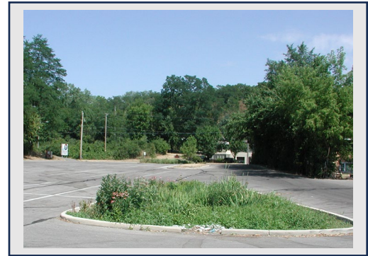
Photo credit: Wisconsin DNR. A biofilter in a parking lot.
