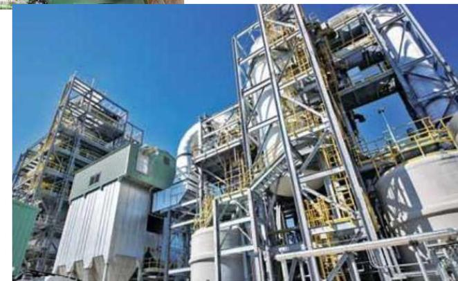
60,000 ton/year high-temp incineration for sorption media from liquid treatment (For about 130 MGD from WRRFs)
