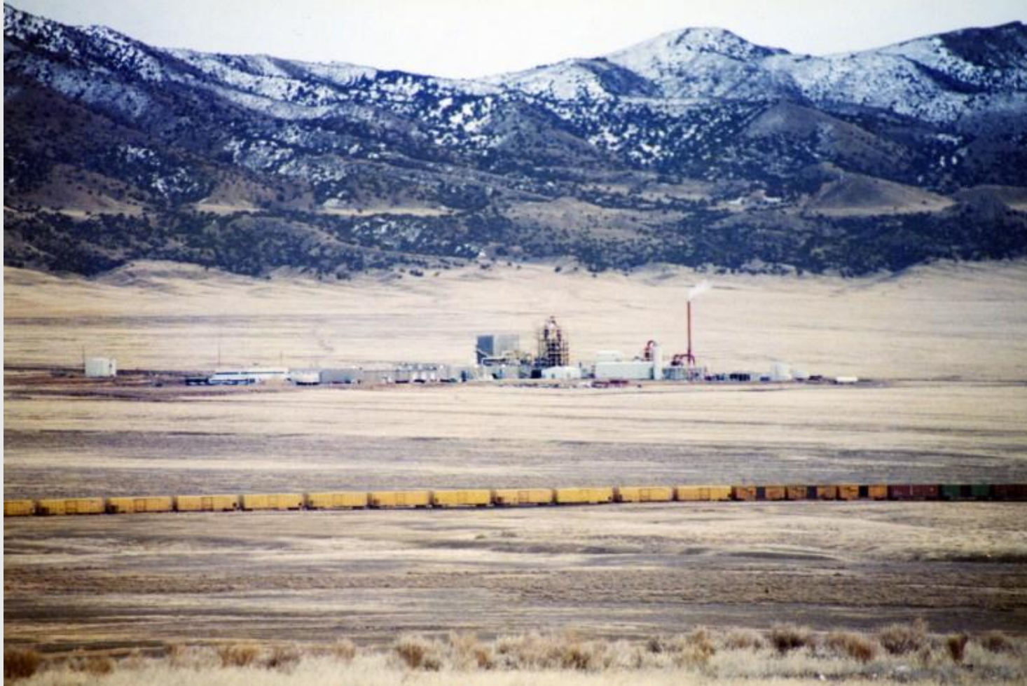
50,000 Ton per year Haz Waste Incinerator in Utah (Aragonite)
