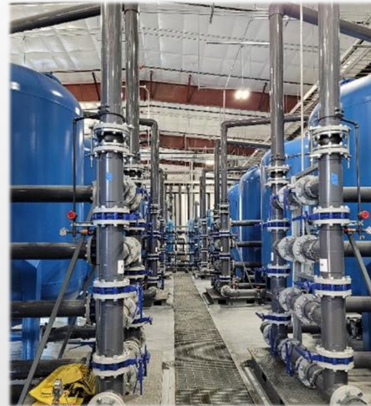
Inside GETS Building Carbon Filtration Vessels
