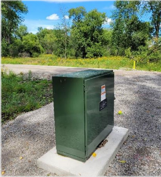
Extraction Well Control Box & Monitoring Well
