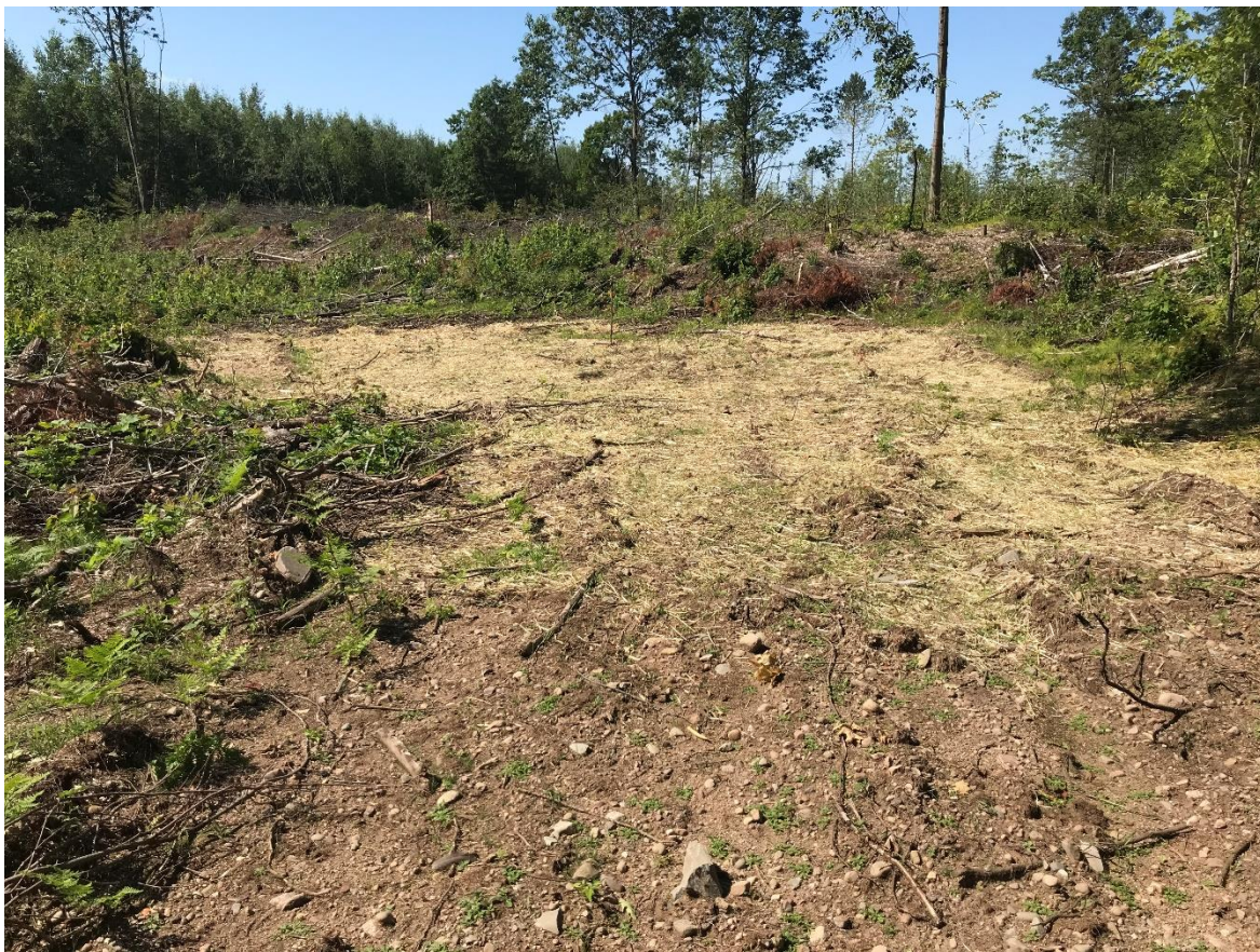
Drill pad for DB-03. Recently seeded & mulched, borehole at upper center, sump area on left. Viewing SW. JTH 8/6/20
